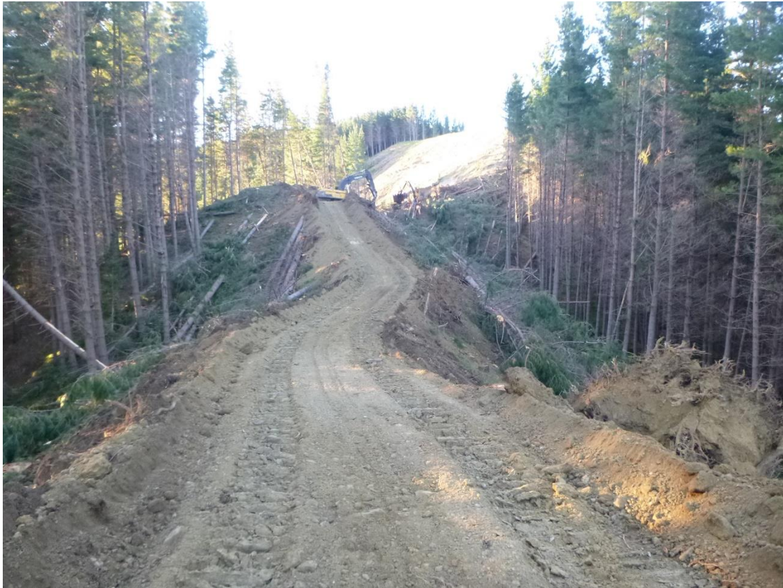
Photo 7: Tahurua Earthmovers tracking into Setting 509, Crozier Road to allow extraction by Log 19.
