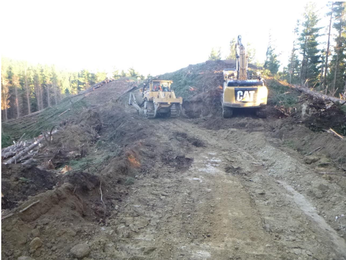
Photo 8: Tahurua Earthmovers tracking in Setting 509.
