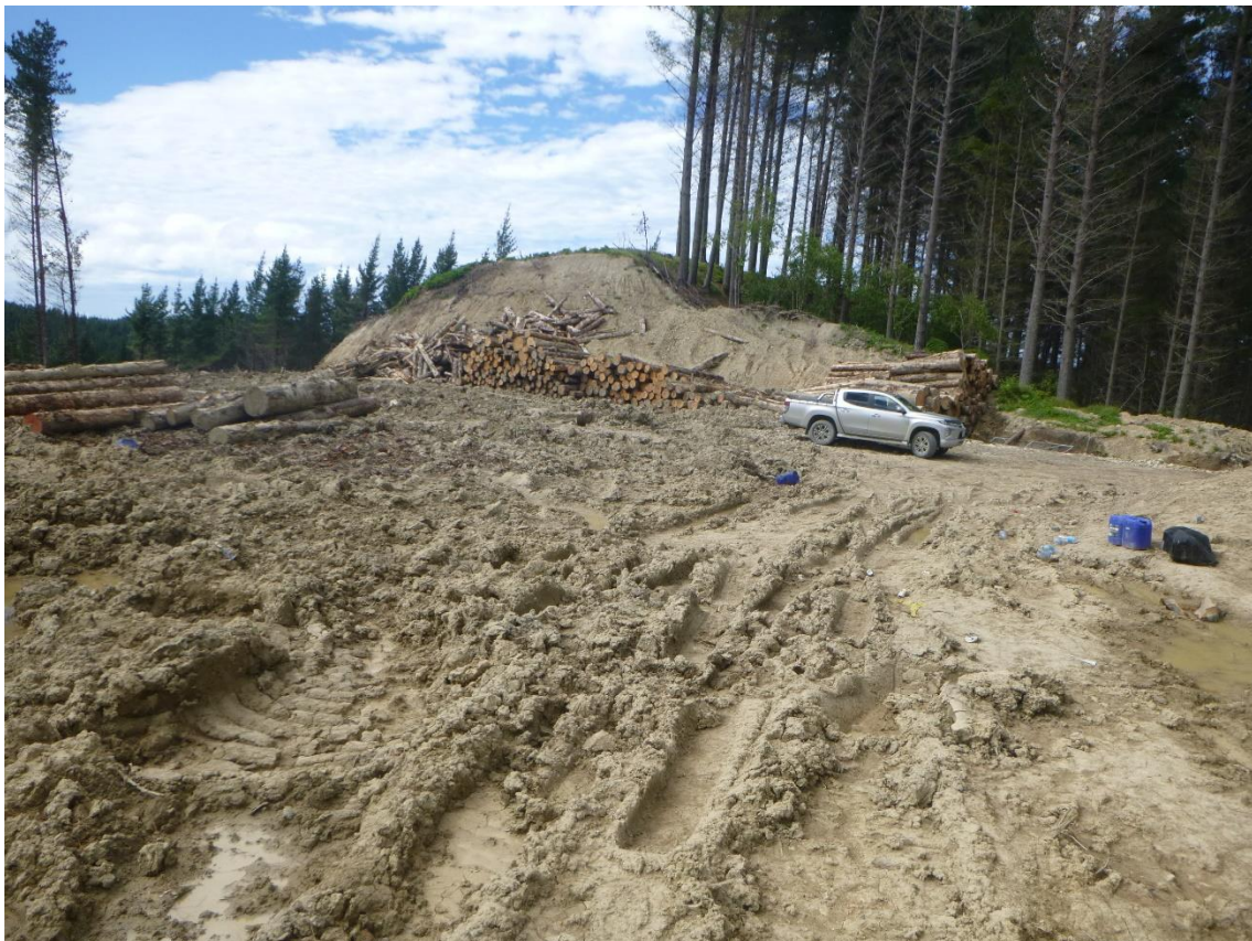
Photo 4: Log 15 completed working on Landing 31 extracting Setting 512.
