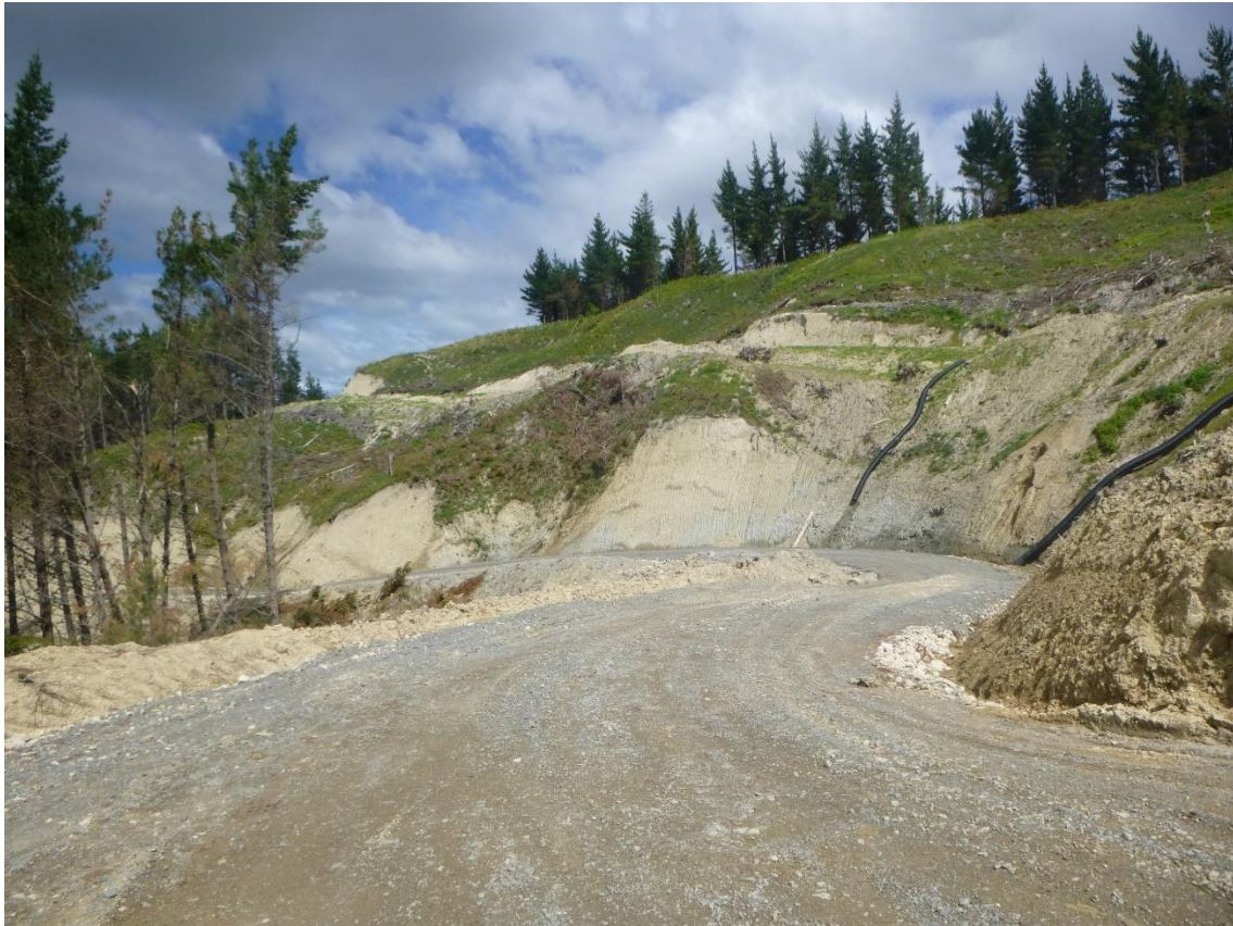
Photo 3: Repair work conducted by Galbraith Earth Movers and Forest Roading Maintenance on Hutchinson Road.
