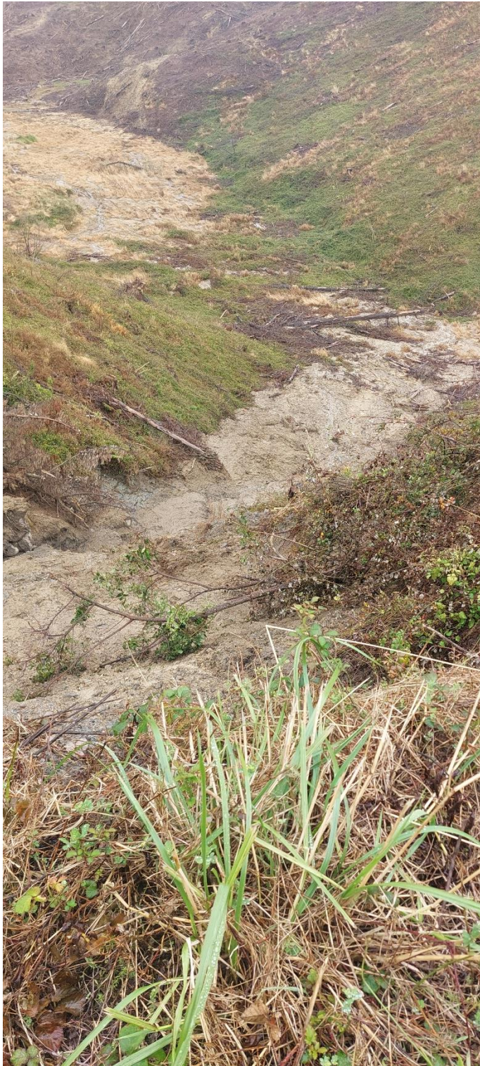
Photo 2: Dropout at Marker 14, Putere Road.
