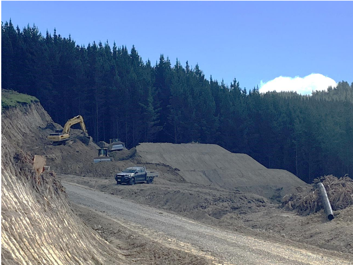
Photo 5: Tahurua Earthmovers working on Landing 34.
