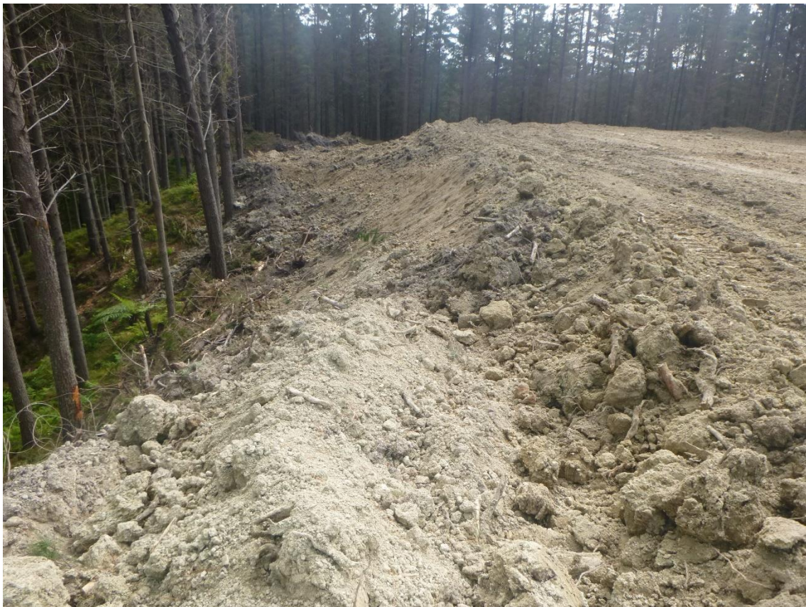
Photos 19 & 20: Galbraith Earth Movers forming Landing 48 on Kiwi Road.
