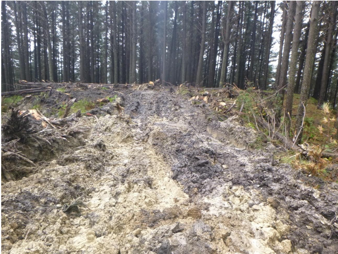
Photo 3: Log 15 clearing off proposed site for Landing 48.
