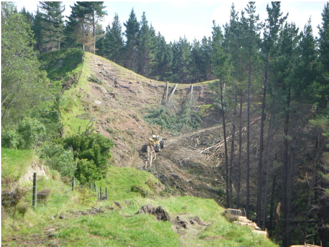
Photo 14: Log 15 extracting stems from Setting 510 back to Pad T2 for processing.
