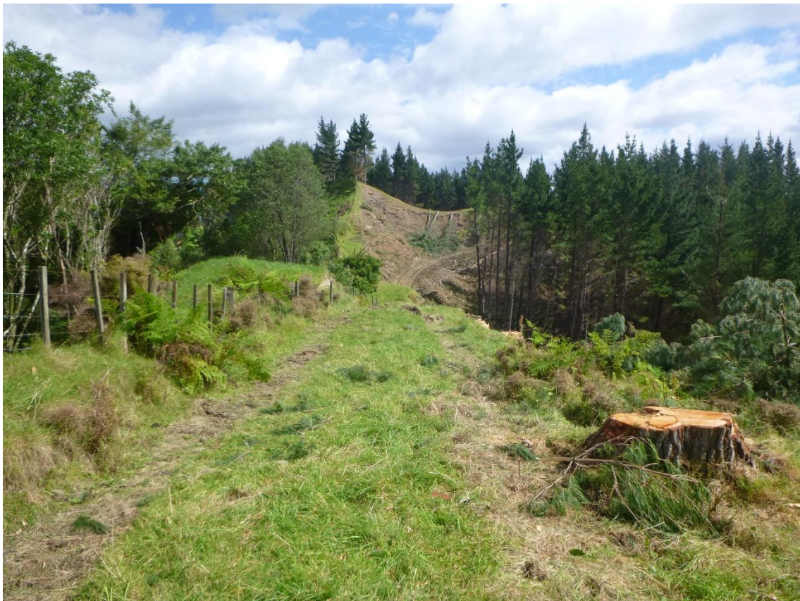
Photo 10: Log 15 falling and extracting stems in Setting 510 Dallas Road against significant native vegetation.
