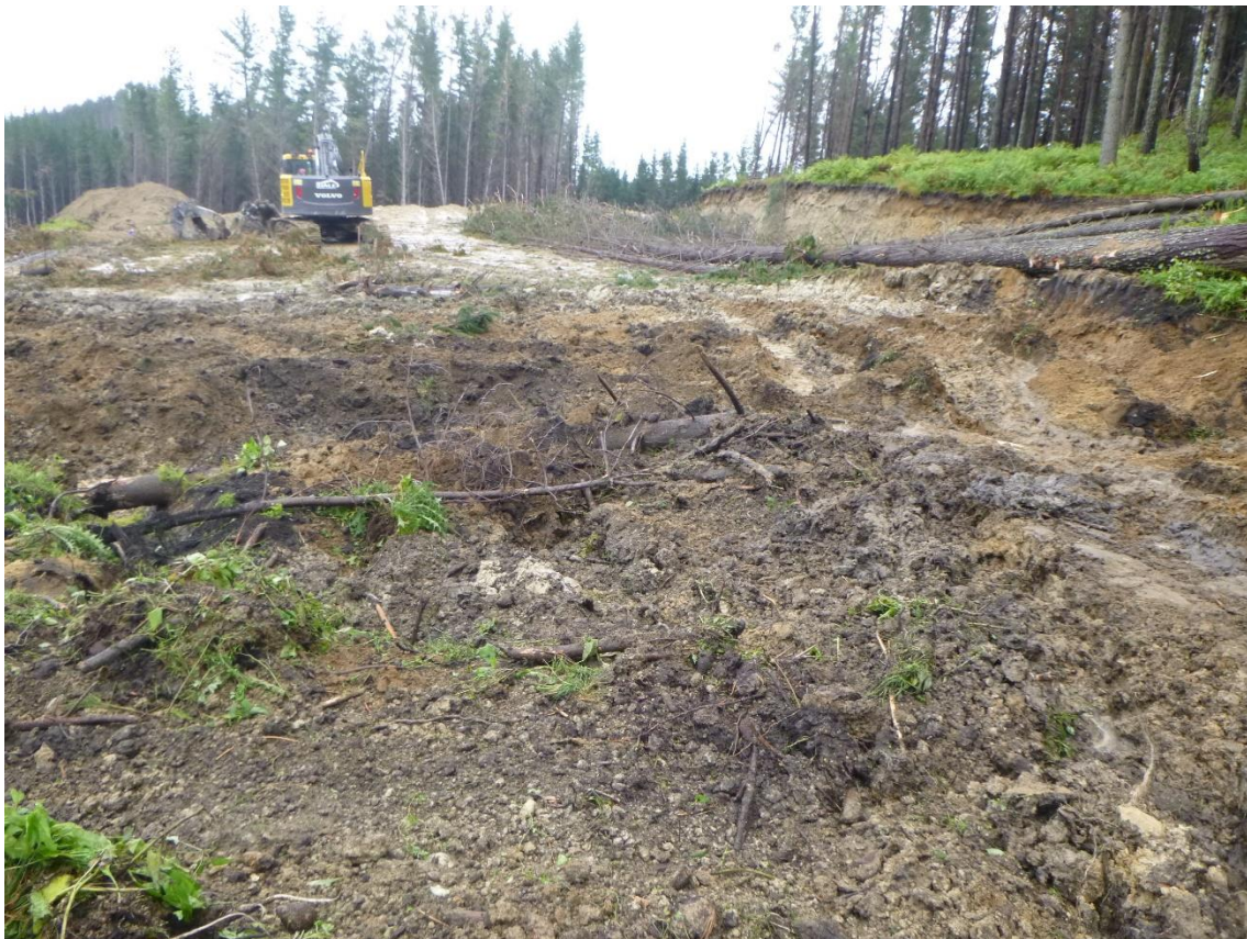
Photo 18: Galbraith Earth Movers formed Pad T2 on Kiwi Road – very soft after cyclone Gabrielle.
