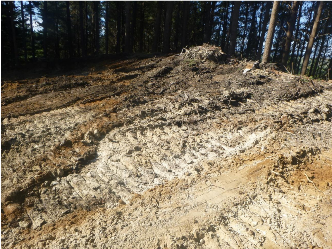
Photos 19 & 20: Galbraith Earth Movers forming Landing 48 on Kiwi Road.
