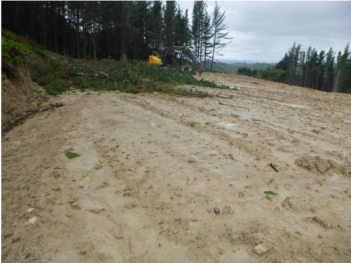
Photo 17: Galbraith Earth Movers formed Pad T2 on Kiwi Road.
