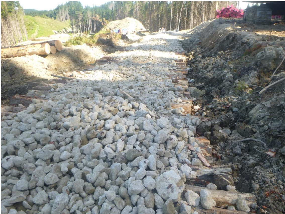
Photo 6: Metal scraped back and corduroy installed at Pad T2 in the loadout bay due to soft conditions.
