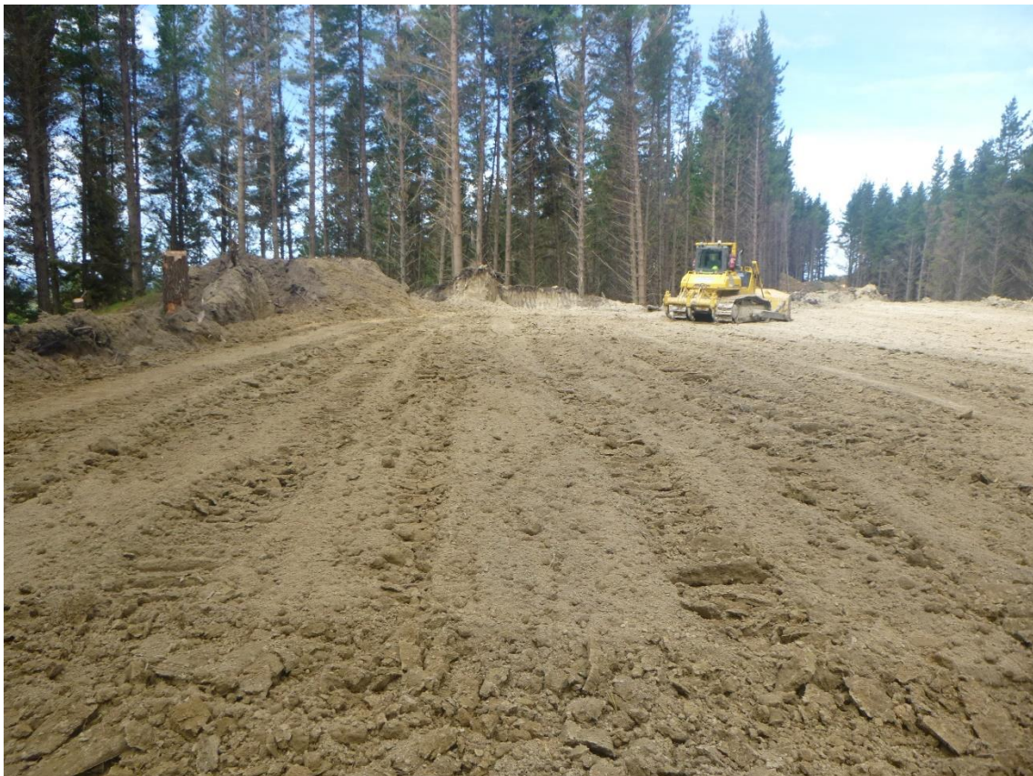
Photos 21 & 22: Galbraith Earth Movers forming landing 48 on Kiwi Road.
