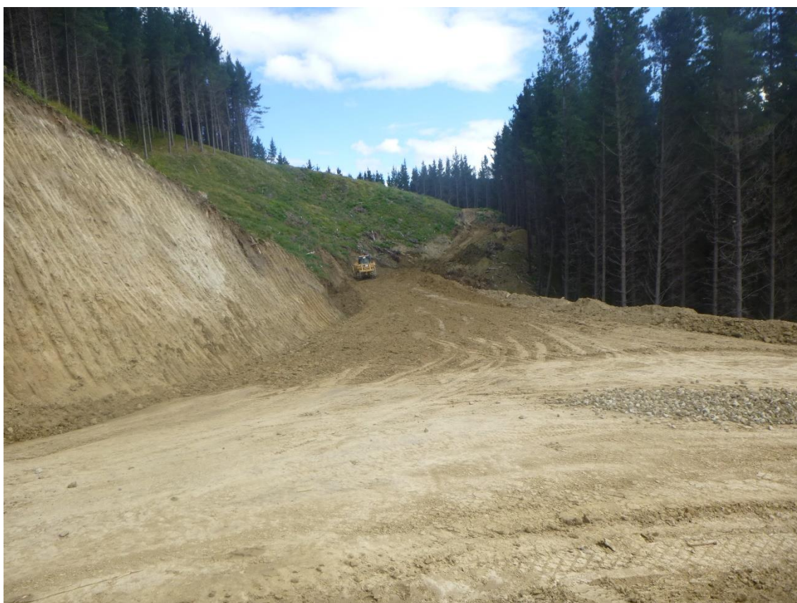
Photo 46: Tahurua Earthmovers forming intersection of Wood Road and Thomson Road near Landing 106.
