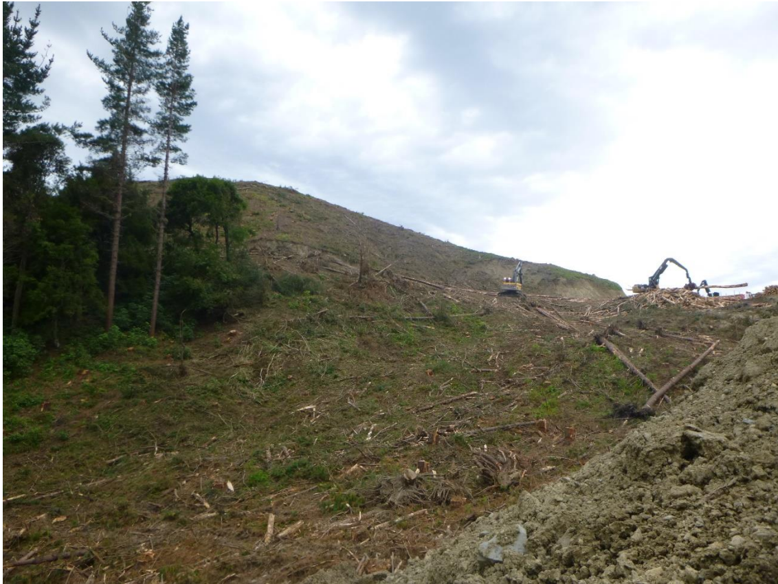
Photo 7: Log 19 shovelling stems off the face in Setting 504 for the construction of Shirley Road.
