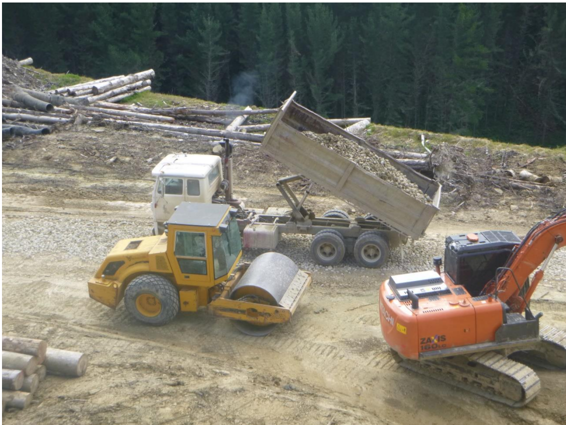
Photo 40: Tahurua Earthmovers metalling Wood Road.
