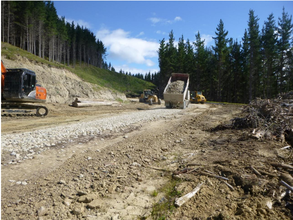
Photos 41 & 42: Tahurua Earthmovers metalling Wood Road.
