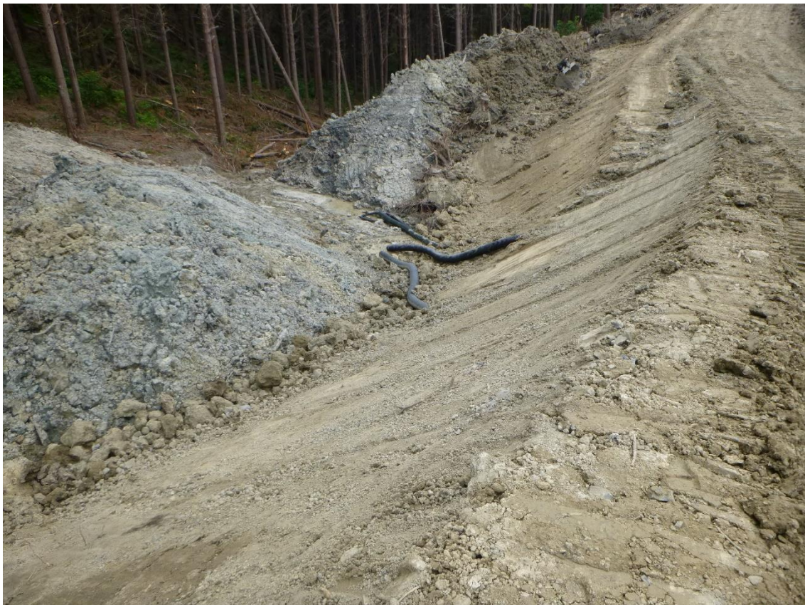
Photos 26: Water controls installed by Tahurua Earthmovers on Cooper Road.
