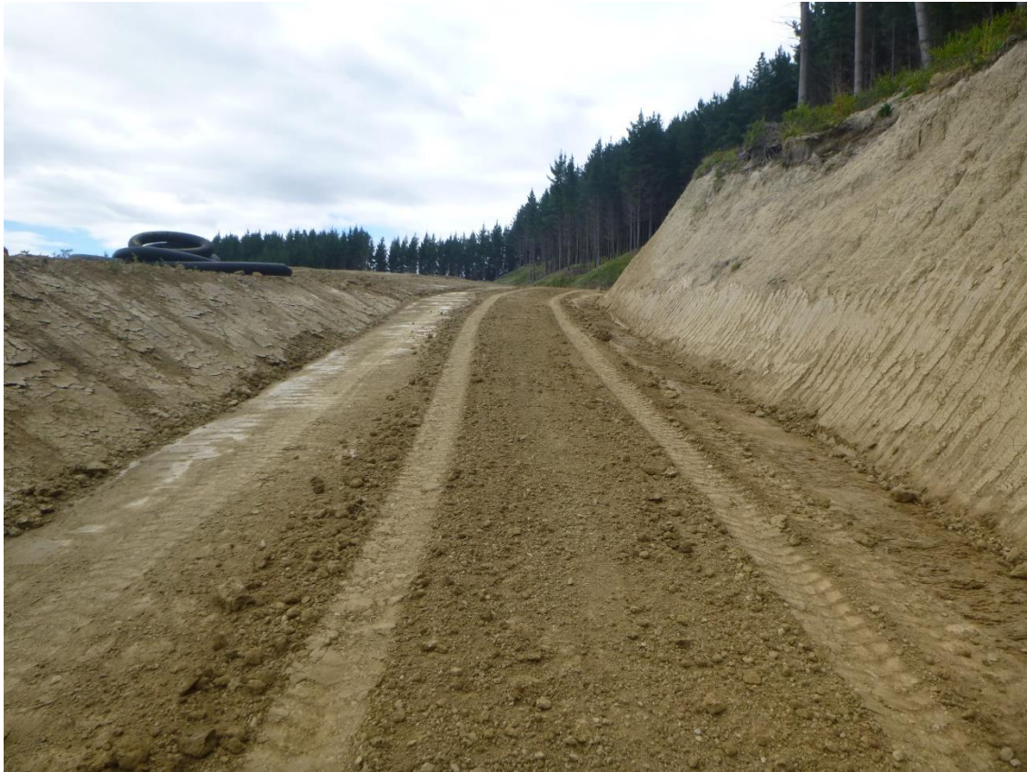
Photo 37: Tahurua Earthmovers forming Wood Road between Landings 106 and 43.
