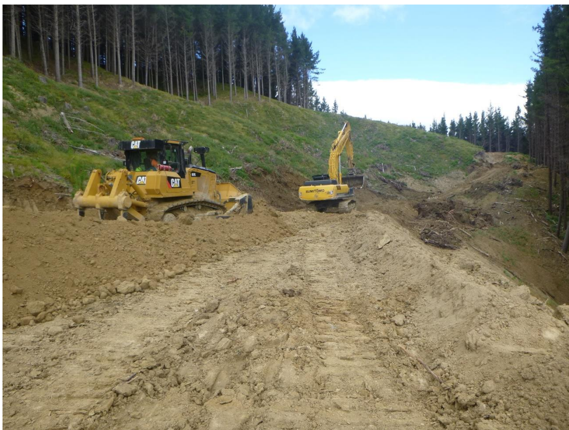
Photo 45: Tahurua Earthmovers undertaking post-harvest rehabilitation to Landing 10.
