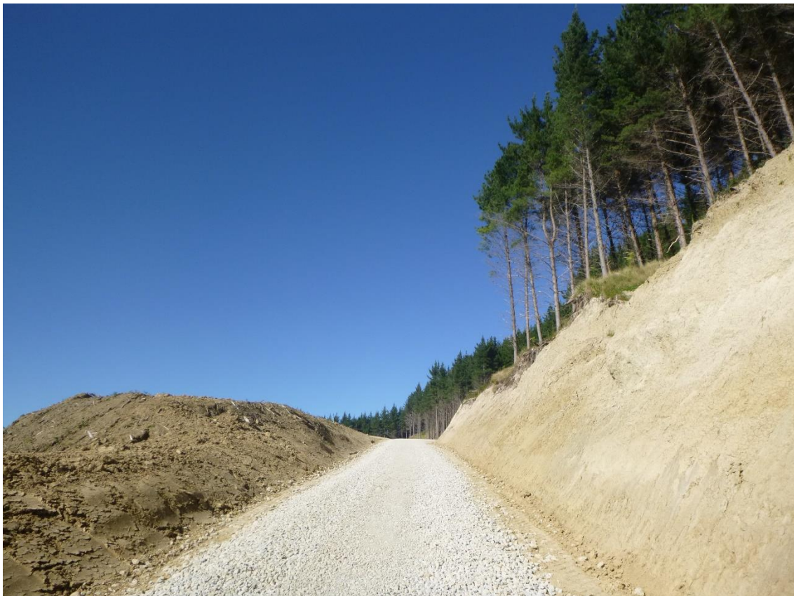
Photos 41 & 42: Tahurua Earthmovers metalling Wood Road.
