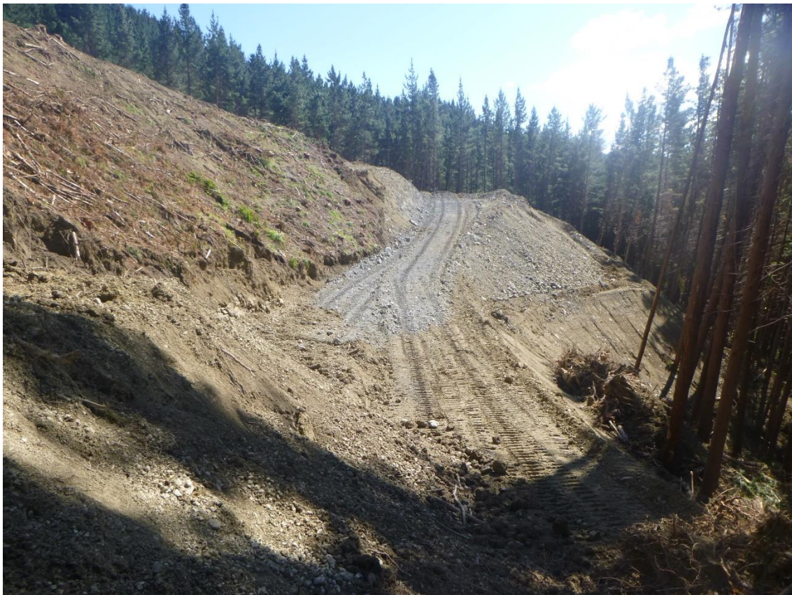
Photo 16: Tahurua Earthmovers constructing Landing 18 and the stab road leading to it.
