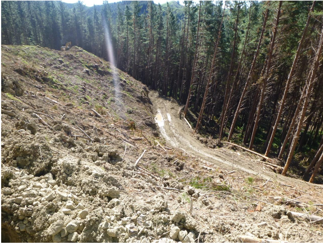
Photo 13: Tahurua Earthmovers constructing benching for Landing 18 on Mad Mutt Road.
