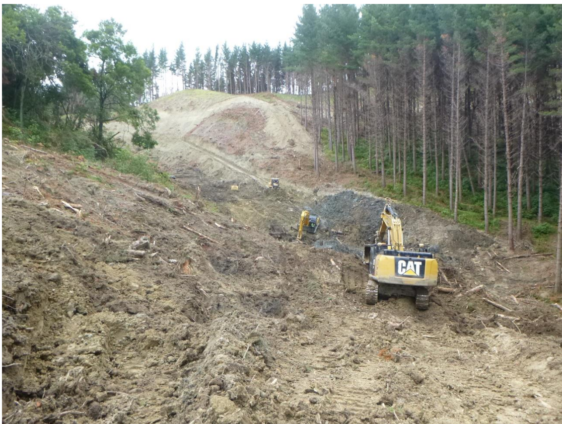
Photo 24: Tahurua Earthmovers installing drainage on Cooper Road.
