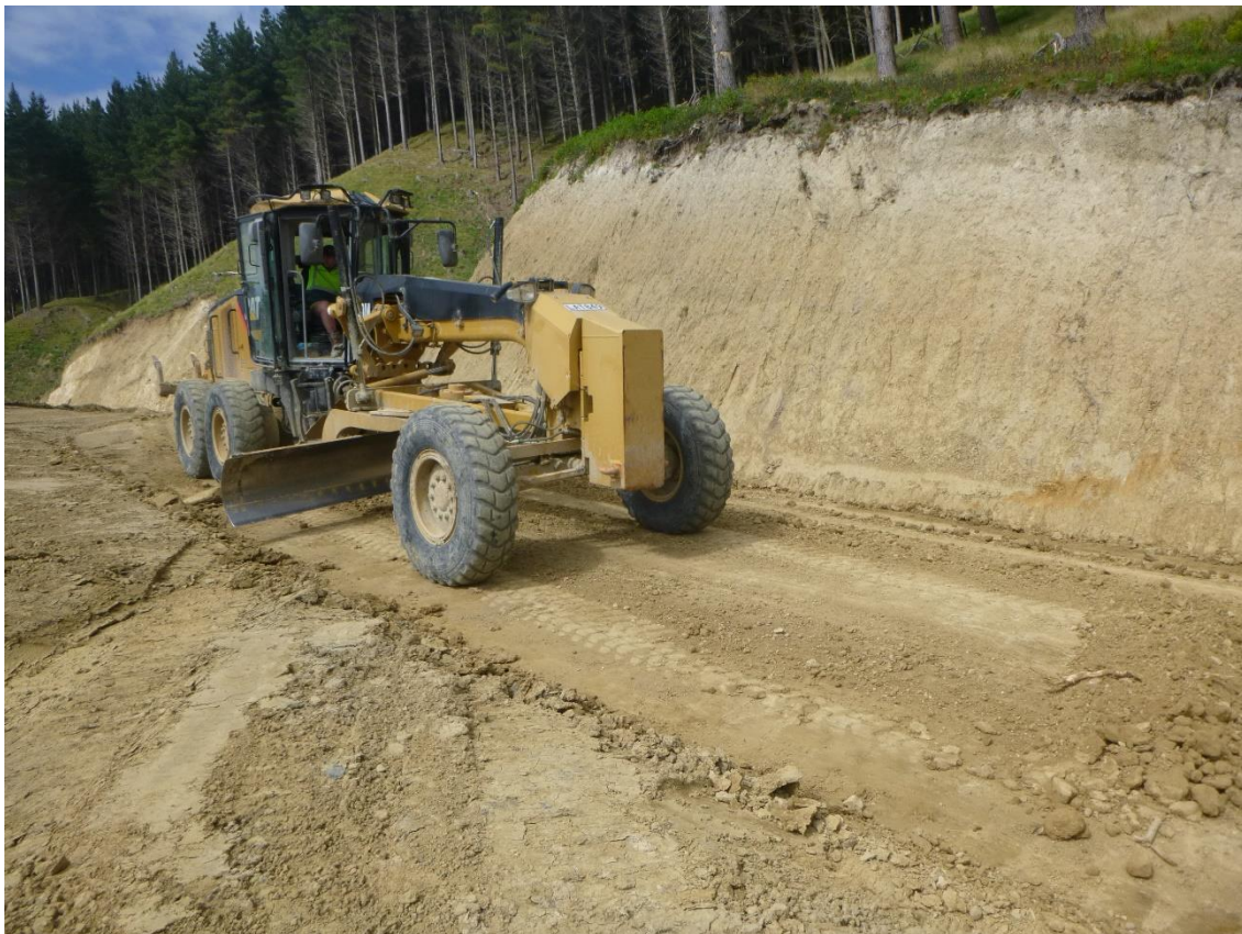
Photo 38: Tahurua Earthmovers grading / shaping Wood Road between Landings 106 and 43 in preparation for metalling.
