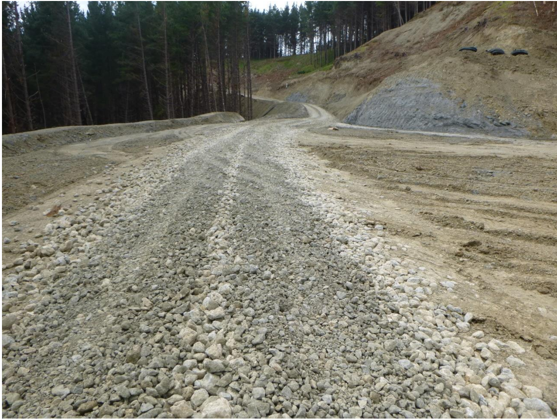
Photo 19: Tahurua Earthmovers metalling a loadout bay on Landing 18.
