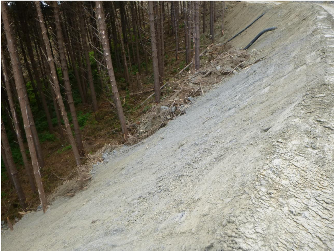
Photo 21: Tahurua Earthmovers forming Mad Mutt Road and installing water controls between Landings 10 and 18.
