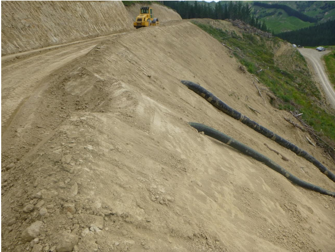
Photo 39: Tahurua Earthmovers forming Wood Road between Landings 106 and 43 and installed water controls.
