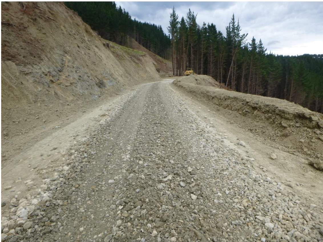
Photo 22: Tahurua Earthmovers metalling Mad Mutt Road between Landings 10 and 18.
