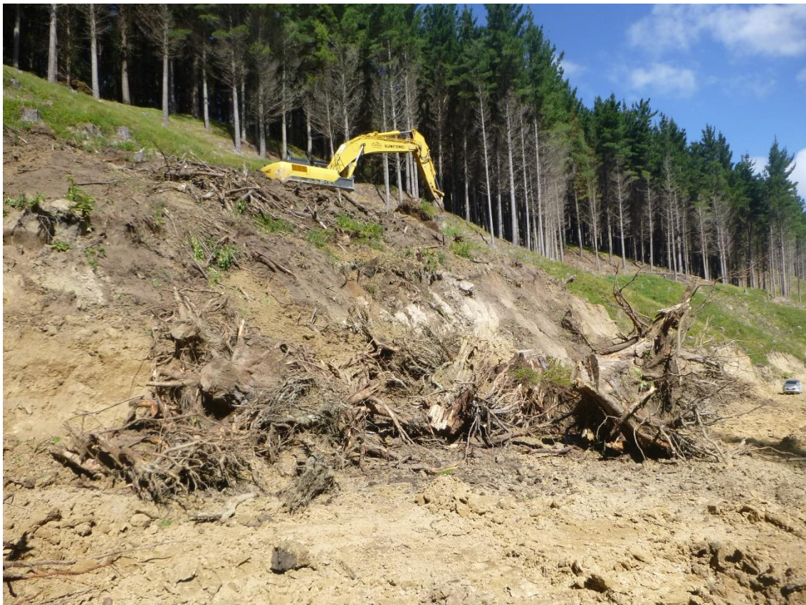
Photos 27 & 28: Tahurua Earthmovers constructing Landing 43 on Wood Road.
