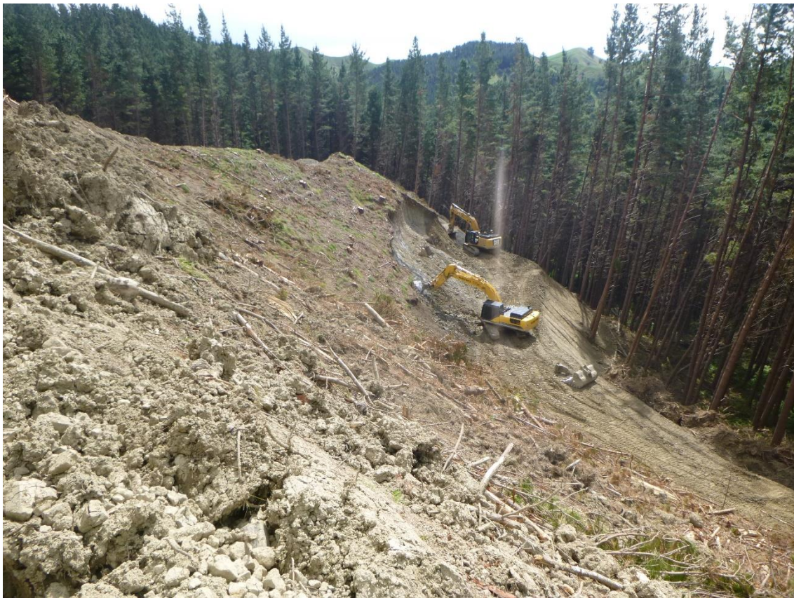
Photo 14: Tahurua Earthmovers constructing Landing 18.
