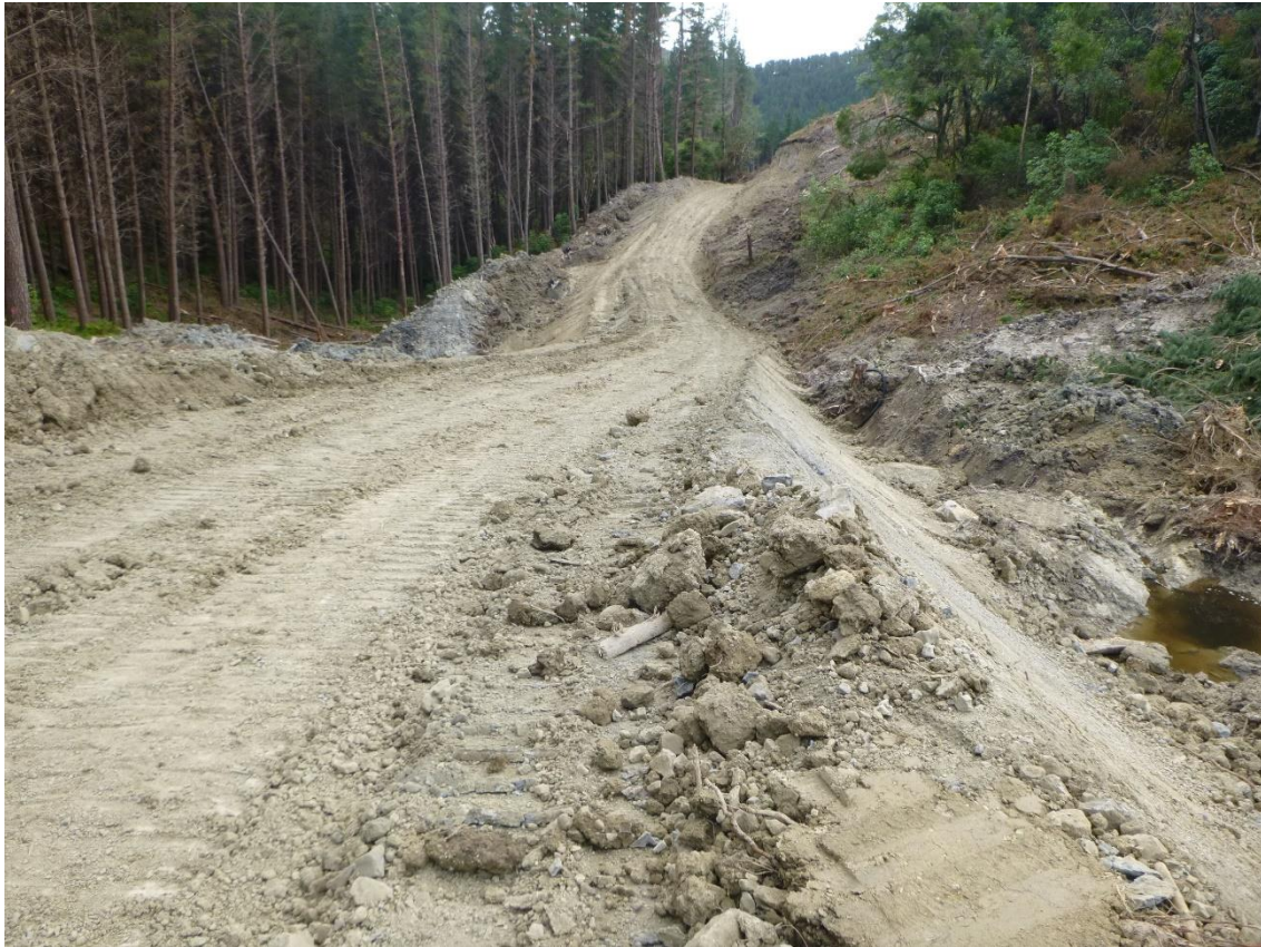
Photos 25: Tahurua Earthmovers forming Cooper Road between Landings 10 and 30.
