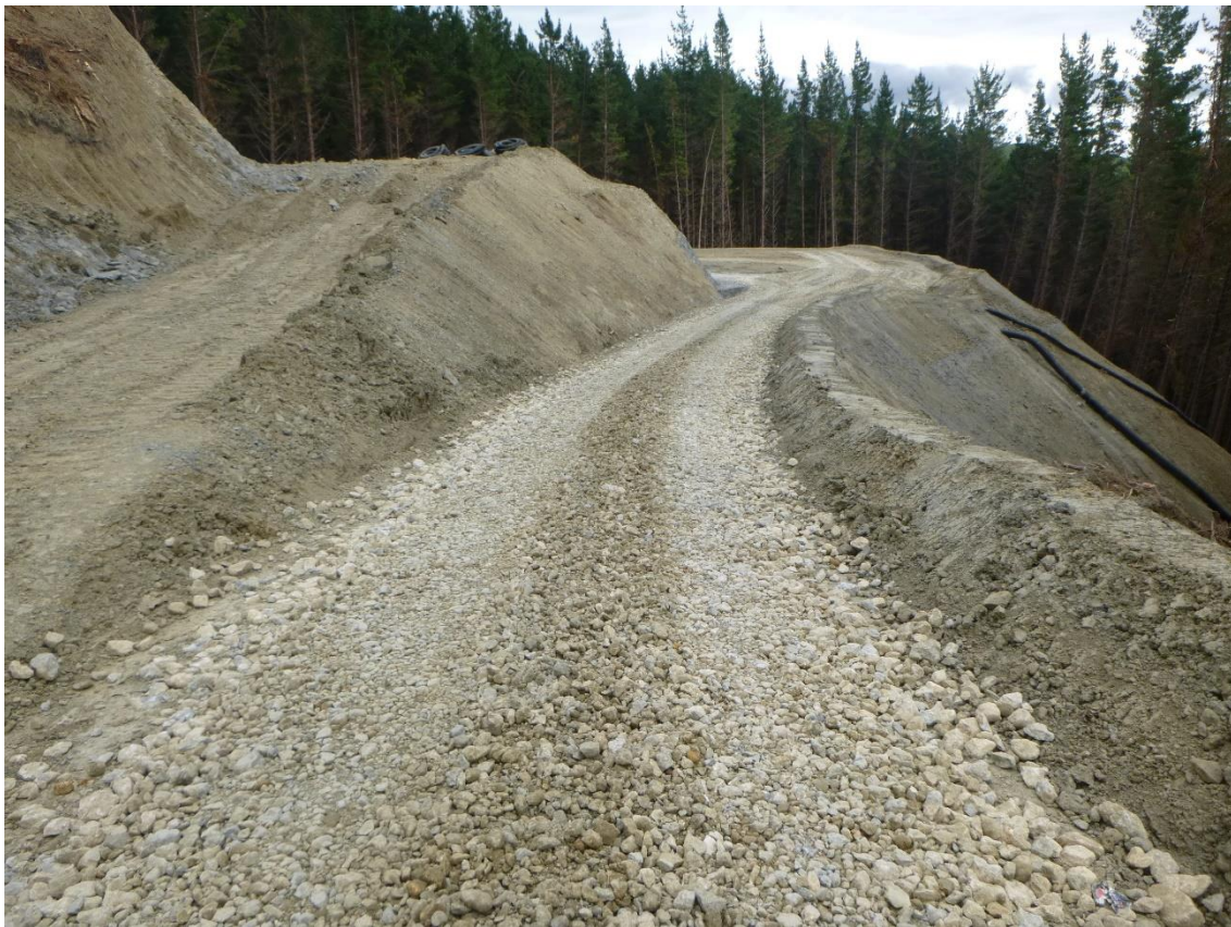
Photo 20: Tahurua Earthmovers metalling a stab road from Mad Mutt Road onto Landing 18.
