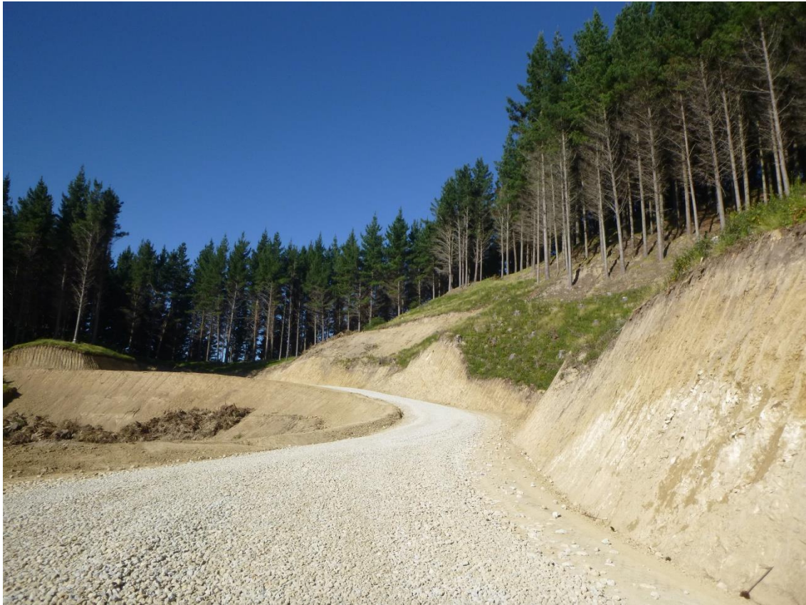
Photo 43: Tahurua Earthmovers metalled Wood Road between Landings 106 and 43.
