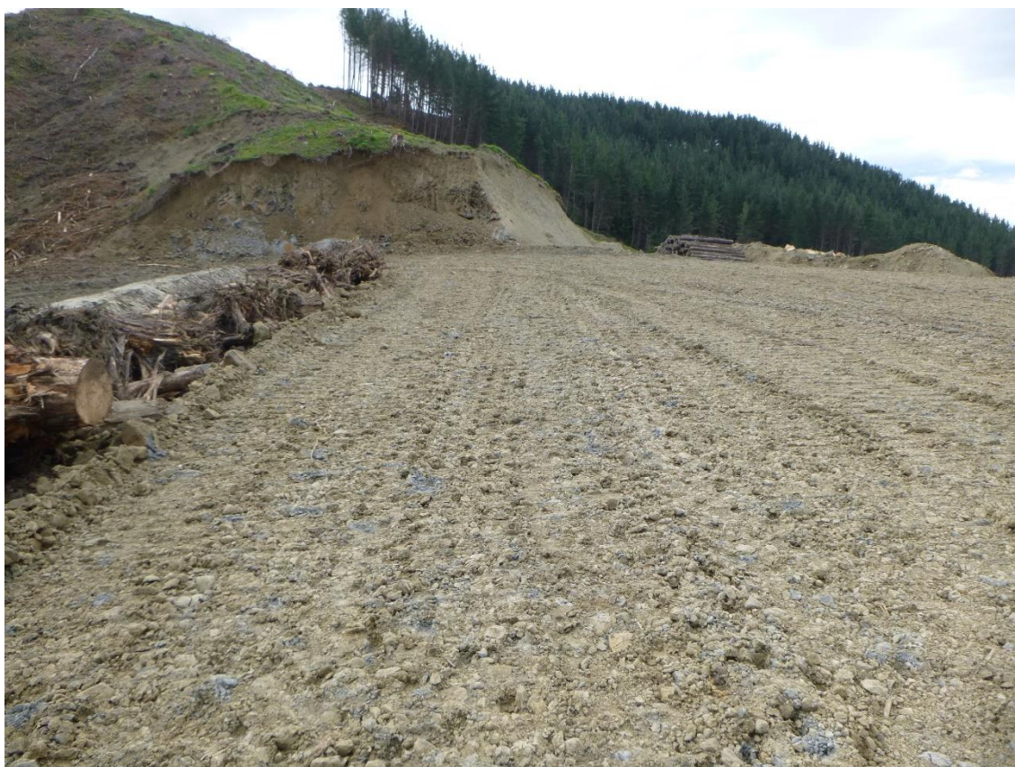
Photos 35 & 36: Tahurua Earthmovers undertaking post-harvest rehabilitation to Landing 10.
