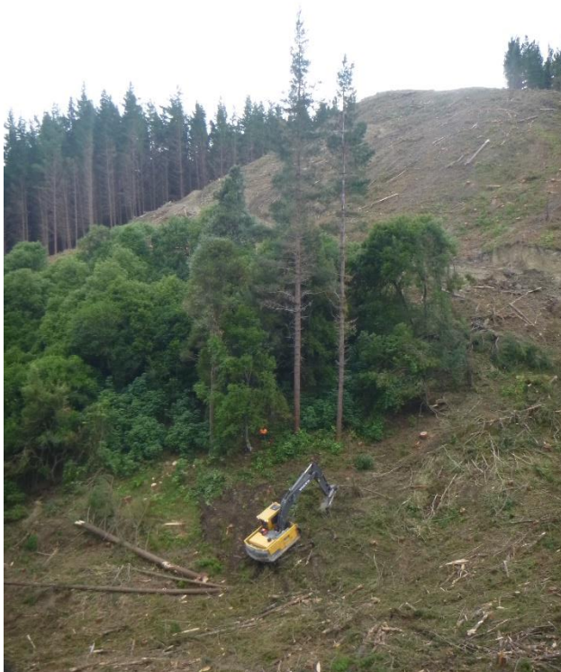
Photo 6: Log 19 machine assisting trees away from the native in Setting 504.
