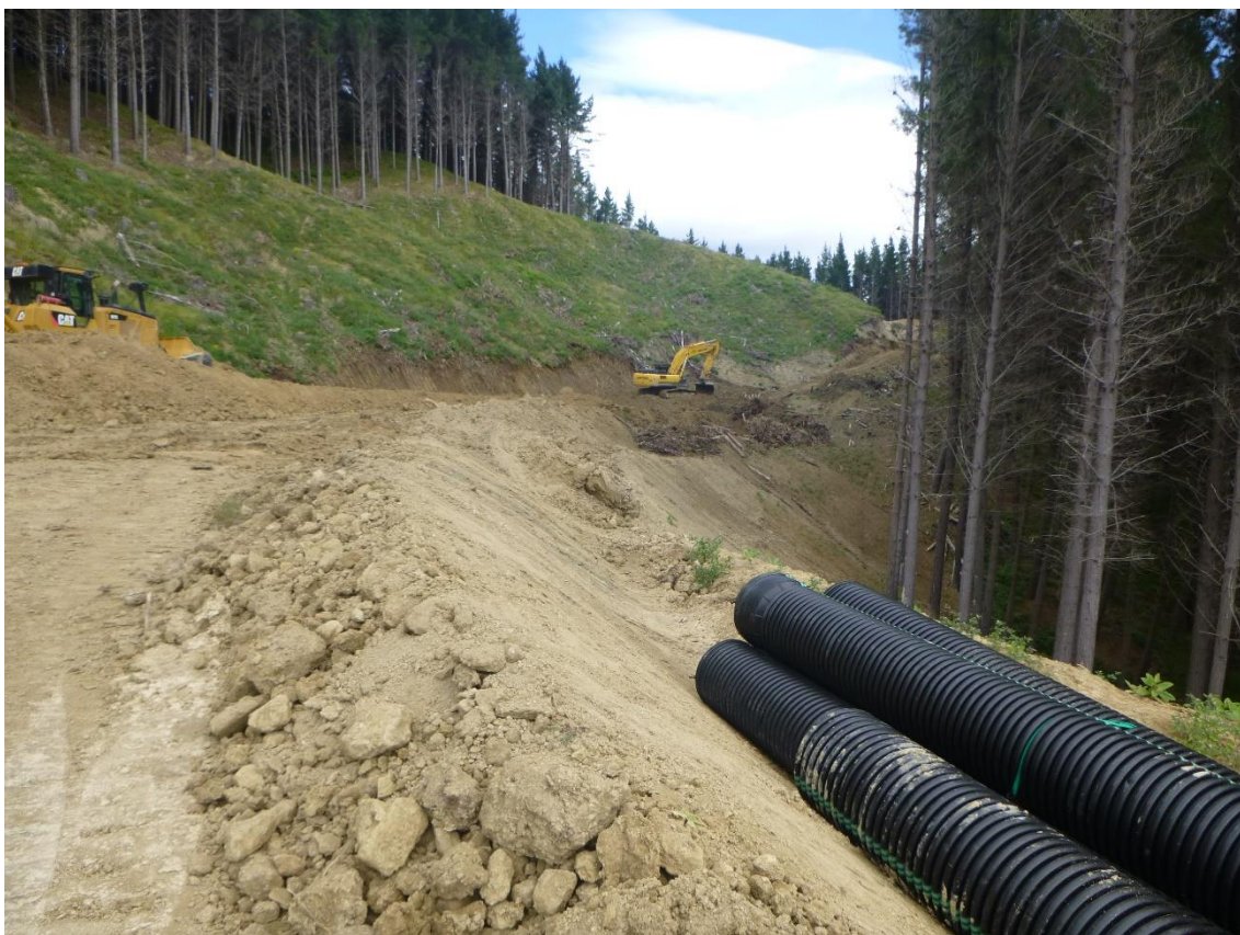
Photo 44: Tahurua Earthmovers undertaking post-harvest rehabilitation to Landing 10.
