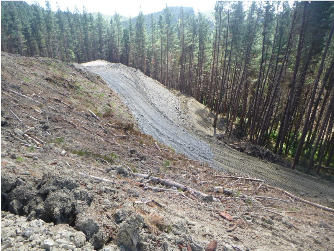
Photo 15: Tahurua Earthmovers constructing Landing 18.
