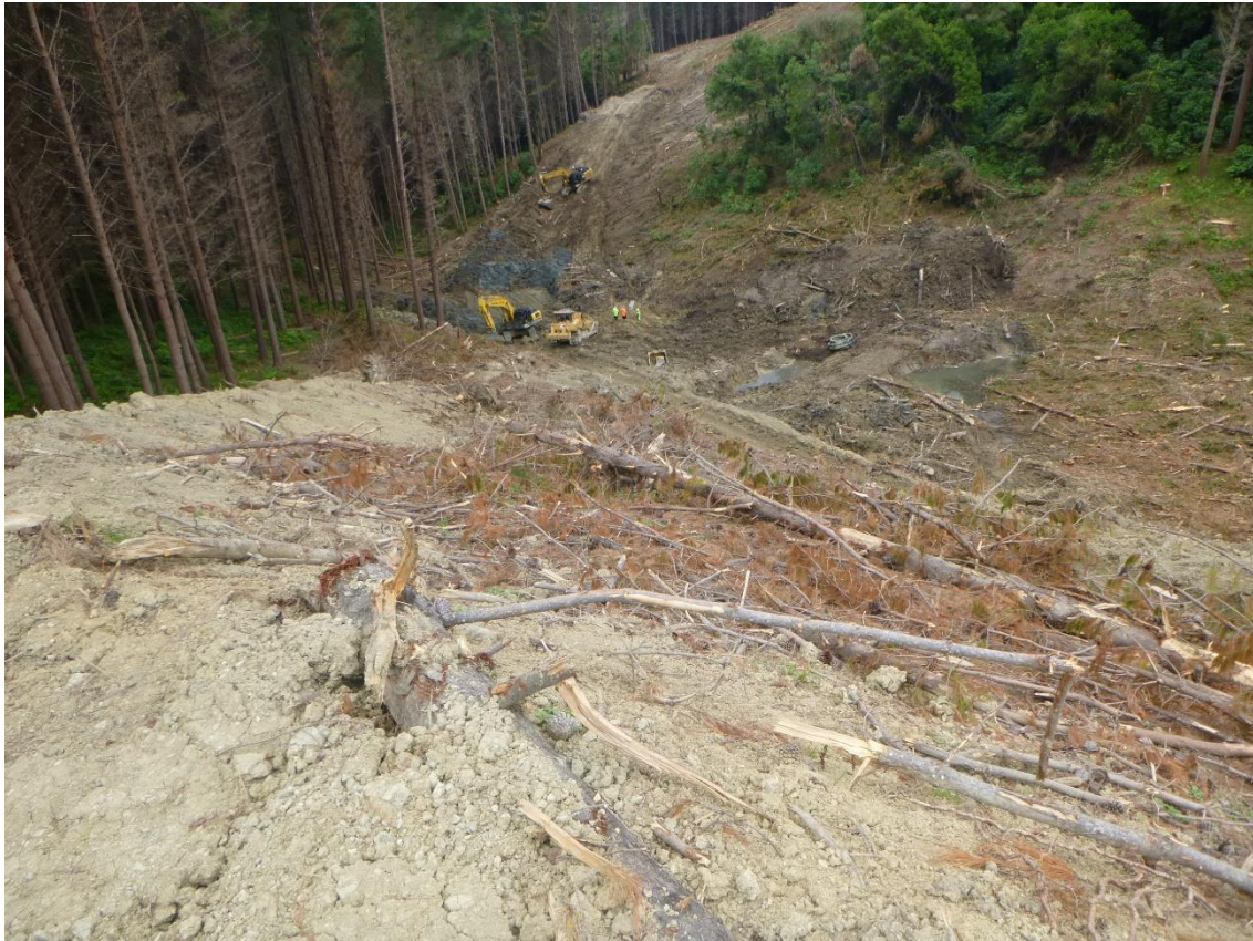
Photo 23: Tahurua Earthmovers beginning construction of Cooper Road and water controls between Landings 10 and 30.
