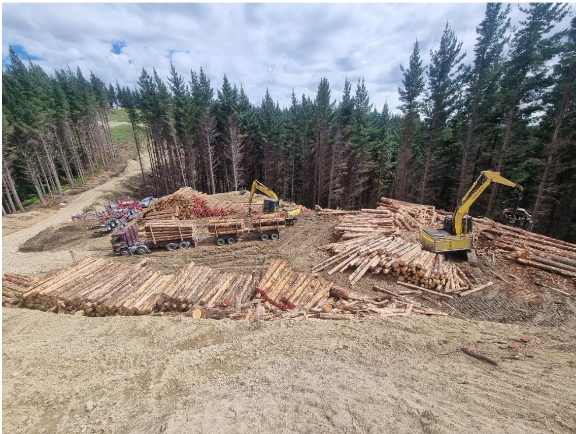
Photo 4: Operations on Landing 31 at the end of Hutchinson Road.
