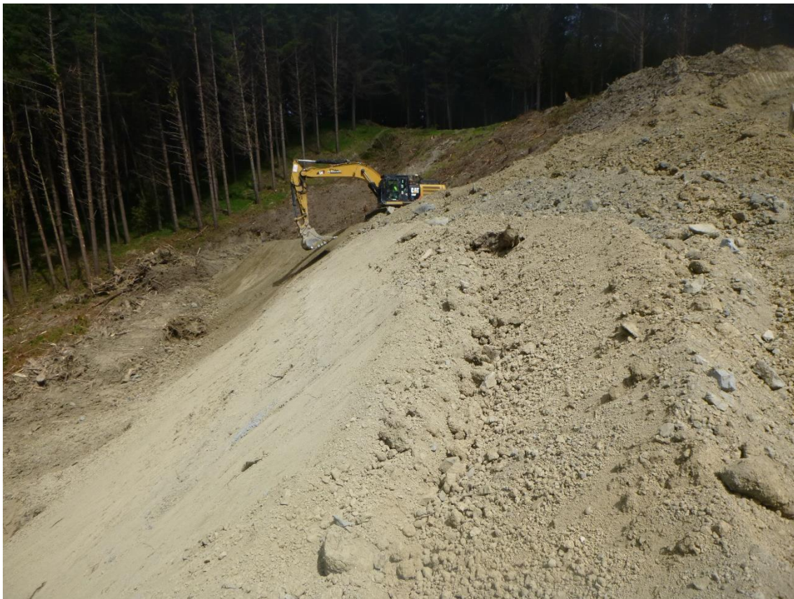
Photo 2: Tahurua Earthmovers benching and stabilising fill material on White Road.
