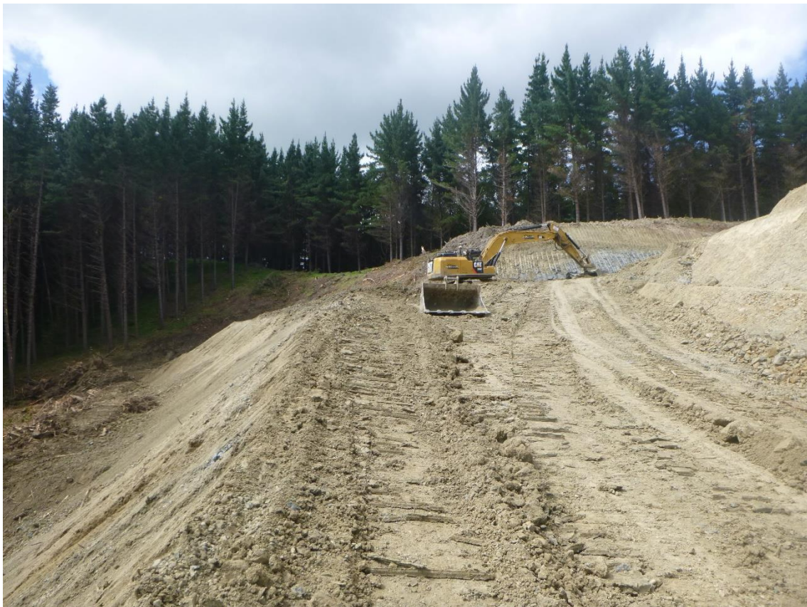
Photo 4: Tahurua Earthmovers forming the intersection of Mad Mutt and White Roads.
