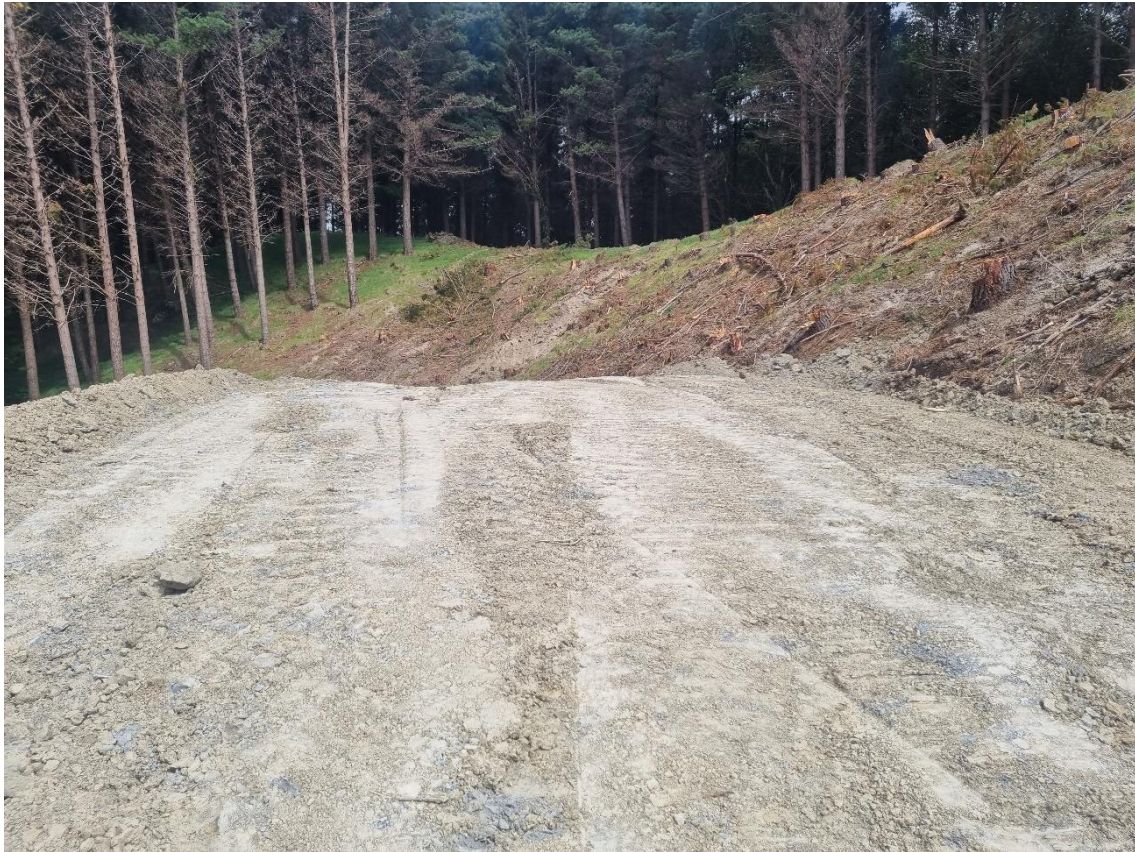
Photo 7: End of White Road looking at proposed location of Landing 11 to be constructed on the boundary of Heywood and Eastwood Forests.
