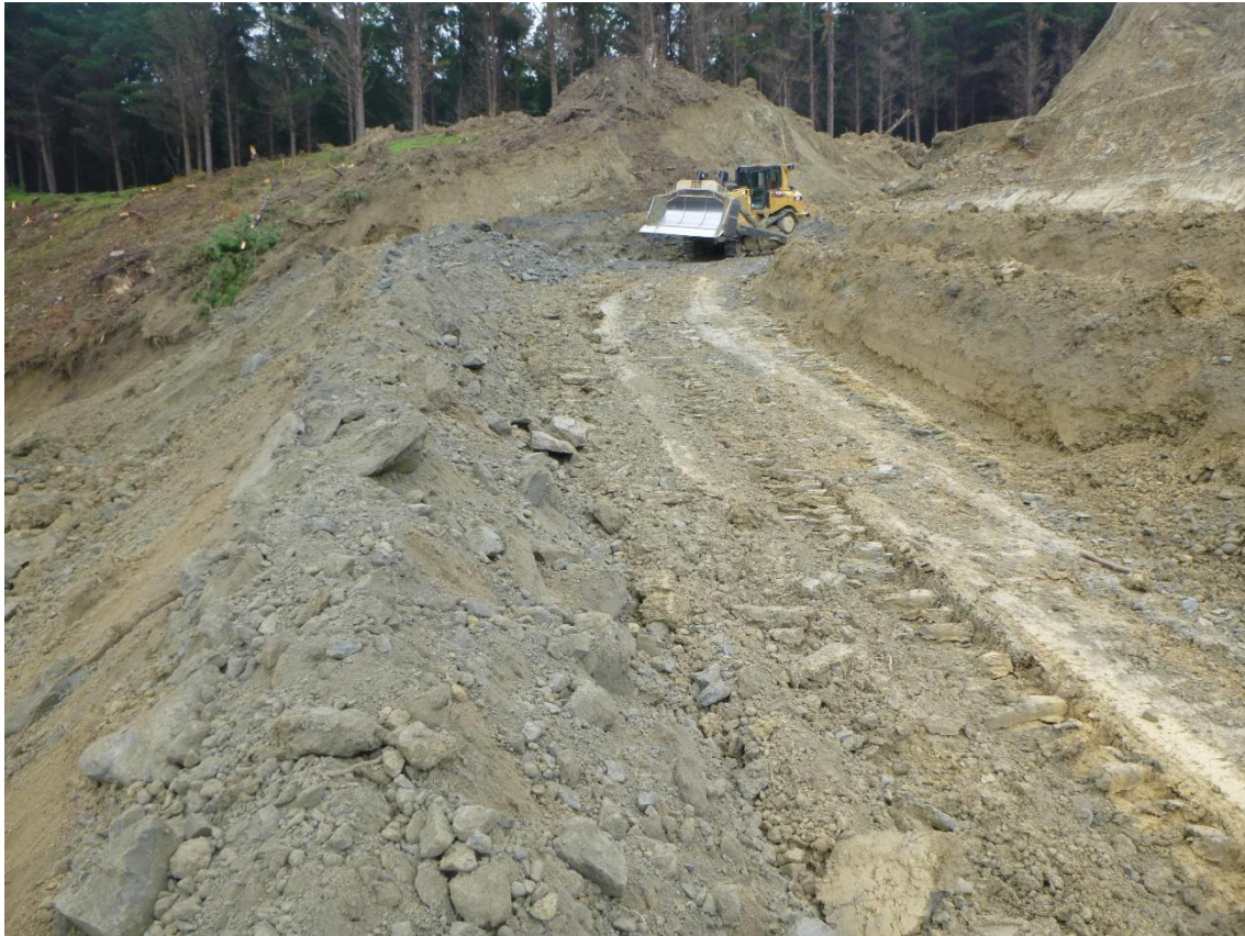
Photo 1: Tahurua Earthmovers forming intersection of White and Mad Mutt Roads. White Road will access Heywood Forest roadline Setting 505.
