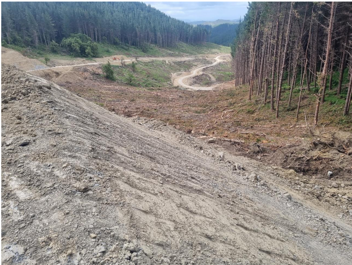
Photo 8: Fill material on the edge of White Road patted down and awaiting grass seeding.
