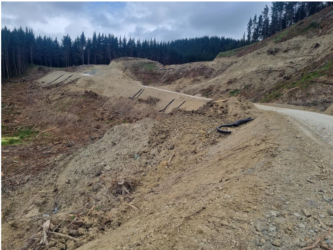
Photo 16: Taurua Earthmovers constructing Mad Mutt Road between Landings 9 and 10 following metalling.
