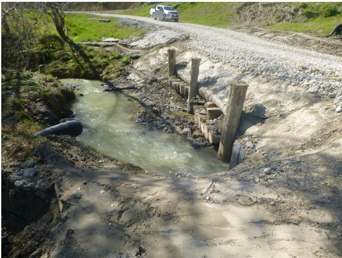
Photo 24: Completed repairs by Tahurua Earthmovers to the temporary crossing at the 3km marker on Mad Mutt Road following cyclone Gabrielle.
