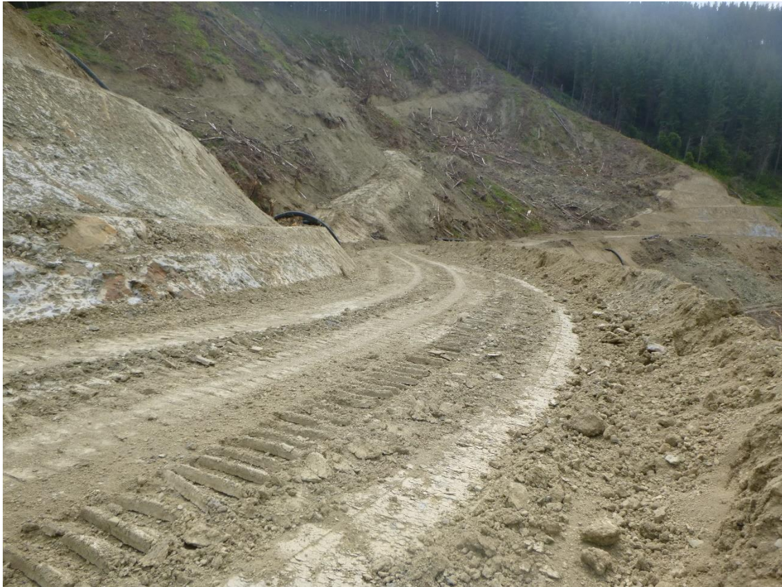
Photo 13: Tahurua Earthmovers constructing Mad Mutt Road between Landings 9 and 10.
