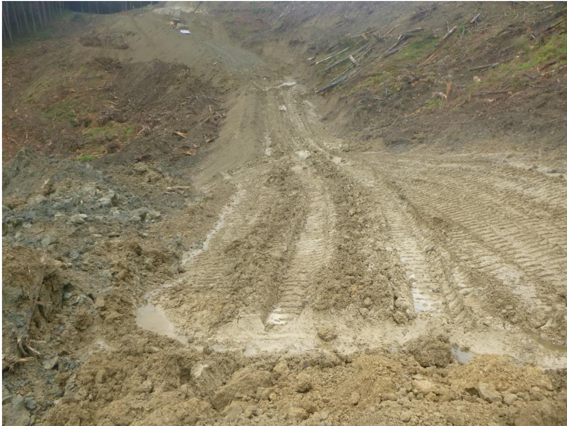
Photo 9: Tahurua Earthmovers constructing Mad Mutt Road between Landings 9 and 10.
