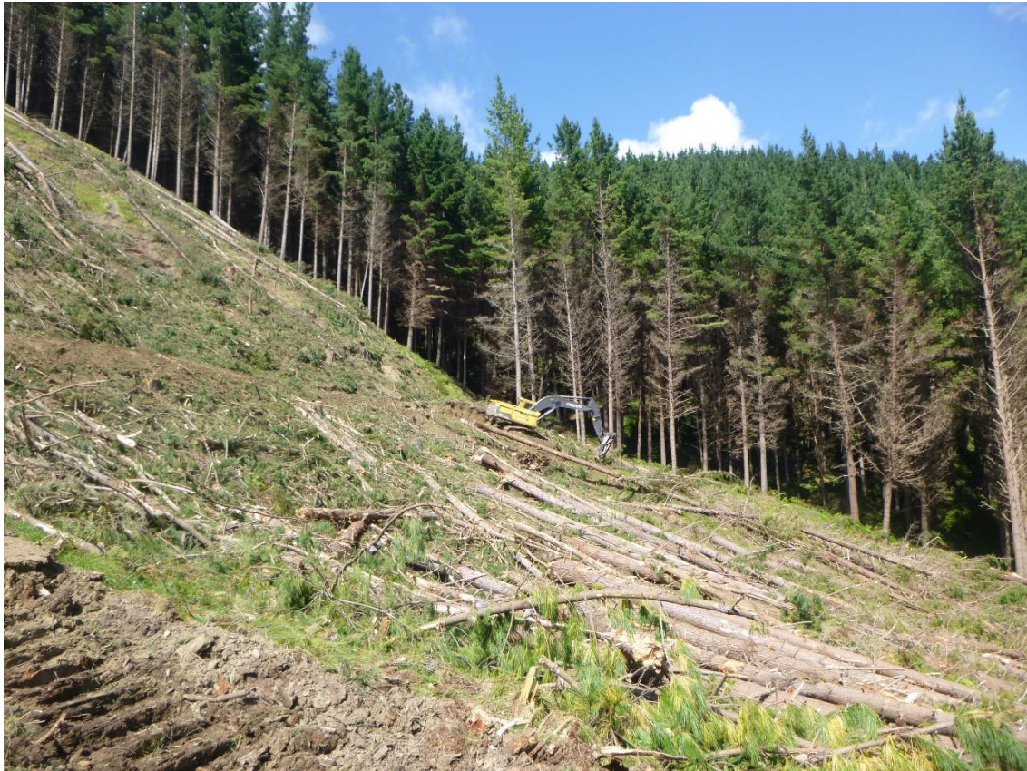
Photo 7: Log 19 shovelling stems off the face for the construction of Landing 18.
