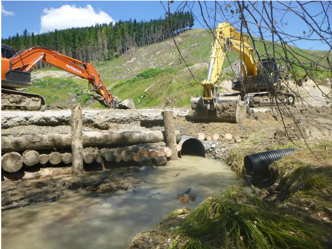
Photo 23: Tahurua Earthmovers undertaking repairs to the temporary crossing at the 3km marker on Mad Mutt Road following cyclone Gabrielle.
