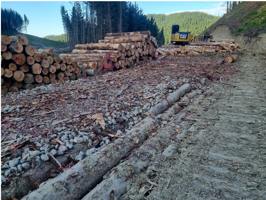
Photo 2: Log 19 operating on a very soft Landing 9A that required plenty of corduroy.
