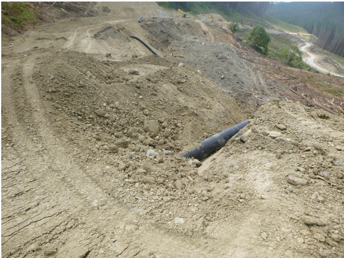
Photo 14: Tahurua Earthmovers constructing Mad Mutt Road between Landings 9 and 10, installing crossroad culverts and fluming.
