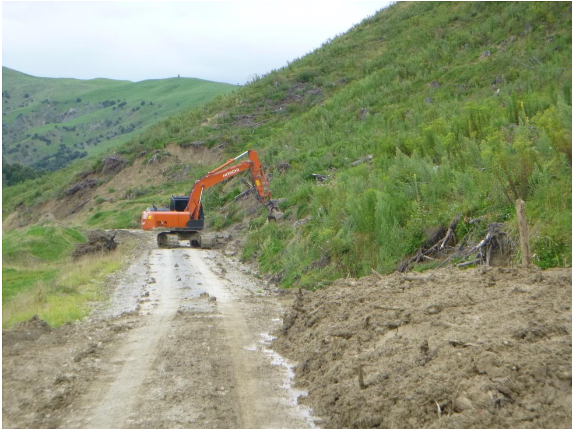
Photo 17: Tahurua Earthmovers carrying out maintenance to Mad Mutt Road following cyclone Gabrielle.
