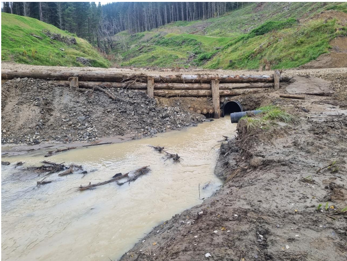
Photos 27 & 28: Completed repairs by Tahurua Earthmovers to the temporary crossing at the 3km marker on Mad Mutt Road following the second rain event.
