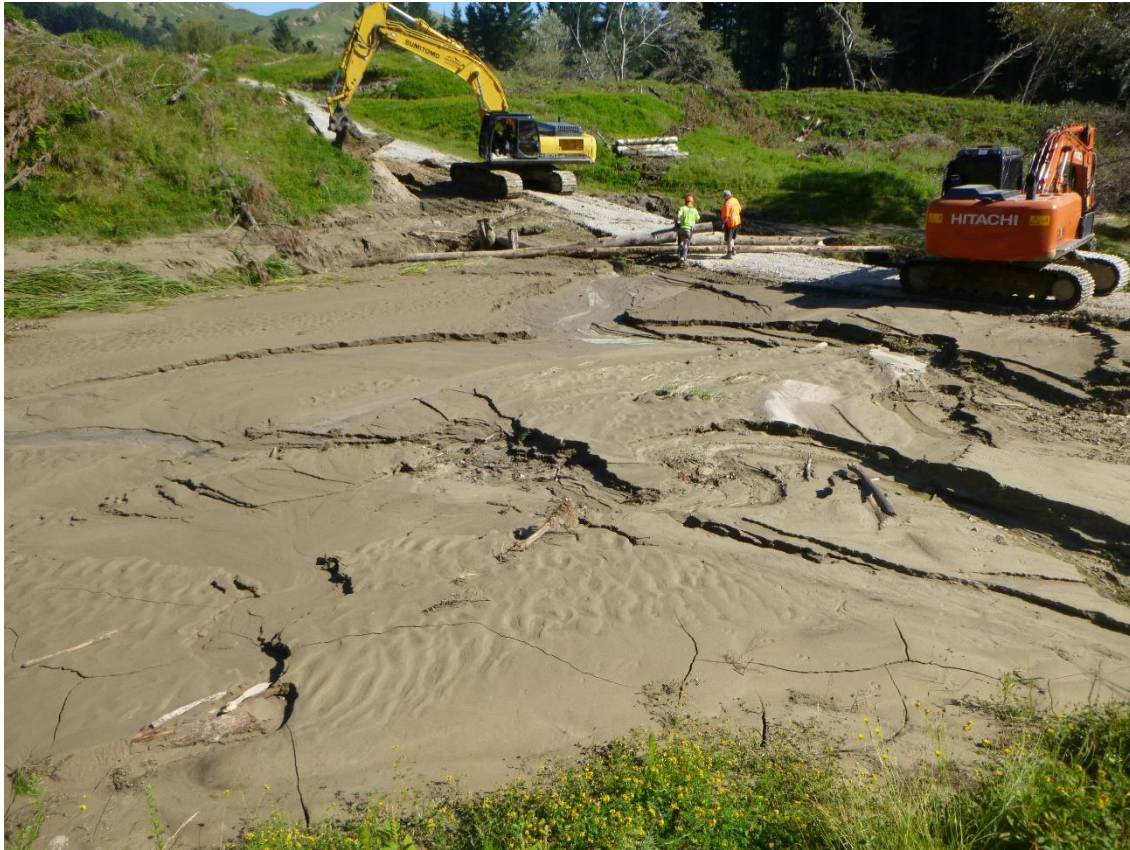
Photo 21: Tahurua Earthmovers undertaking repairs to the temporary crossing at the 3km marker on Mad Mutt Road following cyclone Gabrielle.
