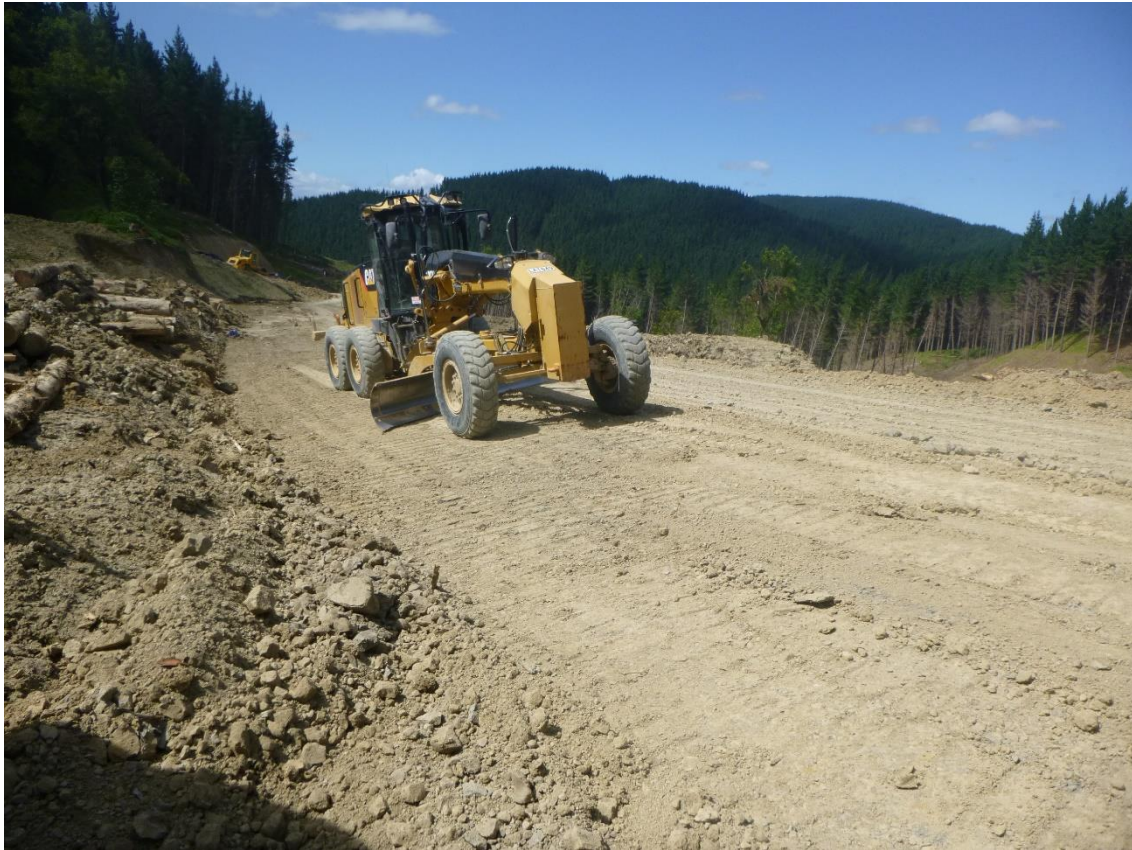
Photo 15: Taurua Earthmovers constructing Mad Mutt Road between Landings 9 and 10.
