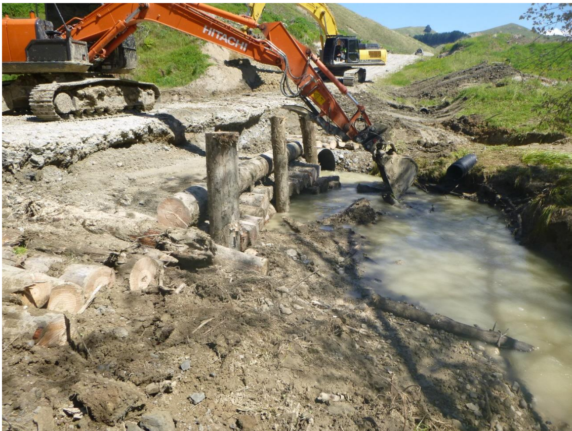
Photo 22: Tahurua Earthmovers undertaking repairs to the temporary crossing at the 3km marker on Mad Mutt Road following cyclone Gabrielle.
