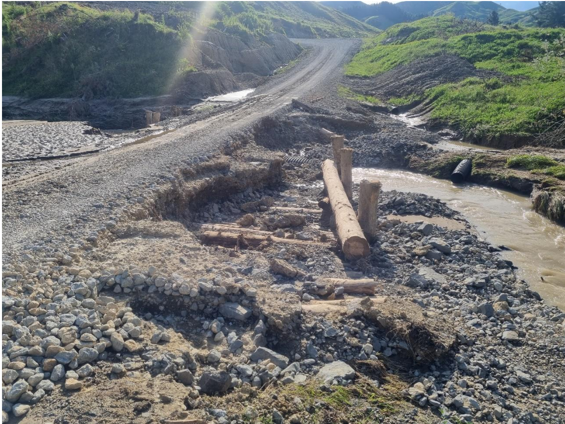
Photos 25 & 26: Further damage to the temporary crossing at the 3km marker on Mad Mutt Road following a second rain event.
