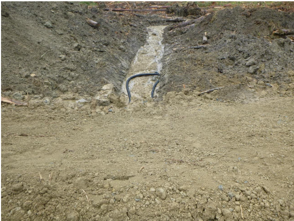
Photo 10: Tahurua Earthmovers constructing Mad Mutt Road between Landings 9 and 10 and extra drainage pipes installed.
