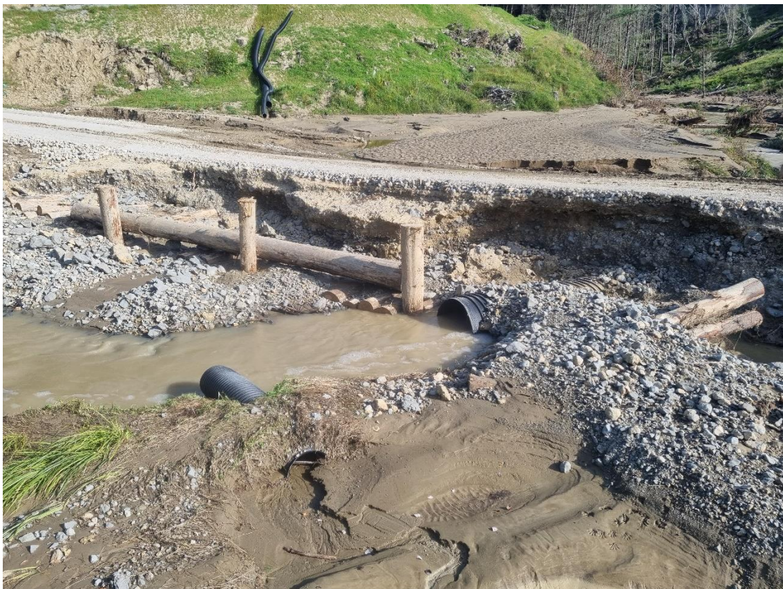
Photos 25 & 26: Further damage to the temporary crossing at the 3km marker on Mad Mutt Road following a second rain event.
