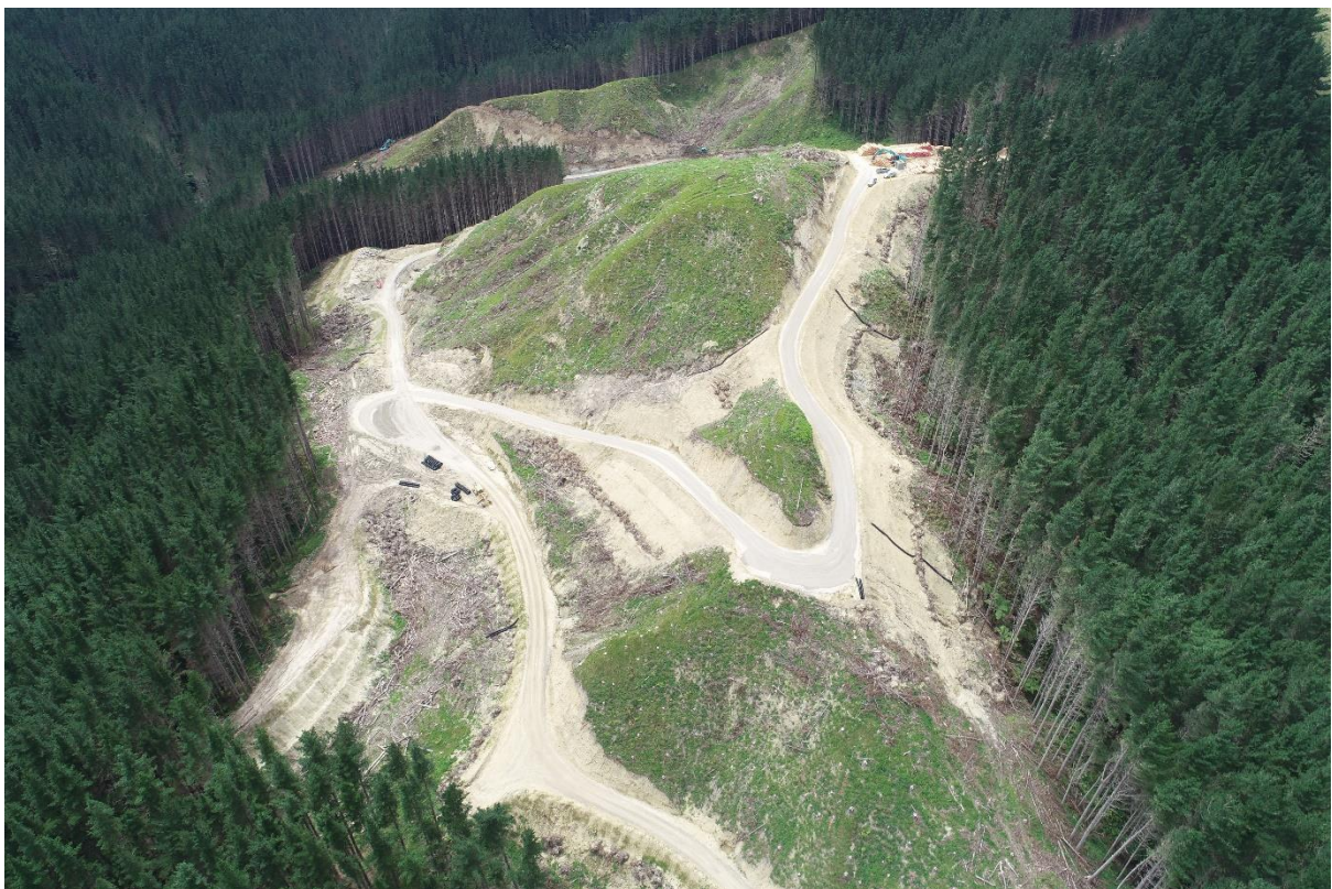
Photo 4: Aerial view of Outlook Road showing engineering work at top left and harvest operations at top right.
