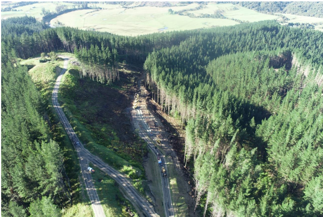
Photo 4: Aerial shot of the roadlining operation on Caulfield Road.
