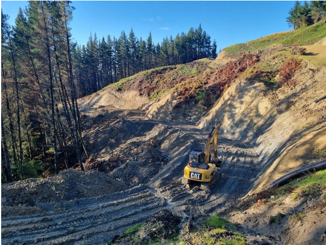
Photo 3: Road formation on Hutchinson Road.
