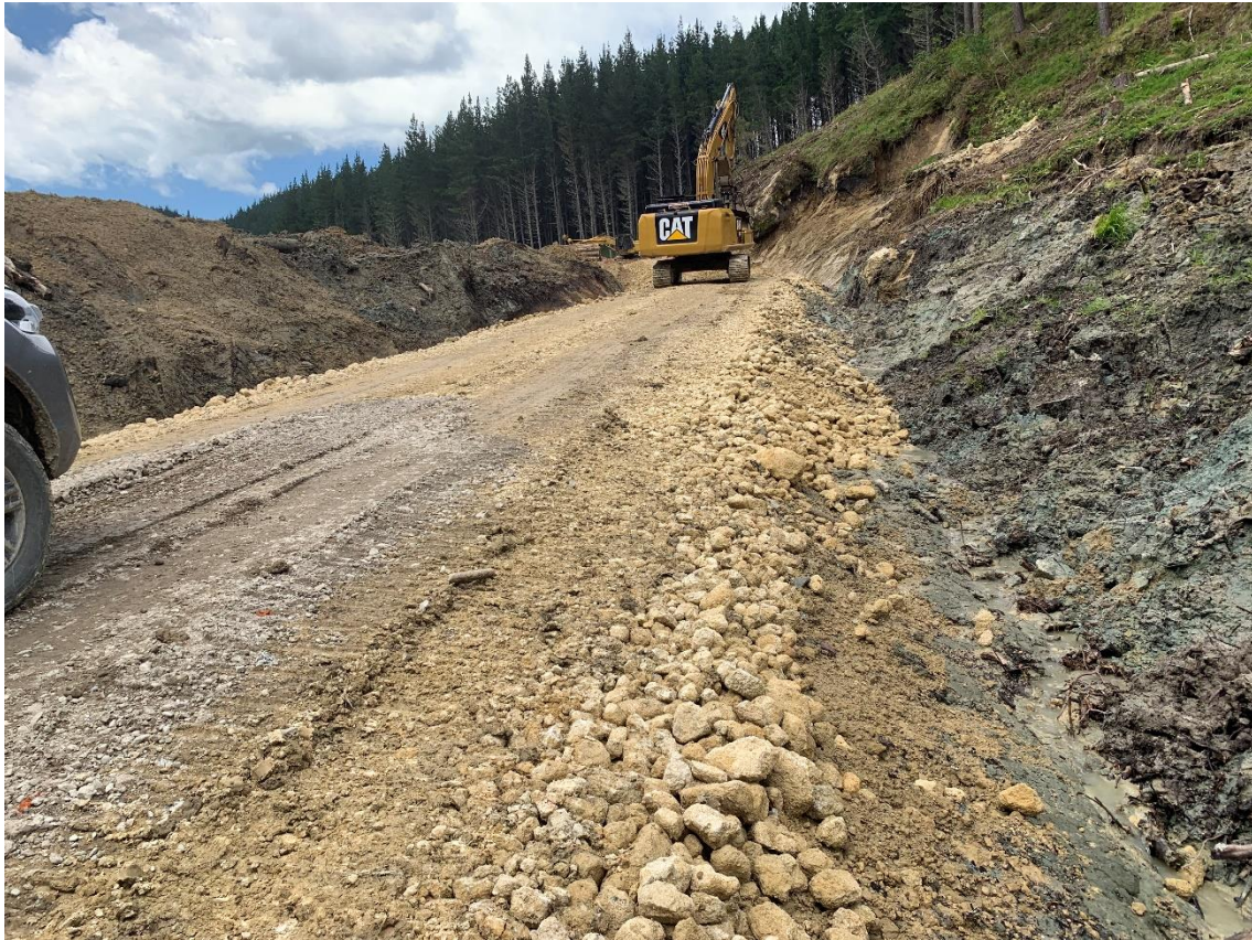
Photos 3 & 4: Excavator paving Griffiths Road.
