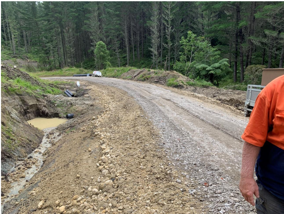
Photo 2: Finished section of Griffiths Road.
