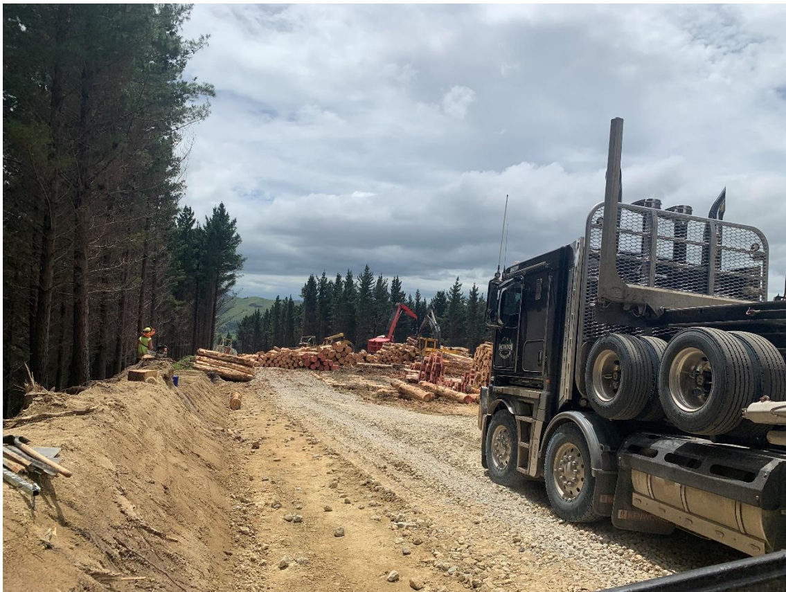
Photo 6: Log 16 working on Landing 49.
