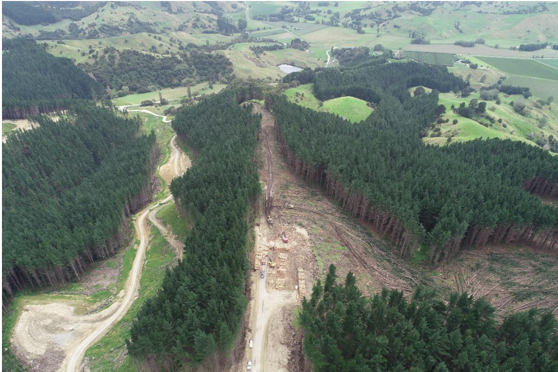
Photo 3: Log 16 working on Landing 49. Lee Pee Road to the left of photo. Landing 49 and corridor to Landing 50 middle of photo and corridor to Landing 51 to the right of photo.
