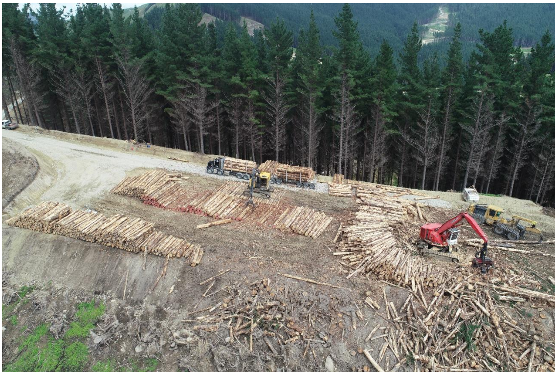
Photo 2: Log 16 operations on Landing 49, Lee Pee Road.
