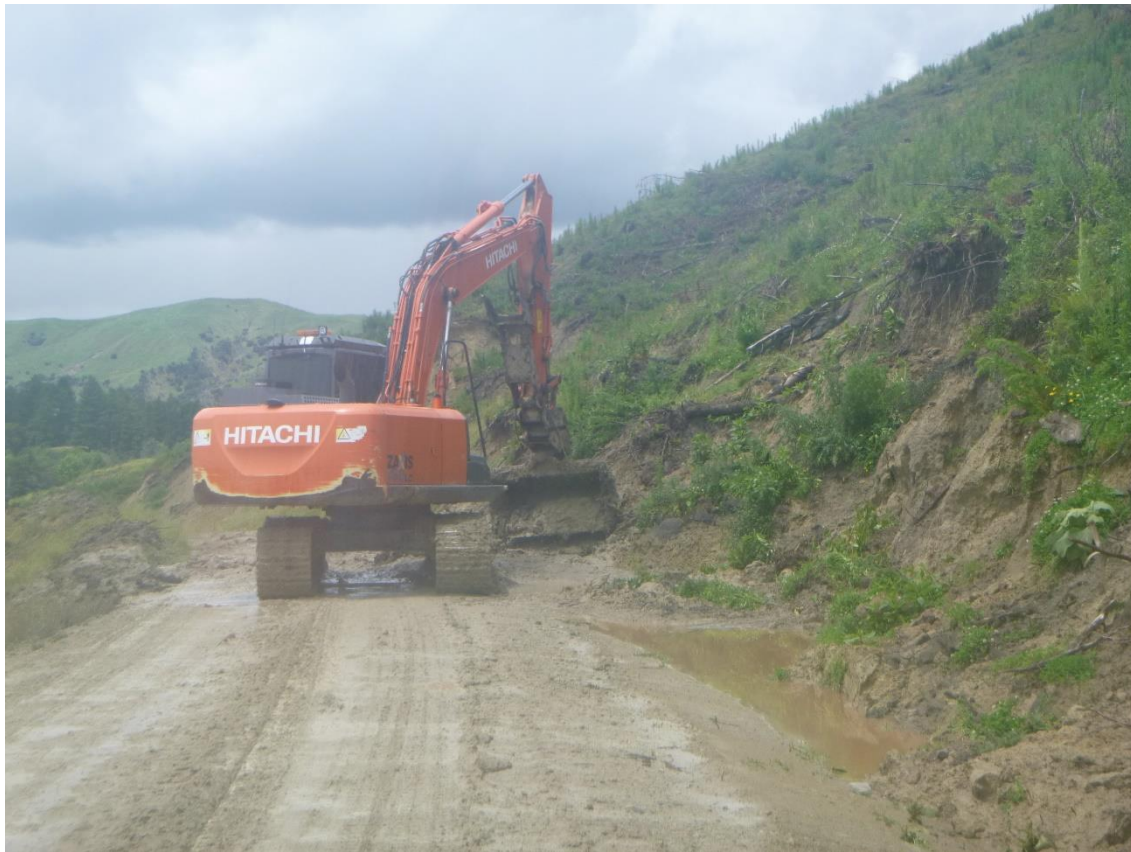
Photos 27 & 28: Tahurua Earthmovers completing maintenance on Mad Mutt Road following Cyclone Hale – clearing slips.
