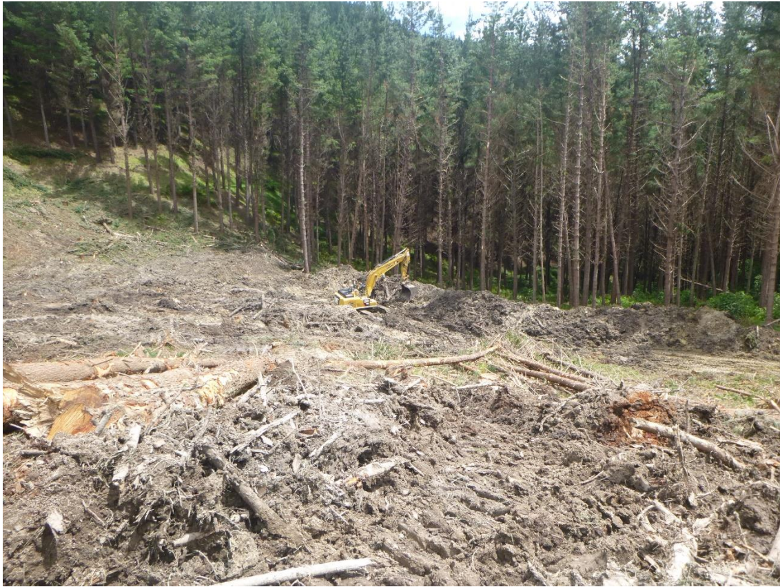
Photos 9 & 10: Tahurua Earthmovers constructing Landing 10 – stripping off slash and root balls.
