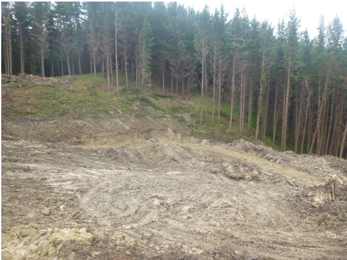
Photos 9 & 10: Tahurua Earthmovers constructing Landing 10 – stripping off slash and root balls.
