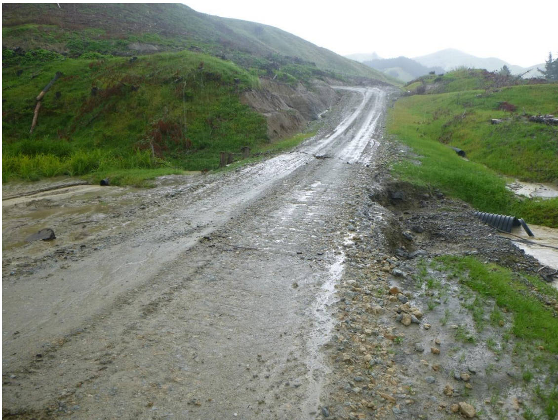
Photo 30: Tahurua Earthmovers completing maintenance on Mad Mutt Road following Cyclone Hale – repairing temp crossing.
