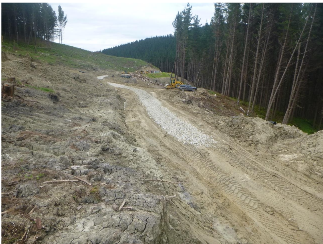
Photo 19: Tahurua Earthmovers beginning metalling Coates Road from Landing 8 to 9A.
