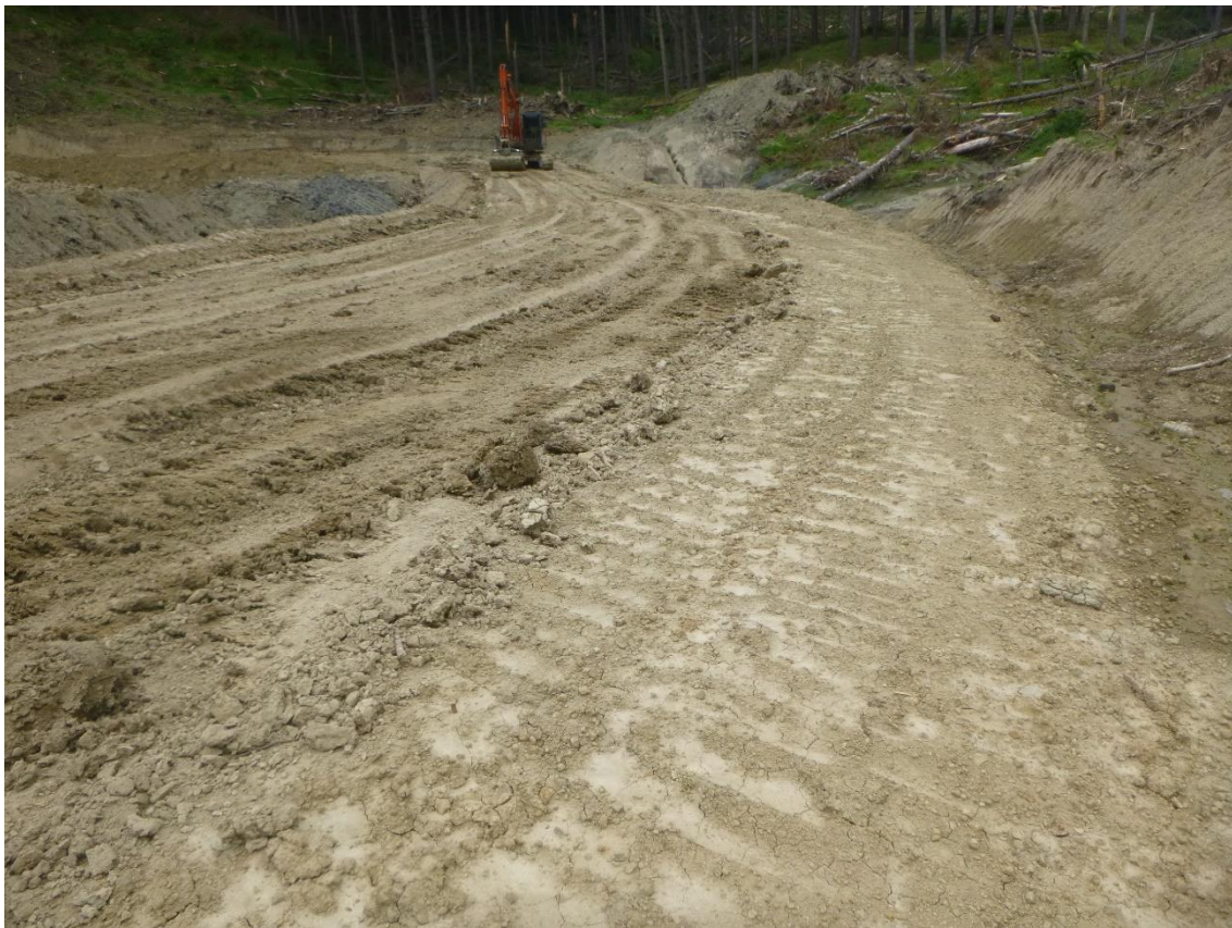
Photo 18: Tahurua Earthmovers cleaning up Coates Road ready for metalling.
