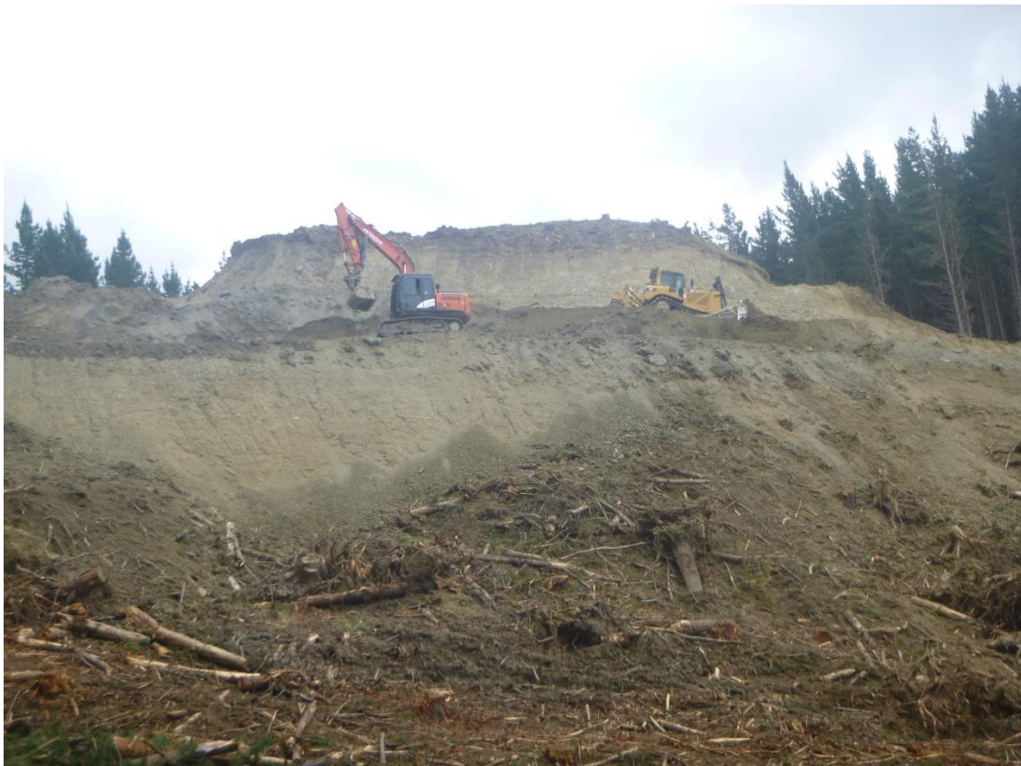
Photo 24: Tahurua Earthmovers constructing Mad Mutt Road between Landing 9 and 10.
