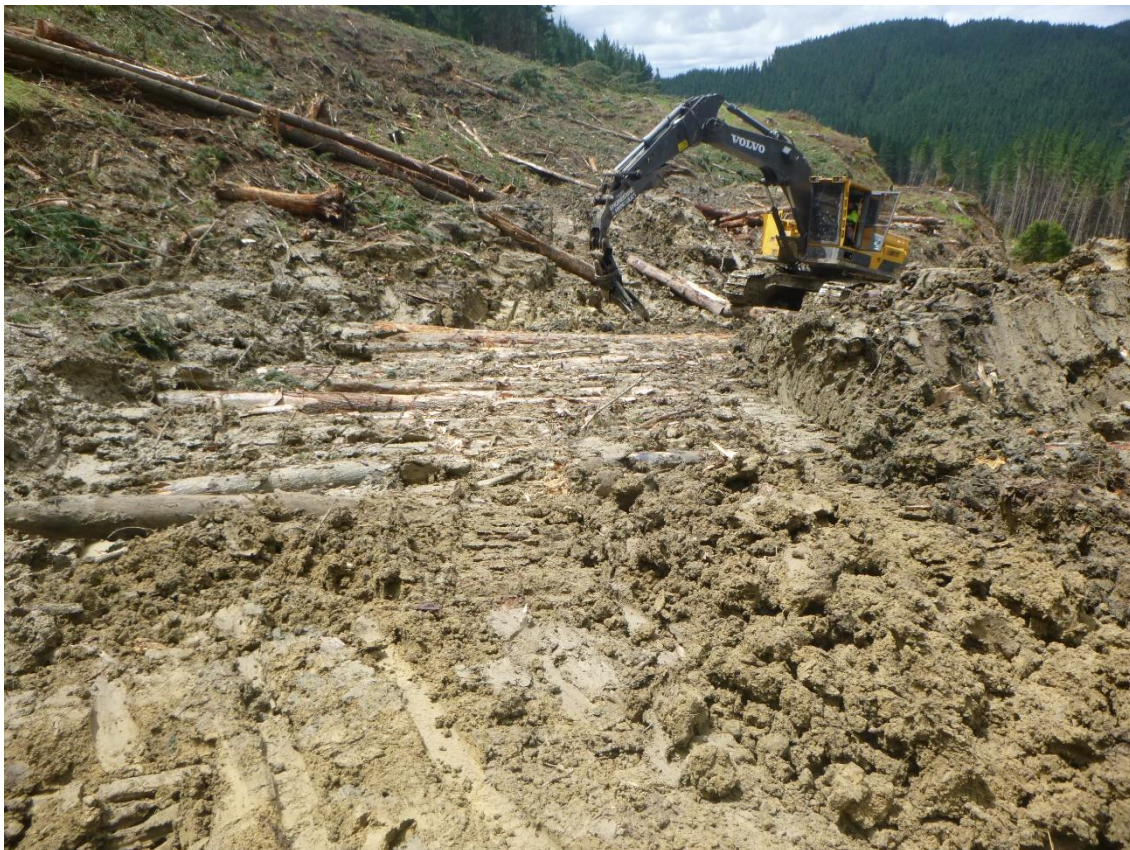
Photo 4: A & R Logging crew, Log 19 laying corduroy from old toppling on the haul track in Setting 500 for extraction back to Landing 9, as machines were getting stuck.
