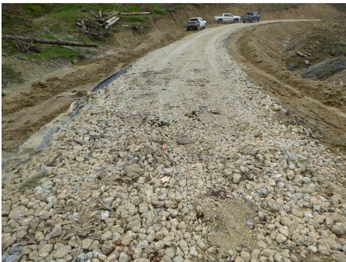
Photo 20: Tahurua Earthmovers metalling Coates Road over the top of geotextiles where the ground was soft.
