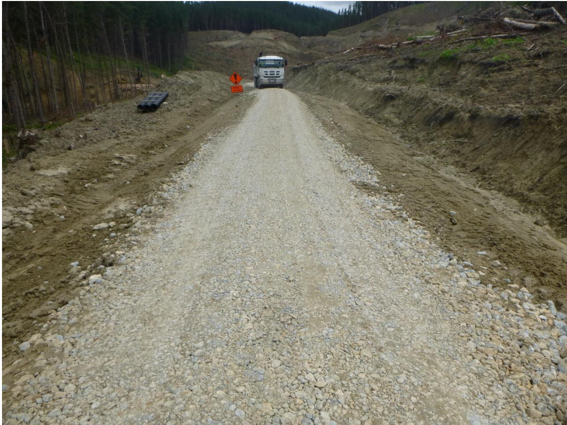
Photo 21: Tahurua Earthmovers metalling Coates Road from Landing 8 to 9A.
