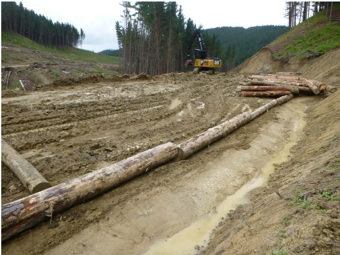
Photo 22: A & R Logging, Log 19 setting up Landing 9A and laying corduroy.
