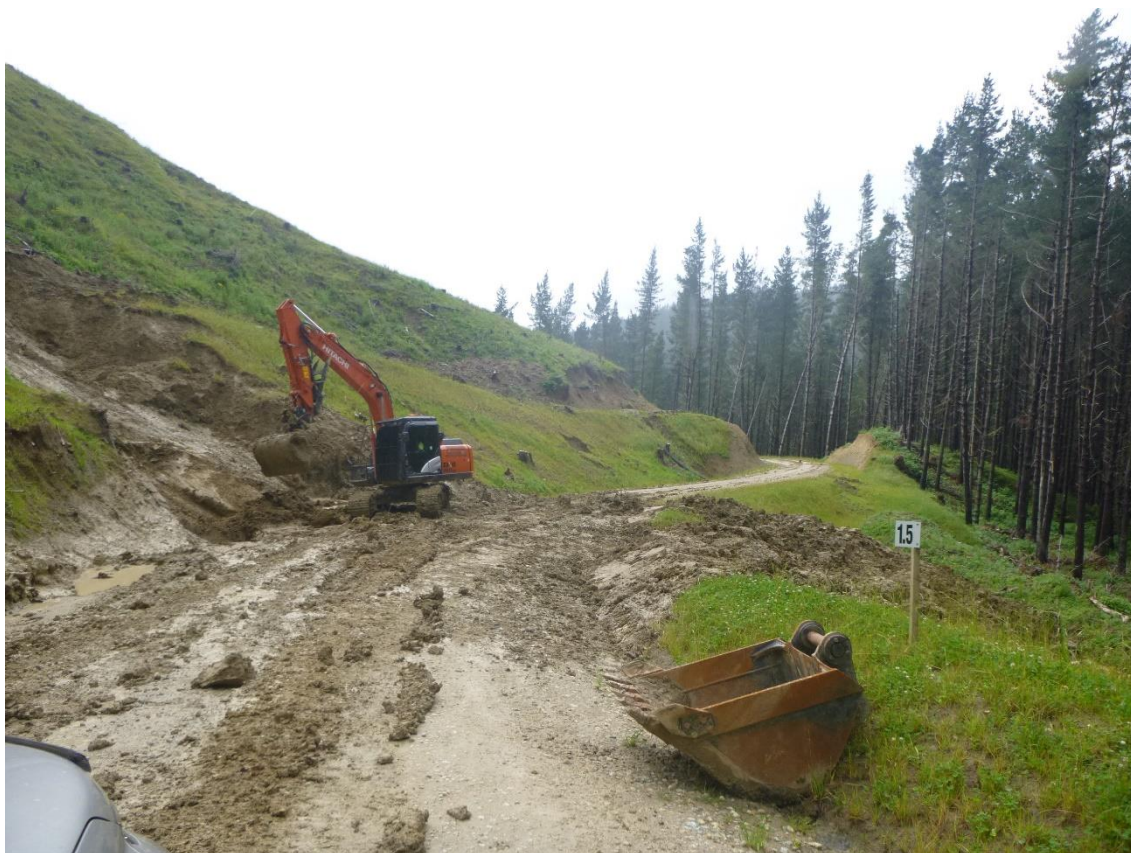
Photos 27 & 28: Tahurua Earthmovers completing maintenance on Mad Mutt Road following Cyclone Hale – clearing slips.
