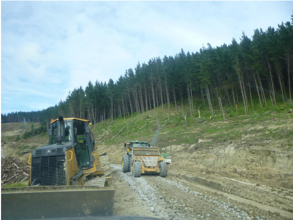
Photo 29: Tahurua Earthmovers completing maintenance on Mad Mutt Road following Cyclone Hale – traction spreads on metal.
