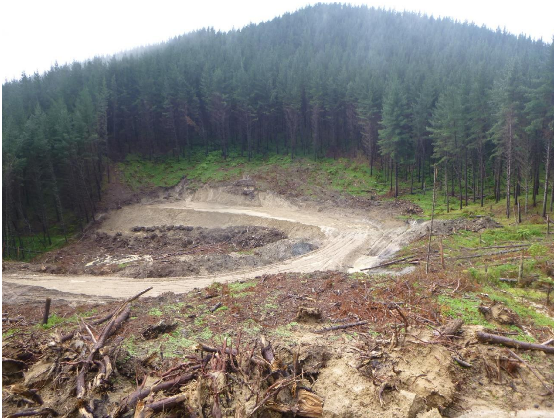
Photo 17: Tahurua Earthmovers constructed Landing 9A on Coates Road.
