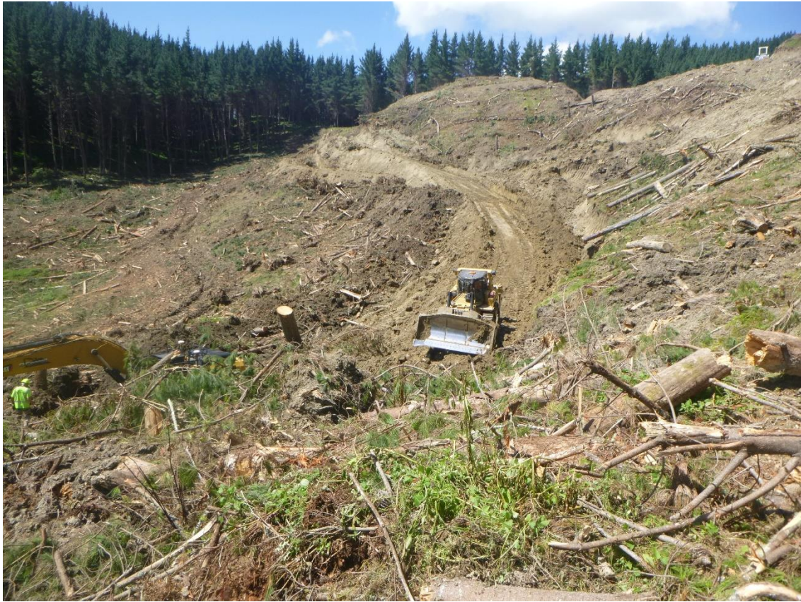
Photo 23: Tahurua Earthmovers in the early stage of constructing Mad Mutt Road between Landing 9 and 10.
