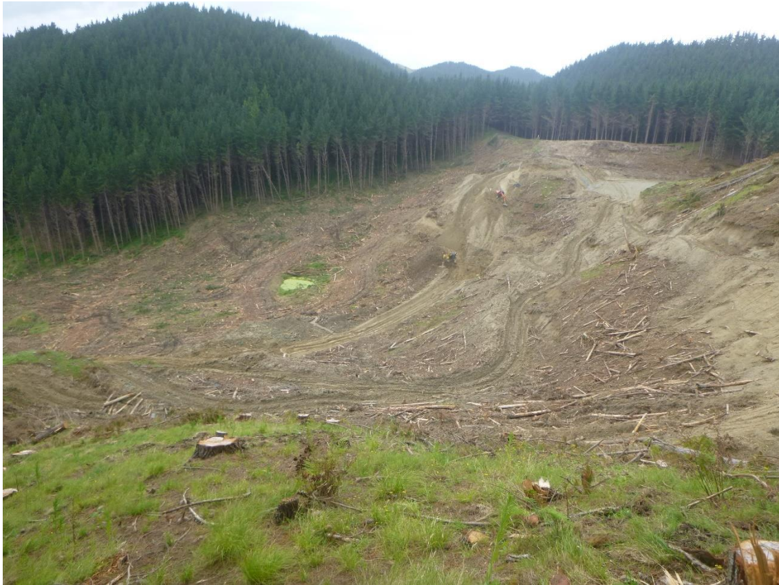
Photo 25: Tahurua Earthmovers constructing Mad Mutt Road between Landing 9 and 10.
