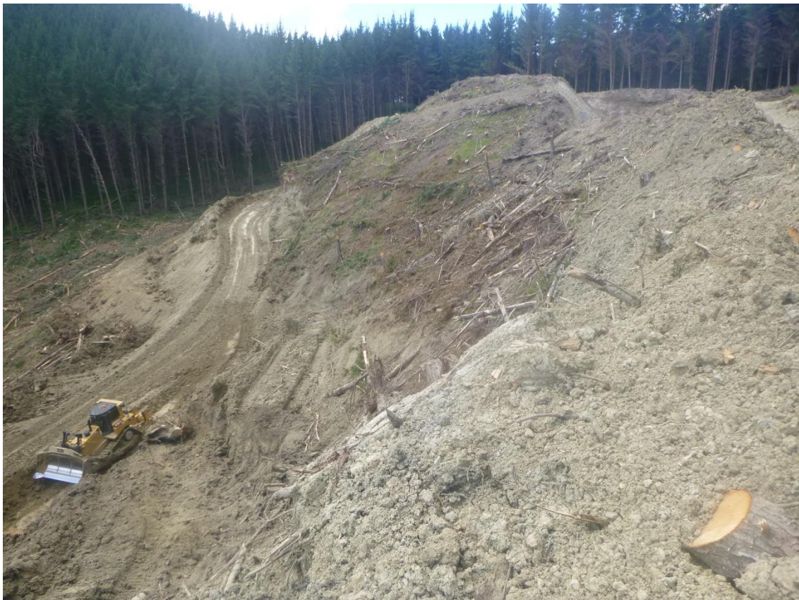
Photo 26: Tahurua Earthmovers constructing Mad Mutt Road between Landing 9 and 10.
