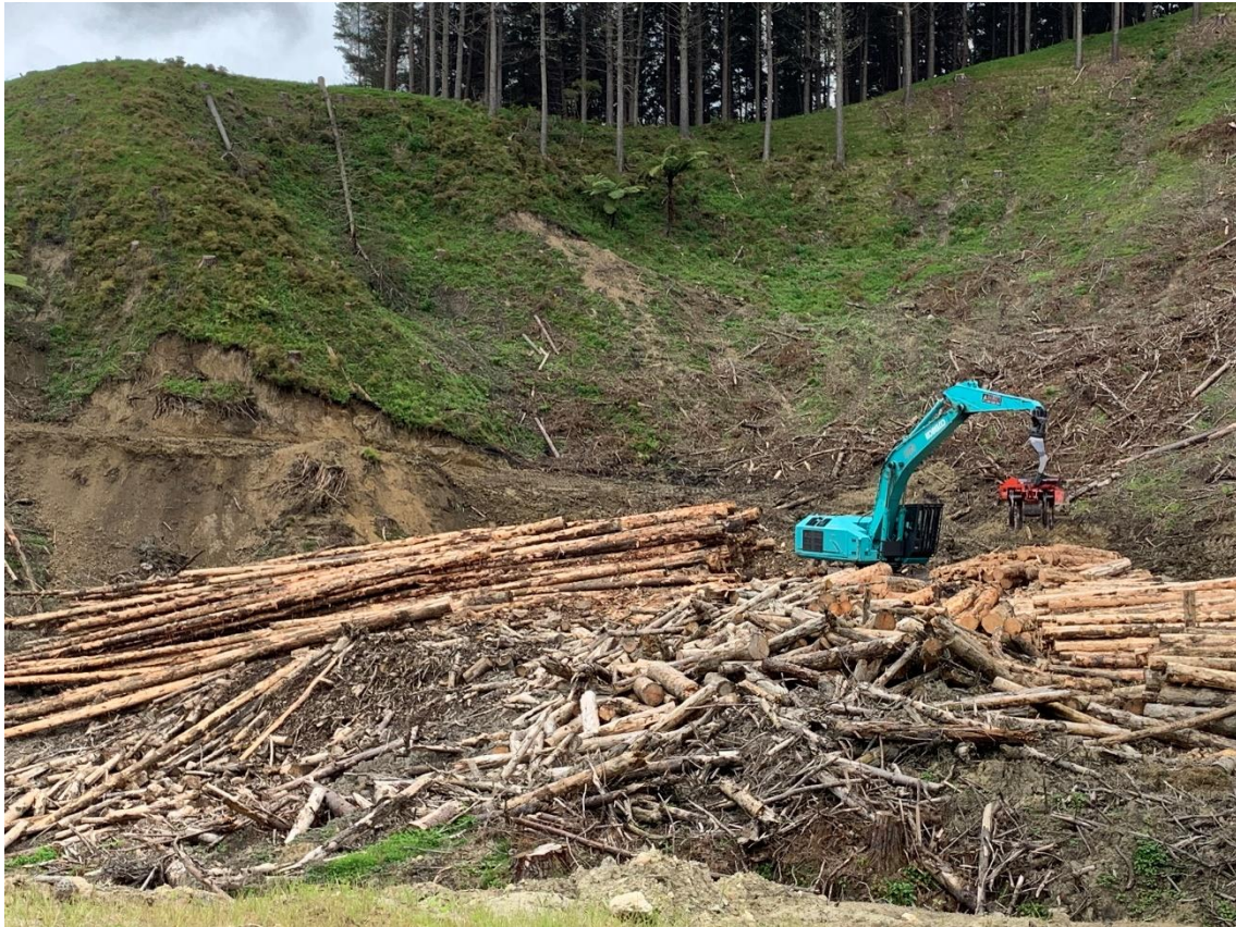
Photo 1: Log 6 Kobelco 50T working on Temporary Landing 1.
