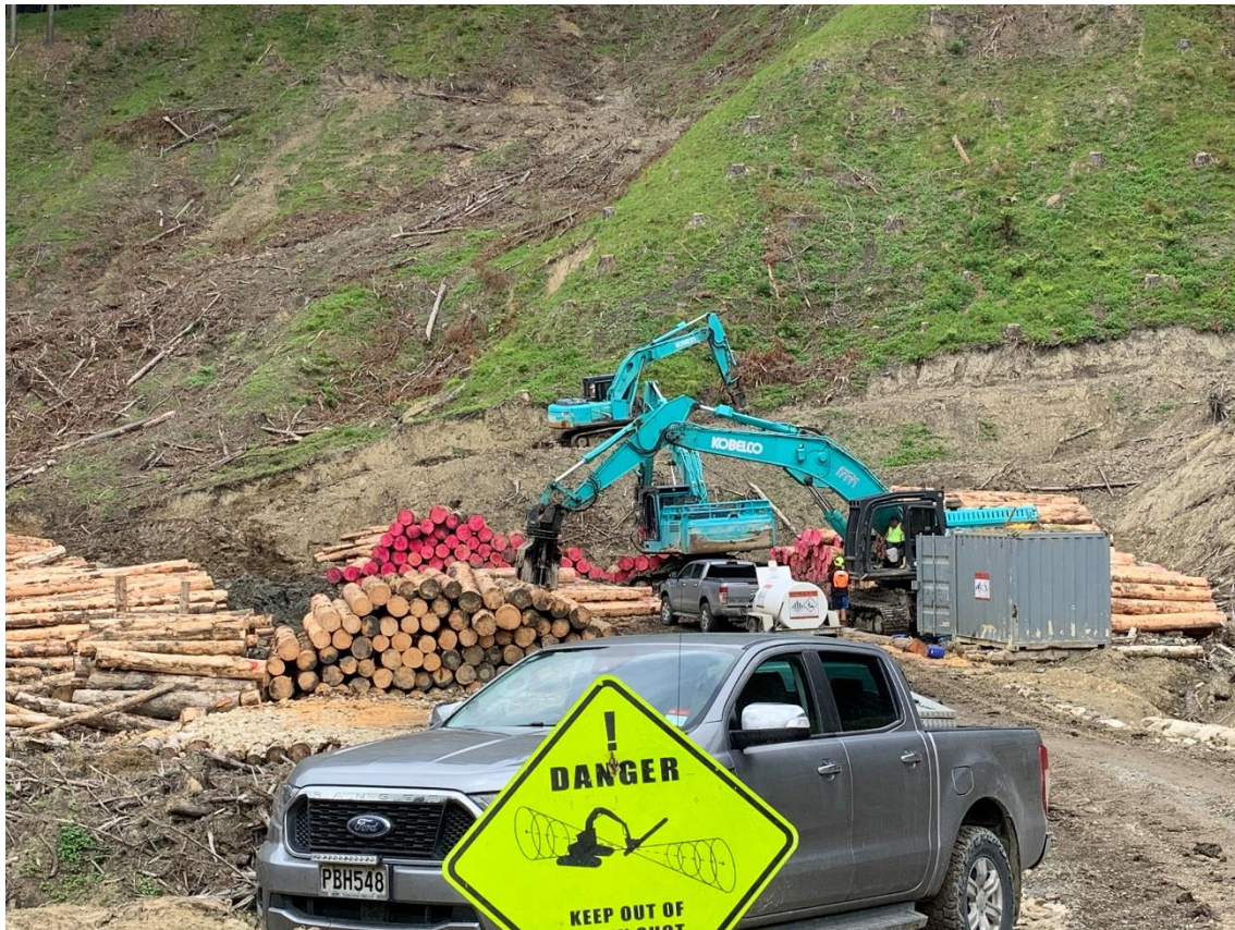
Photo 3: Log 6 crew working on Temporary Landing 1.
