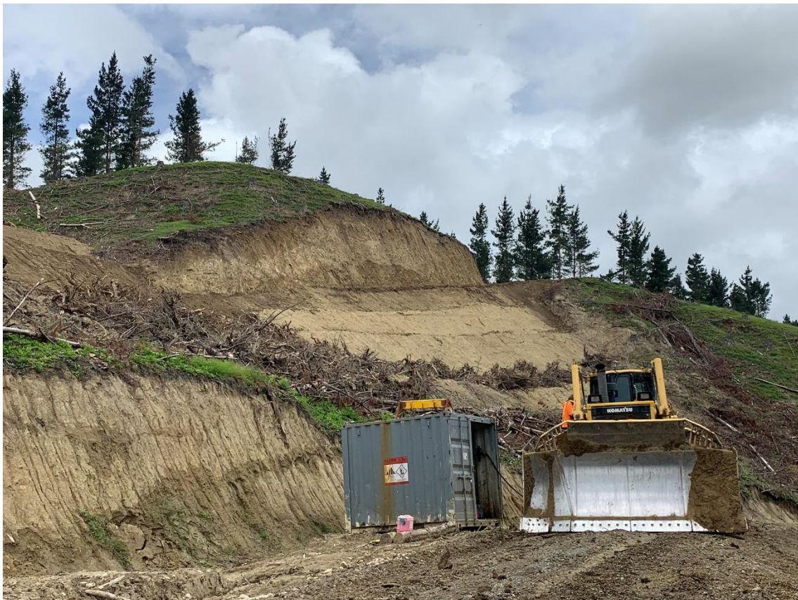
Photo 2: Komatsu bulldozer fuelling up.
