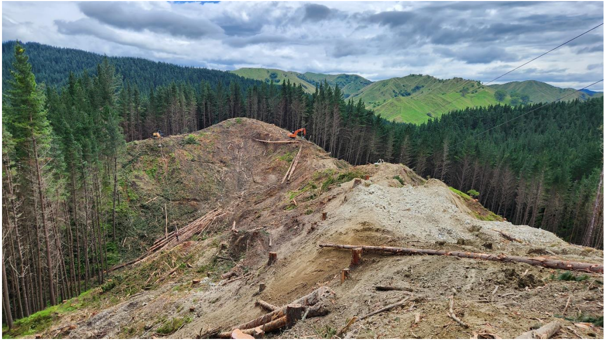
Photo 3: Nearing completion of harvesting work for Cairns Road, Landing 12, Setting 500.
