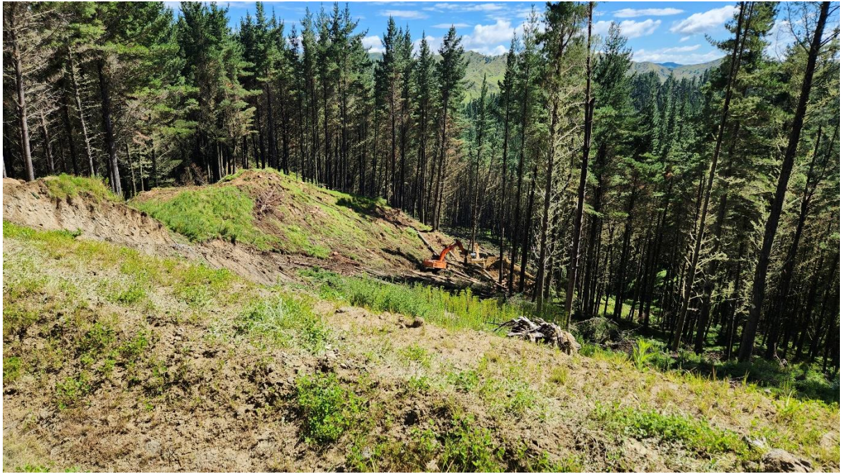
Photo 1: Setting 500 tracking for road benches and to aid in log extraction.
