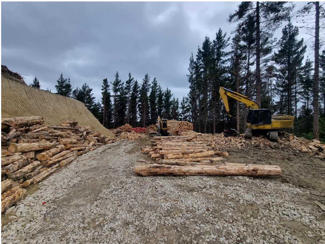
Photo 8: Small operation area on temporary landing for roadlining work.
