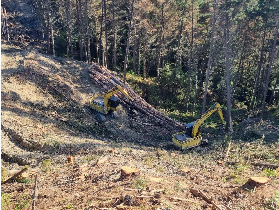
Photo 3: Loaders shovelling wood out of roadline corridor.
