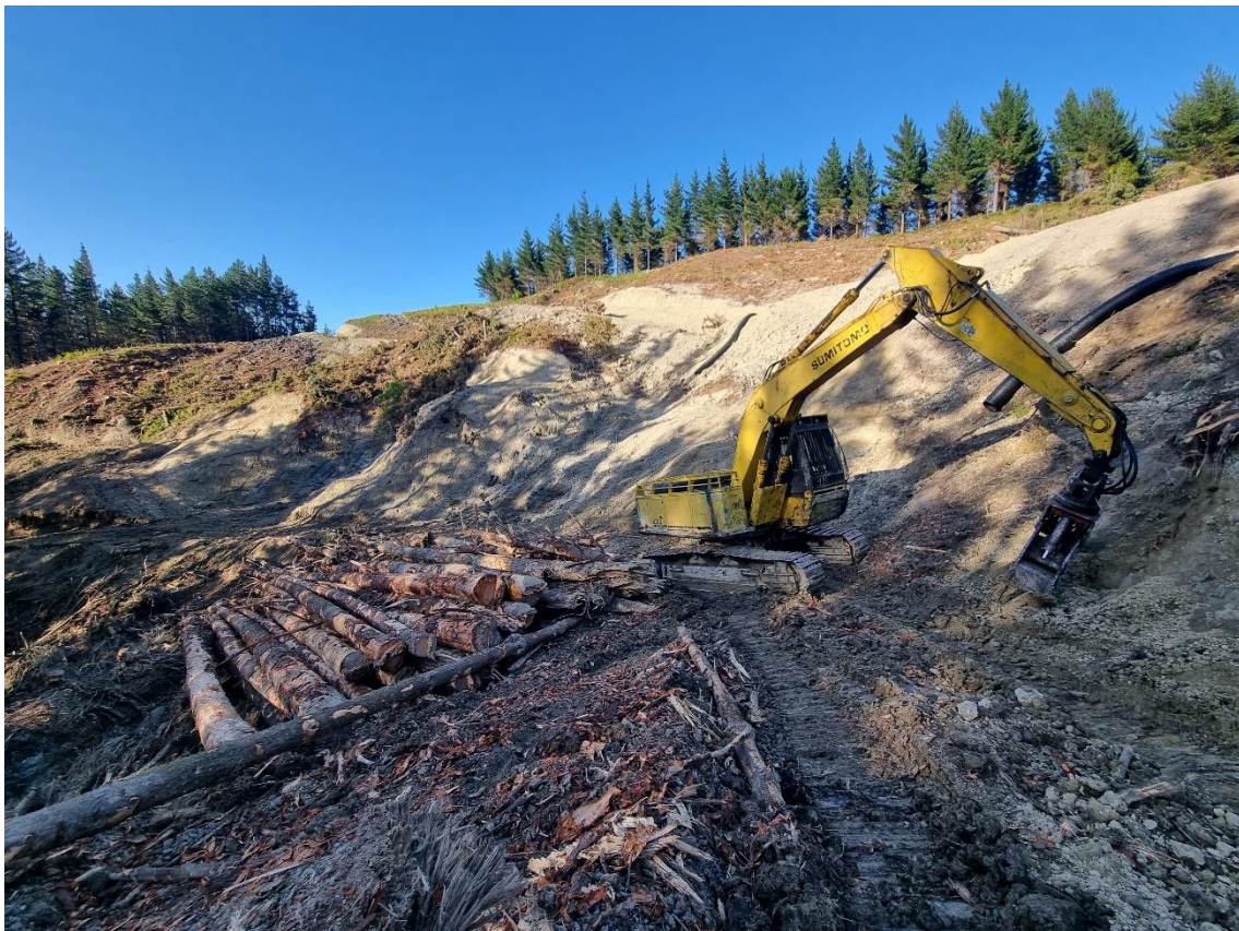
Photo 2: Shovel machine bringing heads out.
