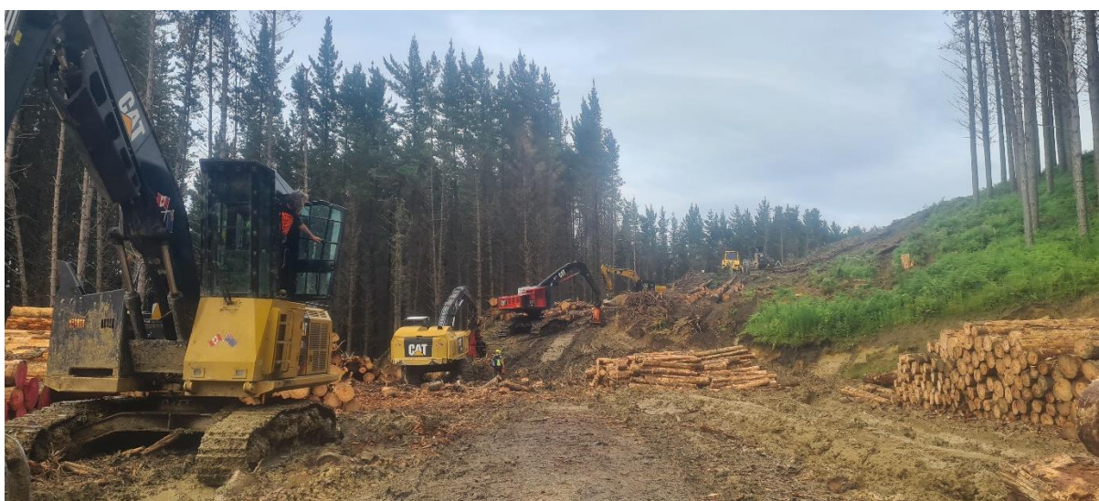
Photo 7: Harvesting and earthworks machinery from Landing 5 to 6 on Drury Road.
