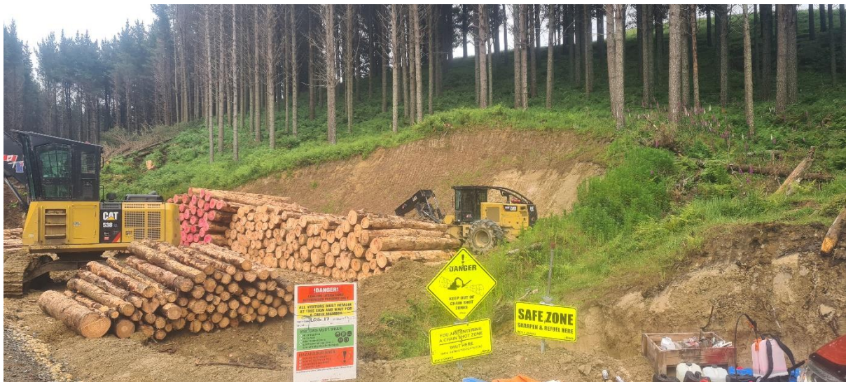
Photo 4: Landing 5 safety warning signs at the entrance.
