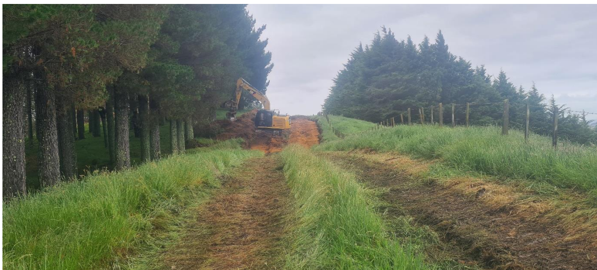
Photo 5: Clearing of topsoil to make way for road between Landings 6 and 7.
