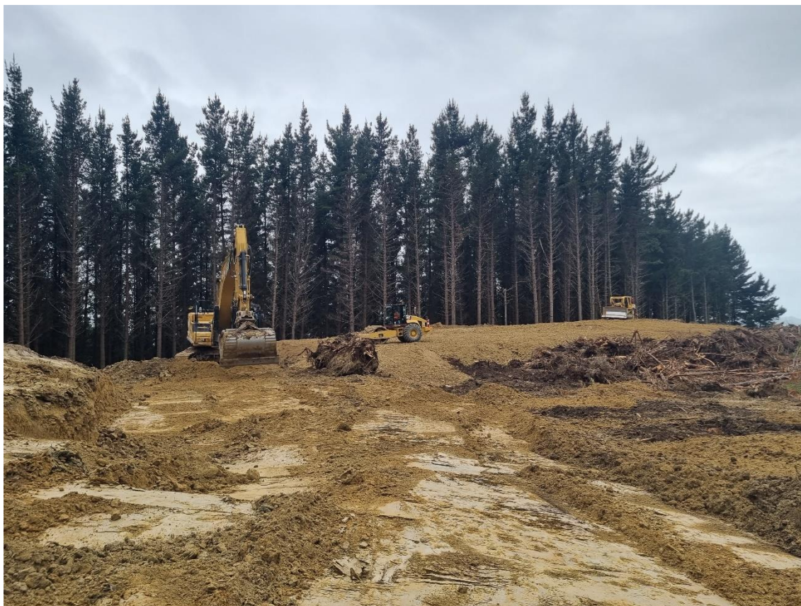
Photo 4: Earthworks operation building Landing 8 and road out.
