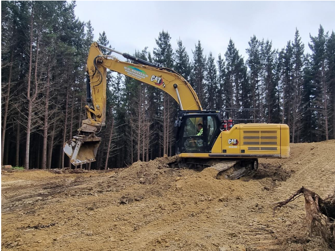
Photo 5: Neville Earthworks forming Landing 8.
