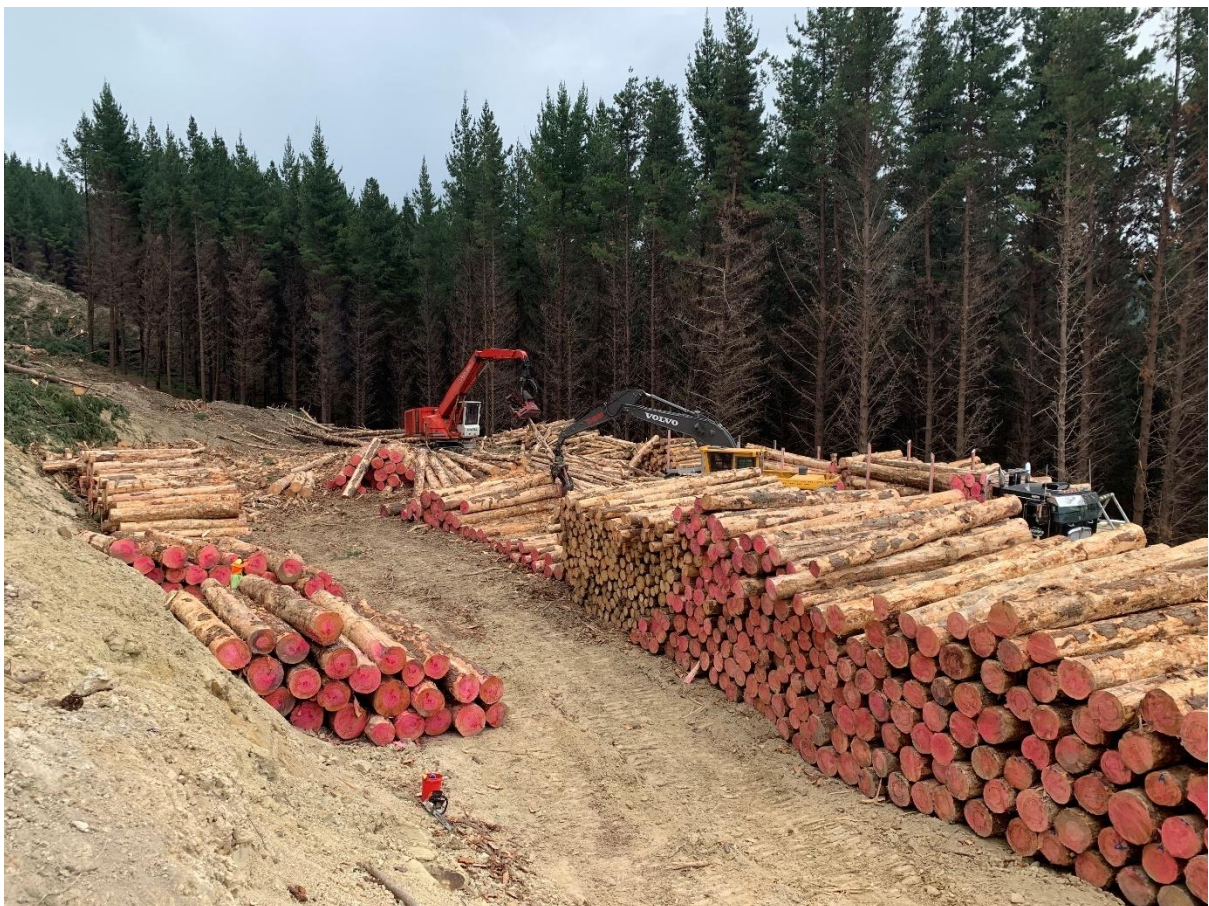
Photo 6: Log 16 operations on Temporary Landing 2, Basil Road.
