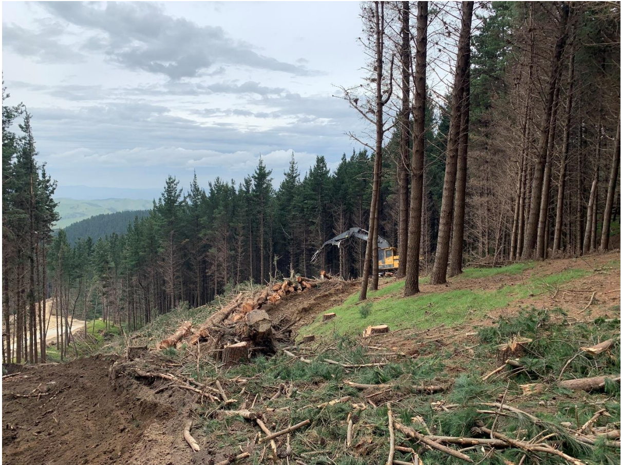
Photo 7: Log 16 shovel loader working in Setting 508.
