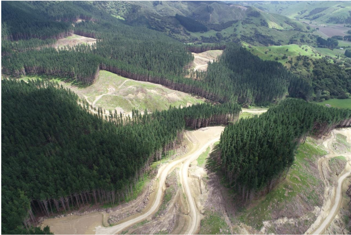
Photo 3: Good view of earthworks and some clearfell settings in Monterey.
