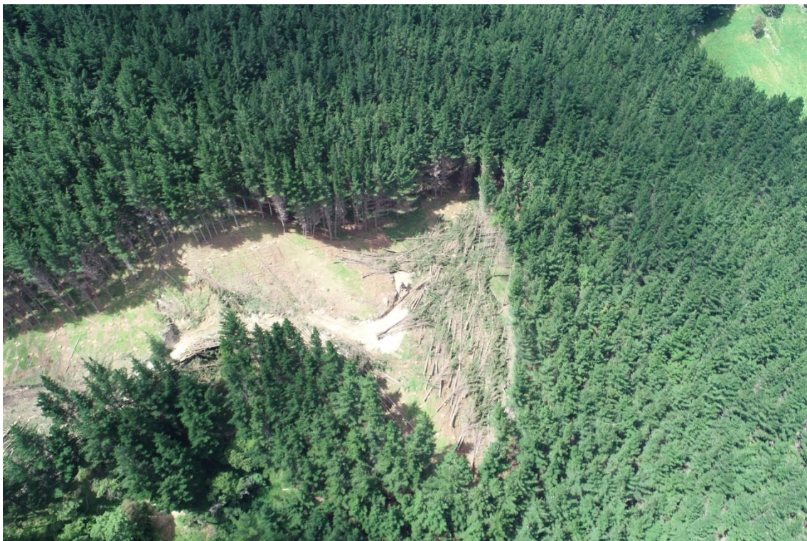
Photo 4: Log 16 Volvo loader shovelling in the area where Landing 48 will be built.
