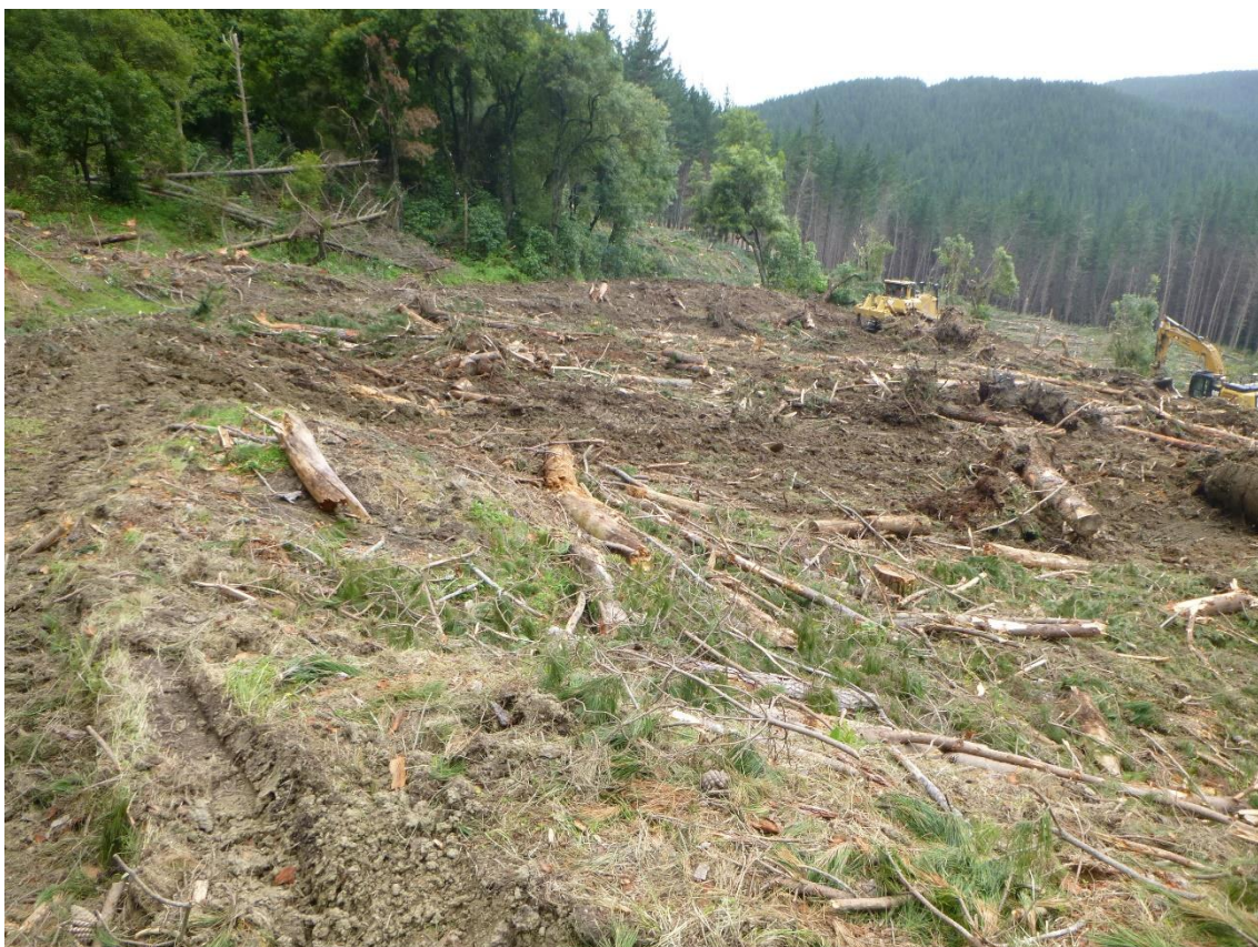
Photo 8: Tahurua Earthmovers stumping and slash stripping in preparation for the construction of Landing 9.
