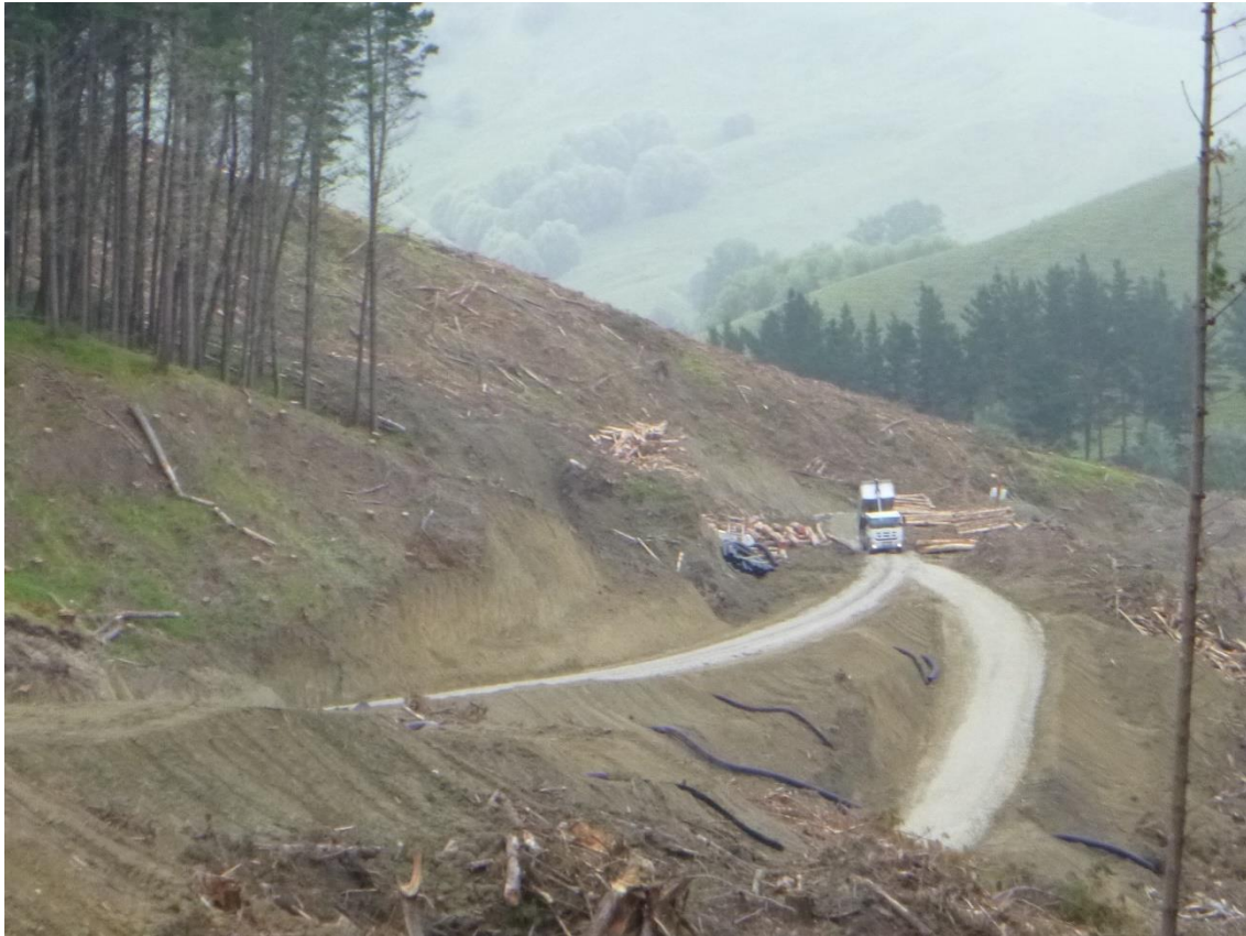
Photo 13: Tahurua Earthmovers laying traction spreads of metal through Landing 7 on Mad Mutt Road.
