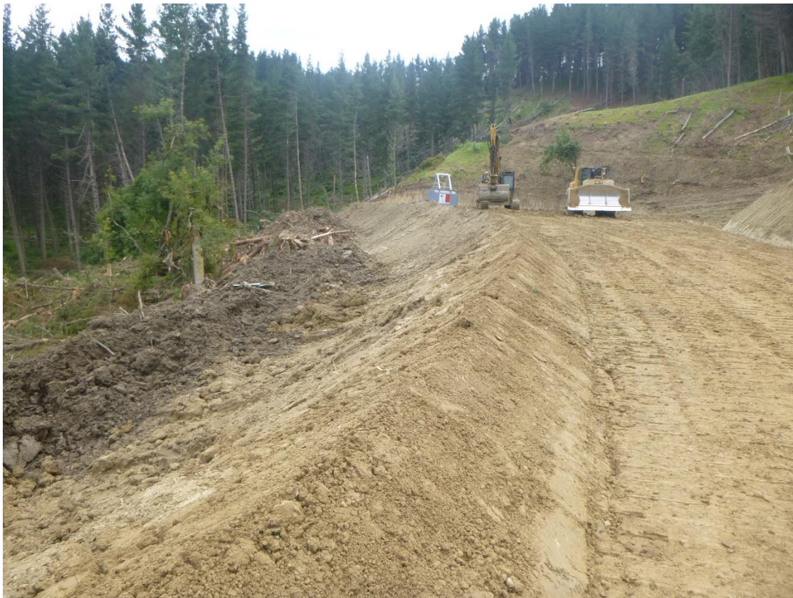
Photo 10: Tahurua Earthmovers recently formed stab road to Landing 9.
