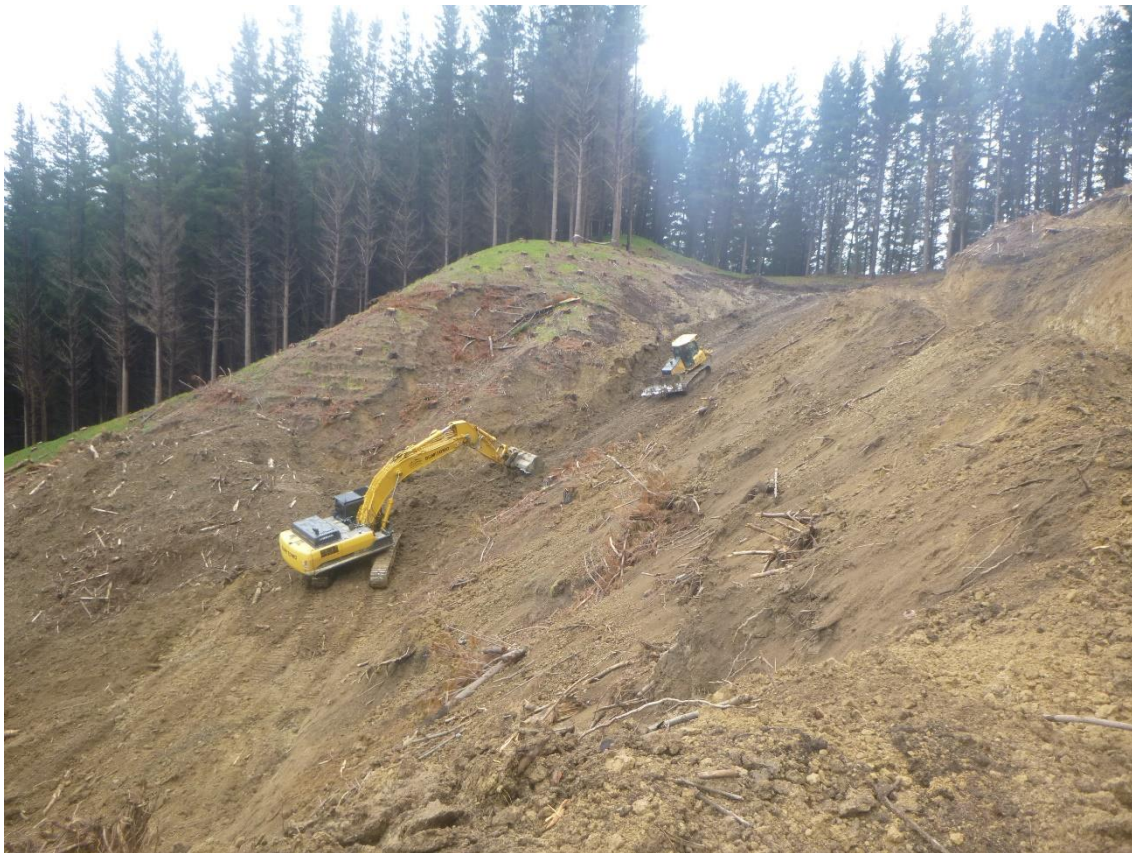
Photo 18: Tahurua Earthmovers partial construction of Landing 43 – stripping off poor material.
