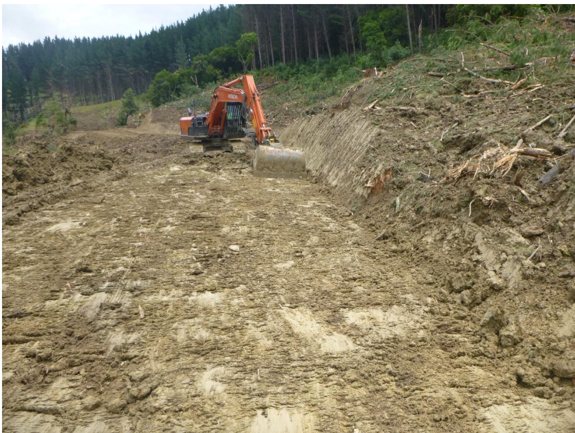
Photo 12: Tahurua Earthmovers shaping Mad Mutt Road between Landings 8 and 9.
