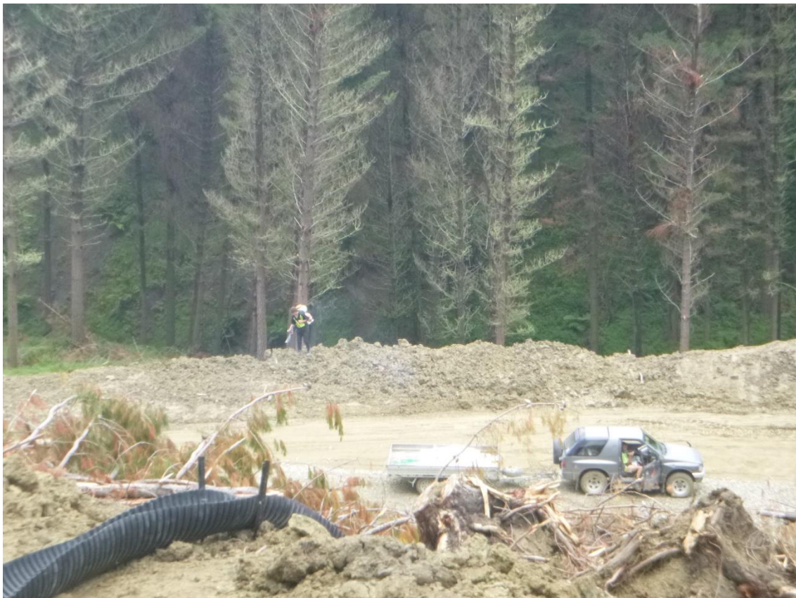
Photo 14: Tahurua Earthmovers grass seeding exposed earth on the road to Landing 39.
