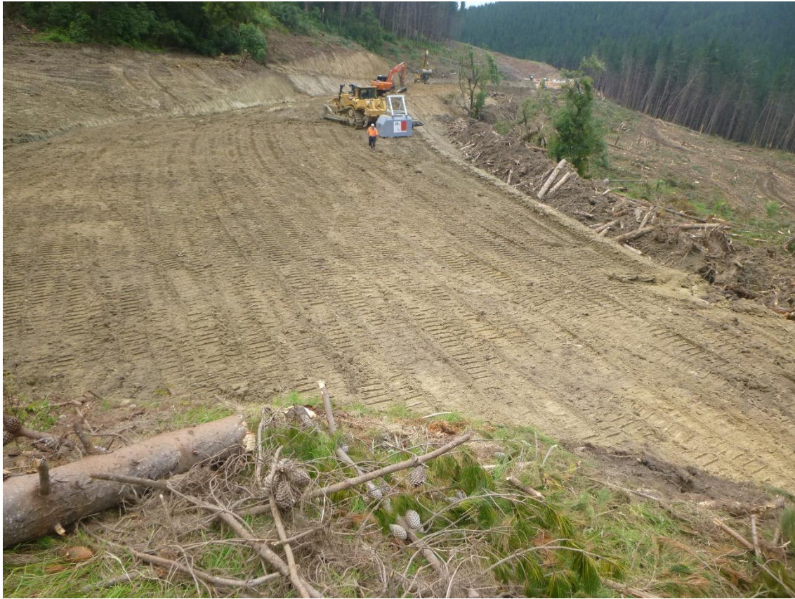
Photo 9: Tahurua Earthmovers constructed Landing 9.
