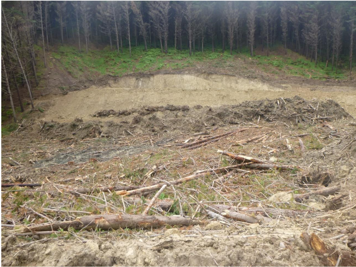
Photo 17: Tahurua Earthmovers partly constructed Landing 9A on Coates Road.
