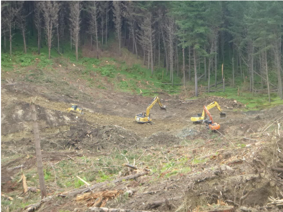
Photo 15: Tahurua Earthmovers slash stripping and early stage of constructing Landing 9A on Coates Road.
