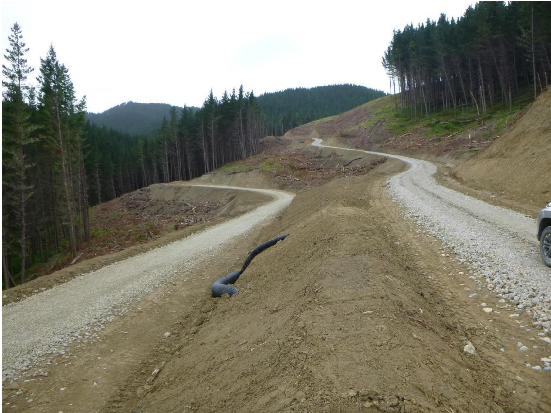
Photo 7: Tahurua Earthmovers formed and metalled road to Landing 39 and Mad Mutt Road from Landing 7 to 8.
