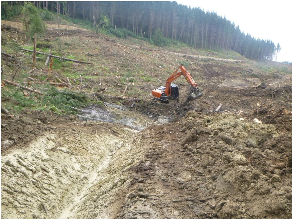
Photo 16: Tahurua Earthmovers preparing the site of a culvert installation on Coates Road.
