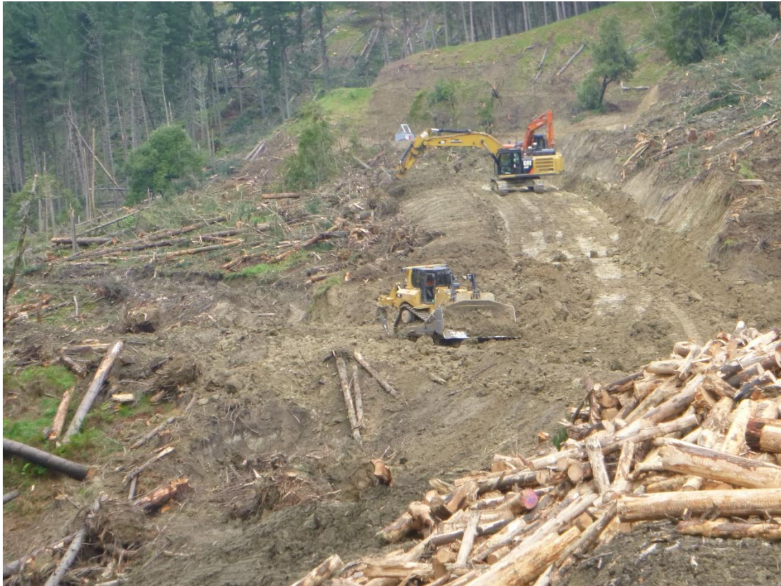
Photo 11: Tahurua Earthmovers forming Mad Mutt Road between Landings 8 and 9.
