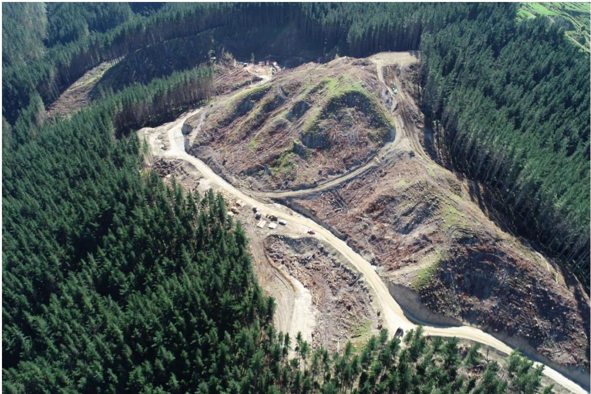
Photo 4: FRM crew, Log 6 working on Temporary Landing 1 at top of photo, 50T bucket digger benching Outlook Road, top right of photo.
