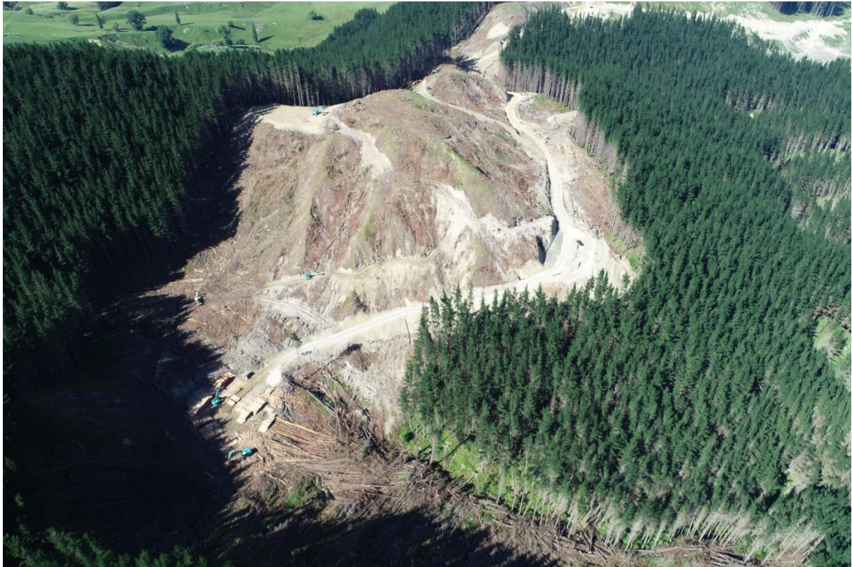
Photo 3: Log 6 working on Temporary Landing 1.
