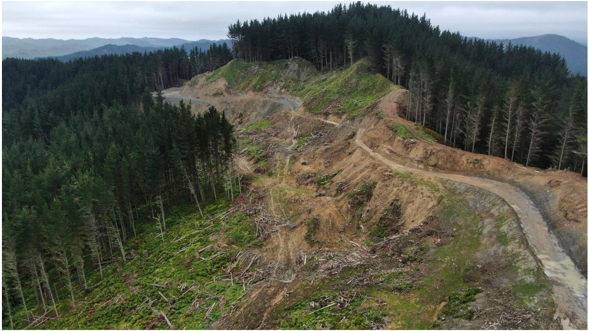
Photo 1: Aerial photo of the start of Wah Road, Setting 506.
