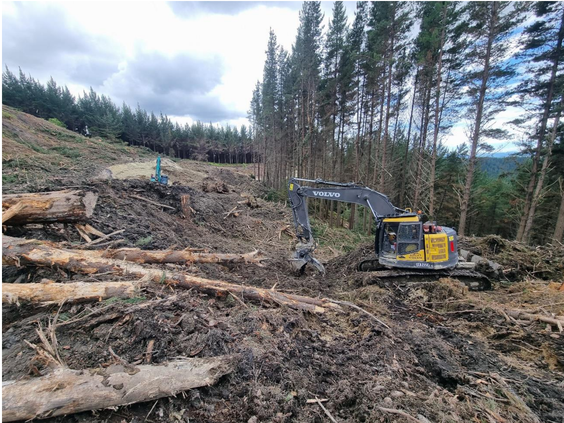
Photo 5: Road formation beginning off Clee Road down to Landing 31.
