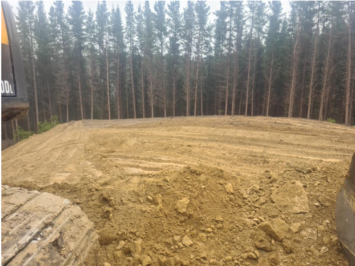
Photo 1: Landing 33 nearing completion.
