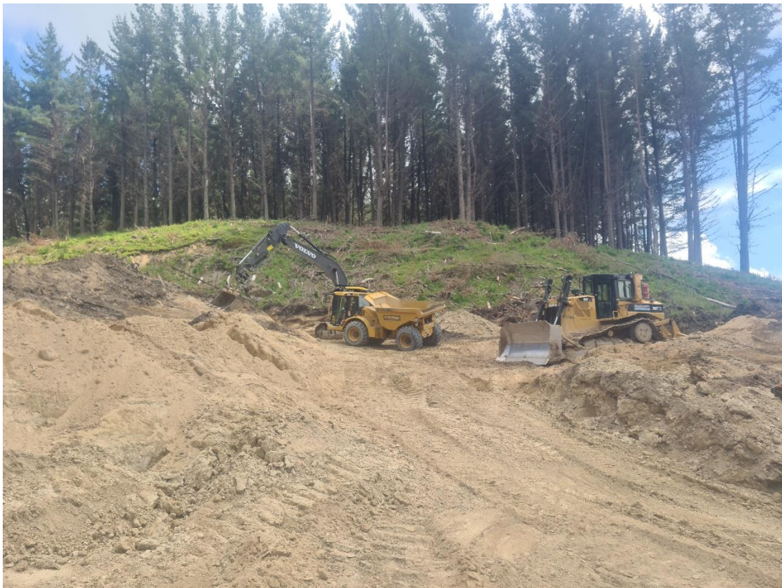
Photo 2: Construction of Drury Road.
