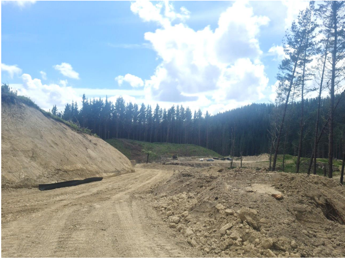
Photo 3: Fresh formation looking back from Landing 33 along Drury Road.
