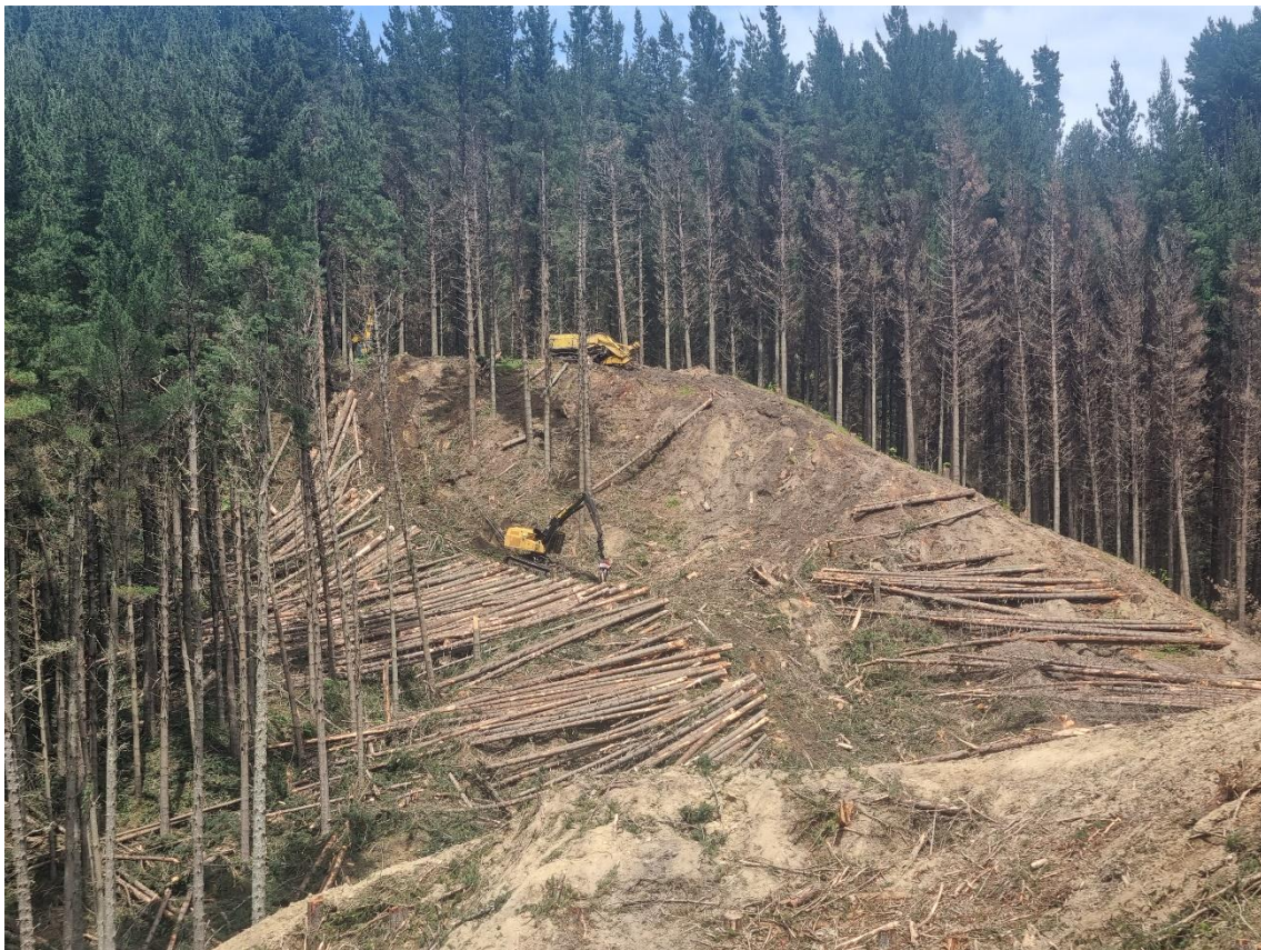
Photo 7: Tigercat feller buncher cutting roadline Setting 502.
