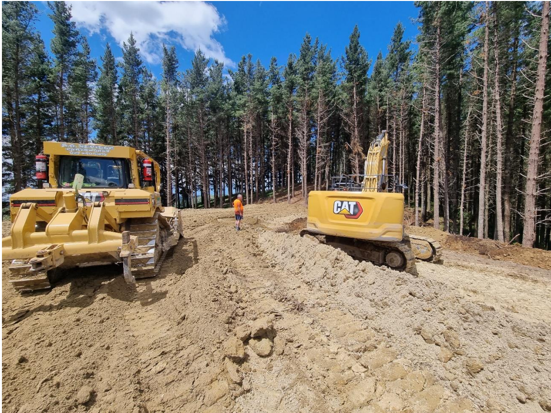
Photo 10: Earthworks machines forming Landing 6.
