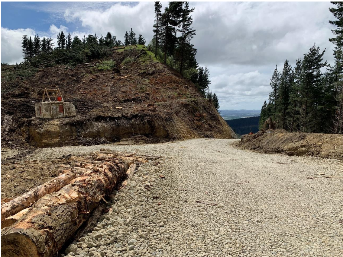
Photo 6: Well-formed section of Clarke Road.
