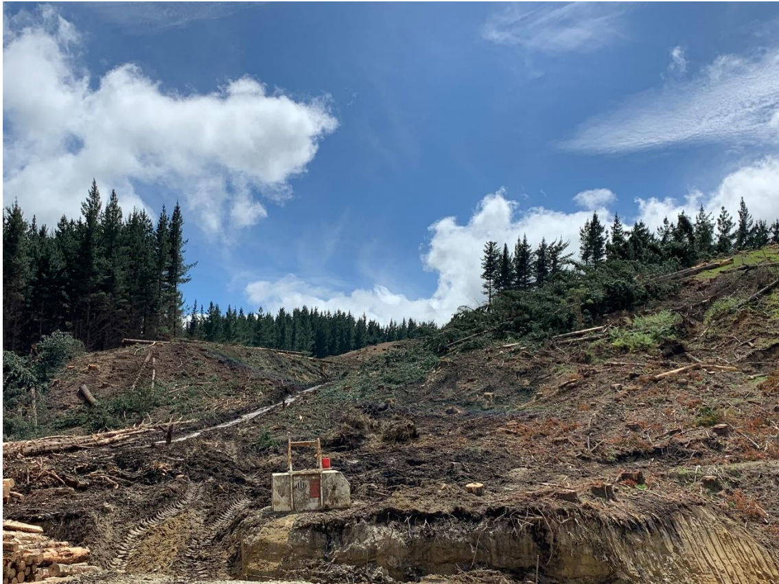
Photo 7: Looking out towards the area where Landings 21 and 21A will be built.
