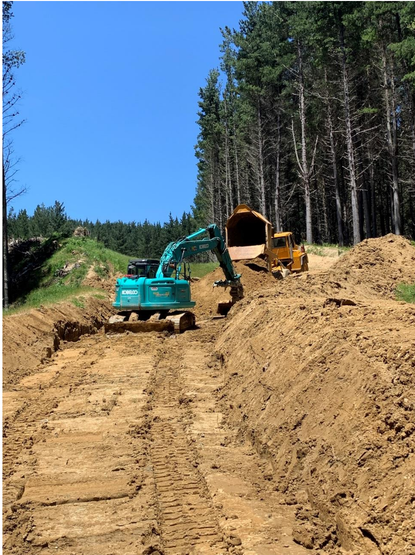
Photo 1: Excavator and moxy building up road formation on Lamont Road, Setting 503.
