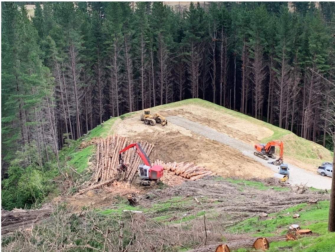
Photo 10: Landing 45 - Log 16 working Setting 502 and Tahurua Earthmovers working on truck loadout area.
