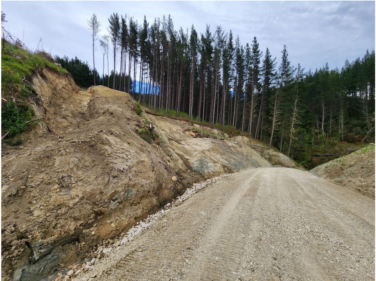
Photo 1: Work completed to prevent road failure at Marker 3 on Murray Road, Setting 500.
