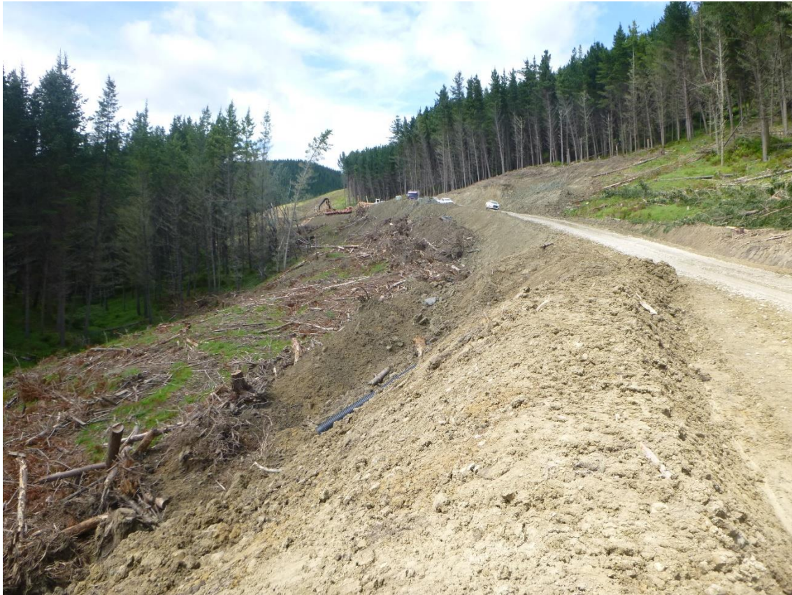
Photo 17: Tahurua Earthmovers recently metalled Mad Mutt Road between Landings 4 and 7 with some water controls yet to be completed.
