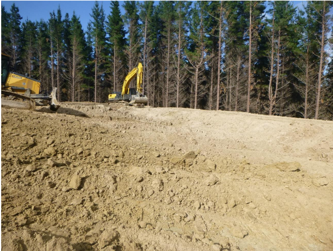
Photo 13: Tahurua Earthmovers forming Landing 41 at the end of Thomson Road.
