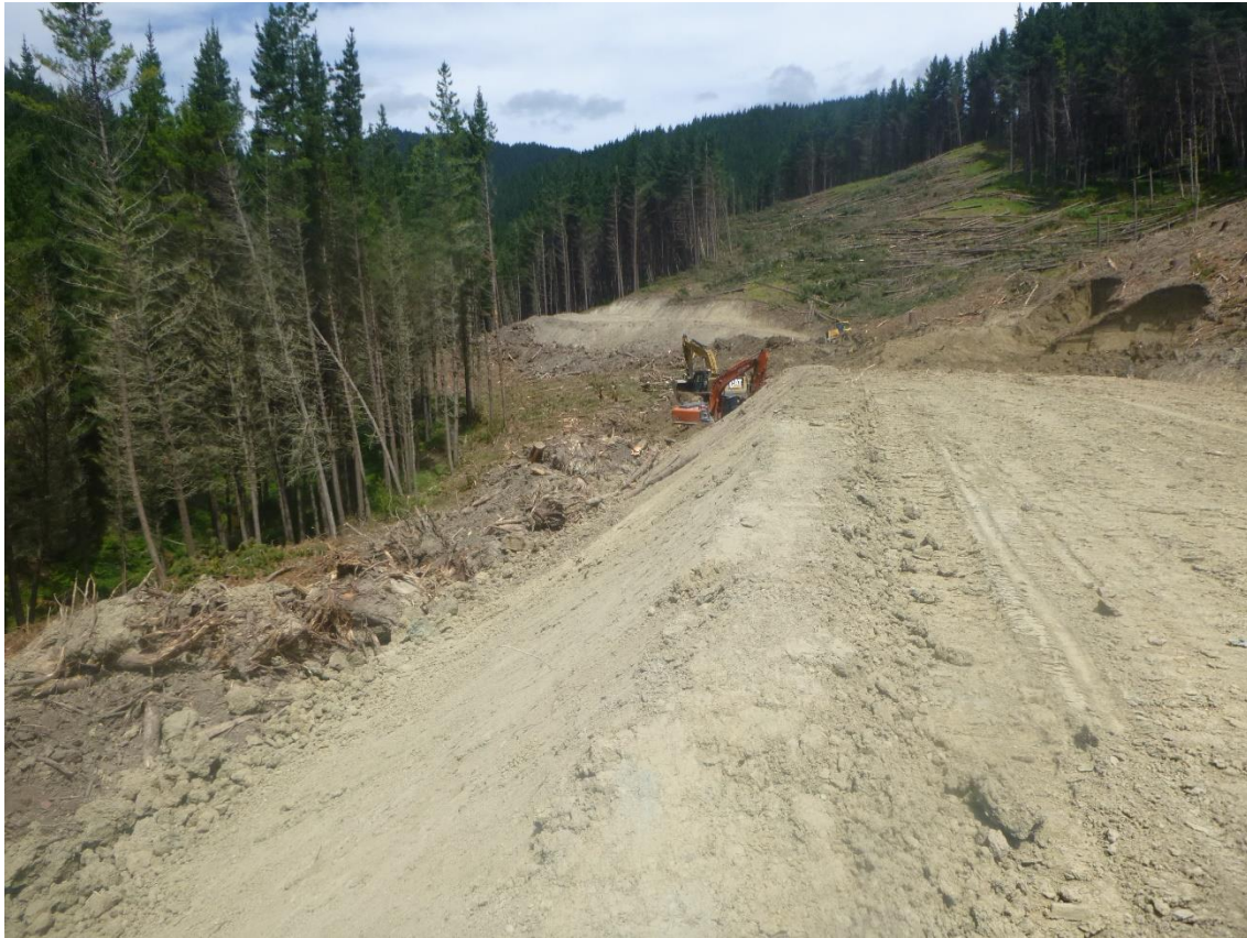
Photo 11: Tahurua Earthmovers formed Landing 7 and beginning the road to Landing 39.
