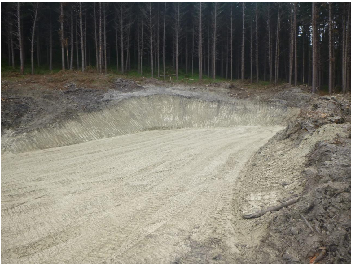
Photo 10: Tahurua Earthmovers recently formed Landing 6.
