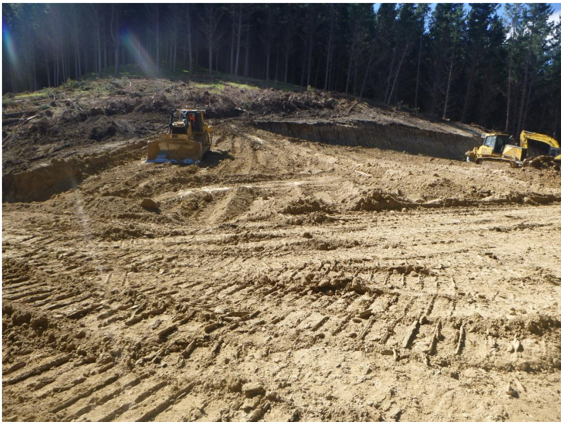
Photo 14: Tahurua Earthmovers forming Landing 41 at the end of Thomson Road.
