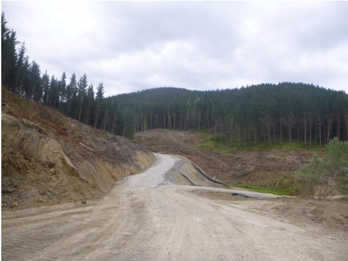
Photo 9: Tahurua Earthmovers recently metalled road to Landing 6, with early stages of construction of Mad Mutt Road in background.
