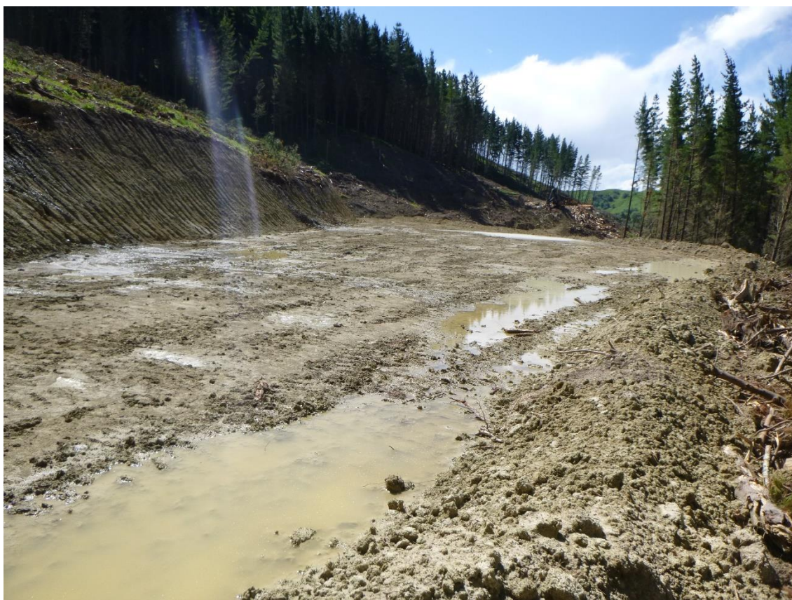
Photo 16: Tahurua Earthmovers almost completed Landing 39.
