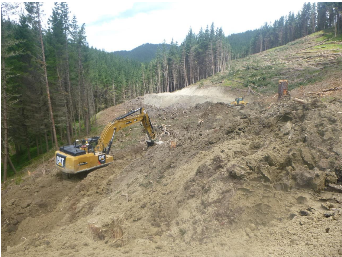
Photo 12: Tahurua Earthmovers forming the road to Landing 39.
