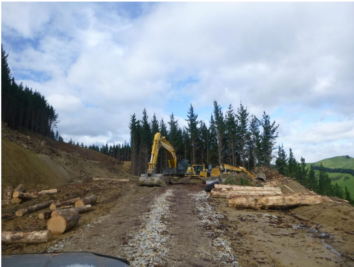
Photo 18: Tahurua Earthmovers beginning the rehab of Landing 106, and formation of switch back on Wood Road.
