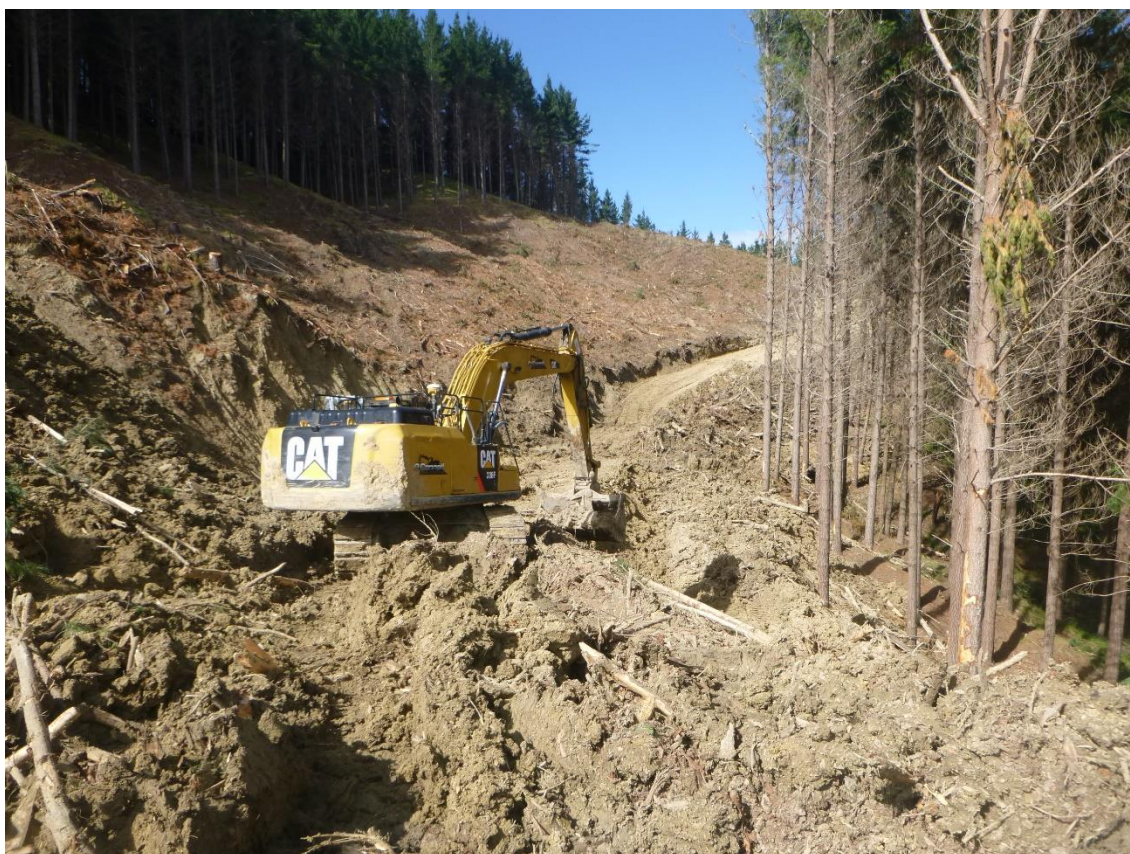
Photo 15: Tahurua Earthmovers beginning forming Thomson Road between Landings 106 and 41.
