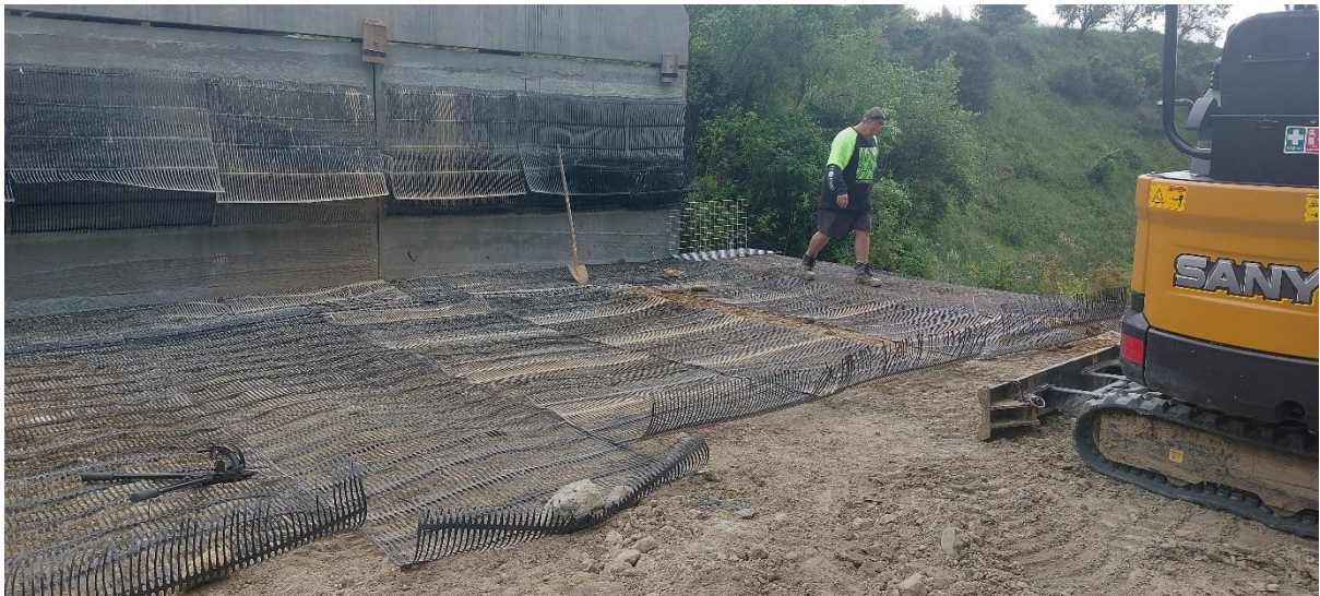
Photos 13 & 14: Installation of Duramesh retaining wall at the Dashwood / Ormsby bridge – George Road.
