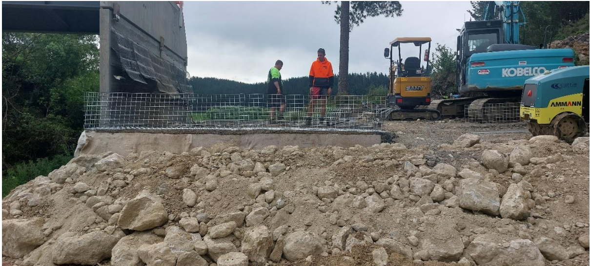
Photos 13 & 14: Installation of Duramesh retaining wall at the Dashwood / Ormsby bridge – George Road.
