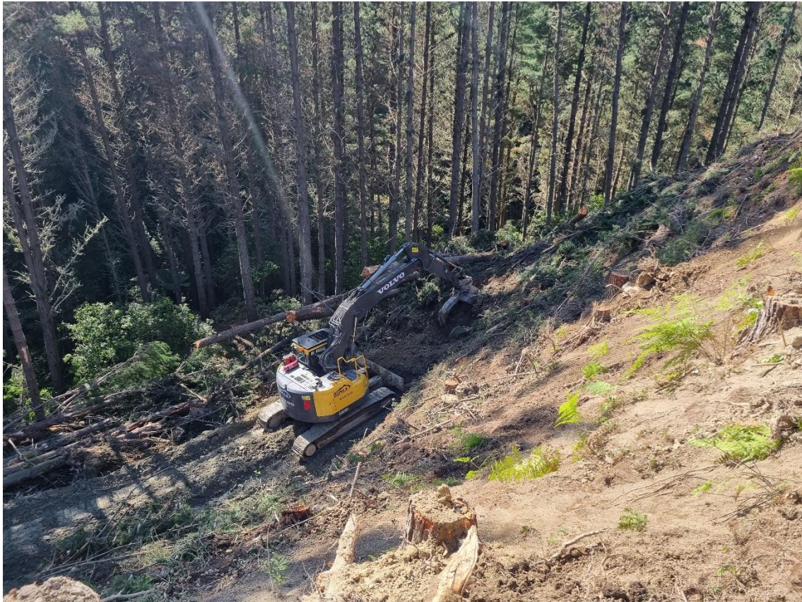
Photo 7: Track work being put in for extraction, doubling up as bench for road formation.
