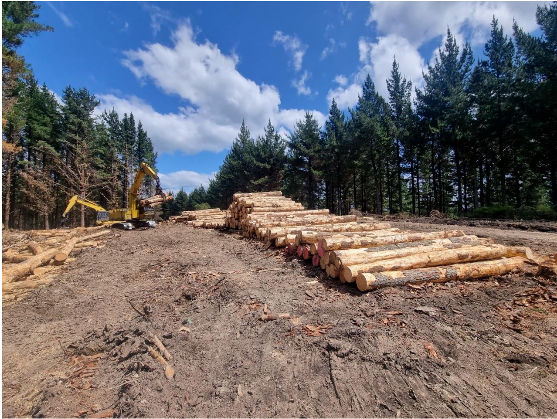
Photo 9: Log stacks being formed on temporary roadlining landing.
