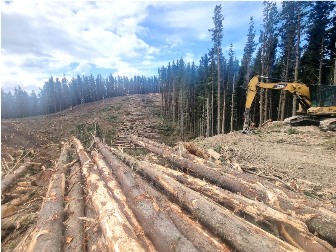
Photo 7: Stacks of stems being stockpiled on Landing 3.
