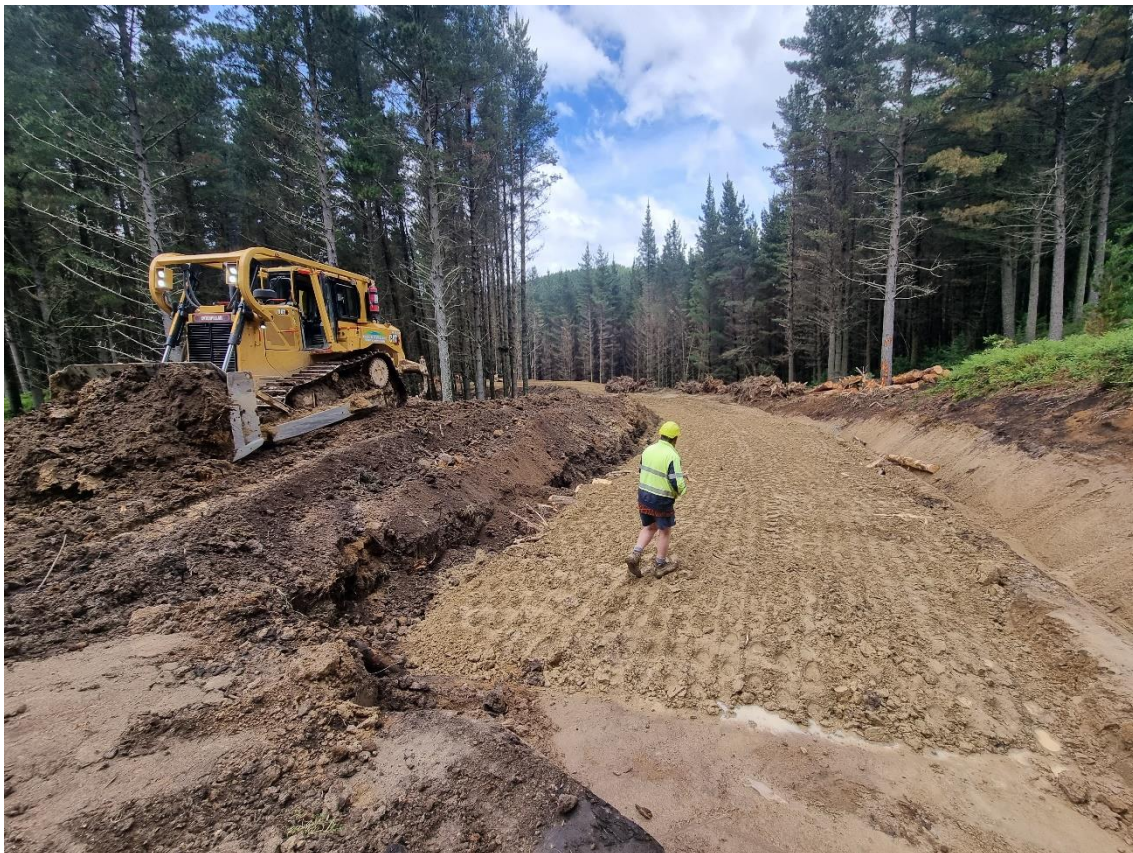
Photo 10: Formation work on road to Landing 9.
