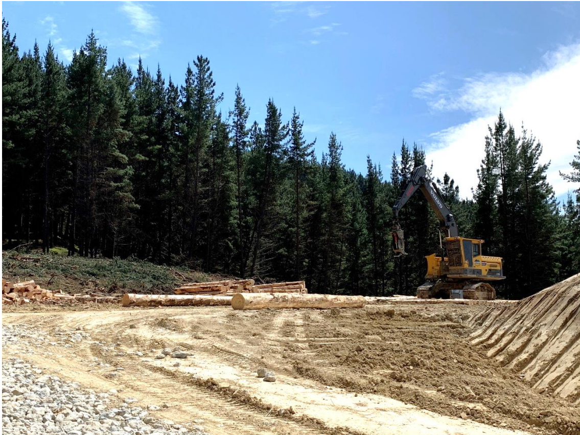
Photo 3: Volvo loader setting up on Landing 9.
