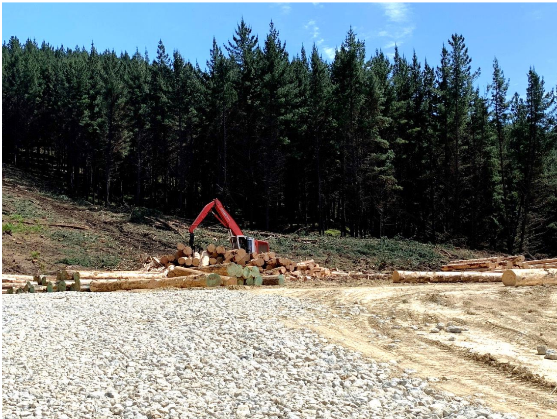
Photo 2: Log 16 Madill 2250C processor working on Landing 9.
