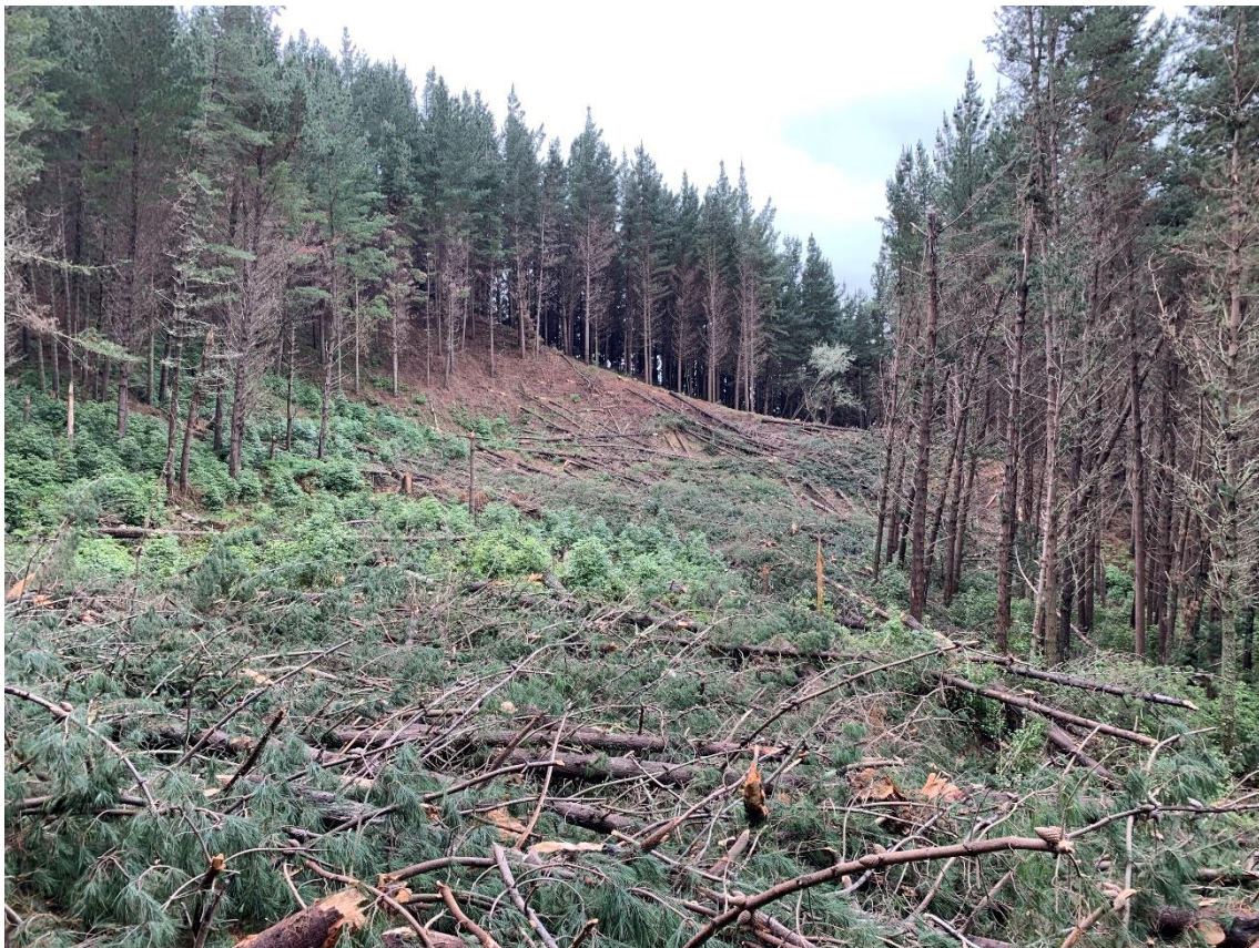
Photo 2: Roadline corridor being felled out towards Landing 28.
