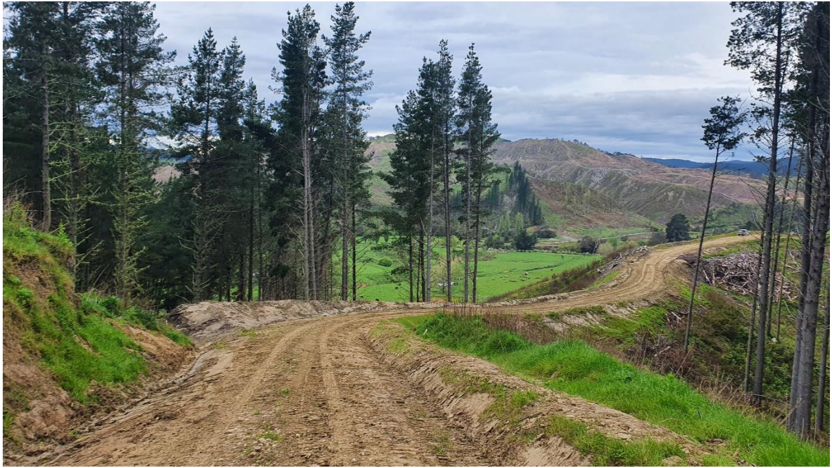
Photo 1: Setting 501 formation being reinstated to Pharm Road for future harvest operations.
