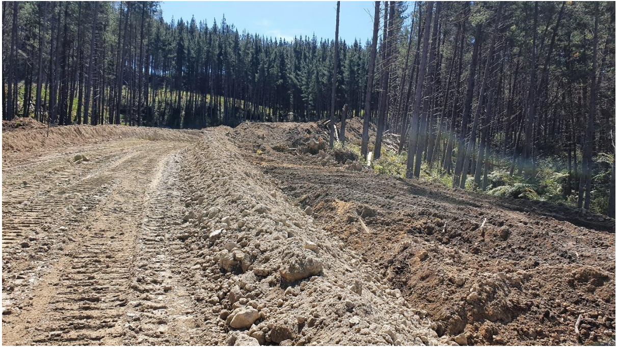
Photo 3: Construction commencing on Davis Road, Setting 502.
