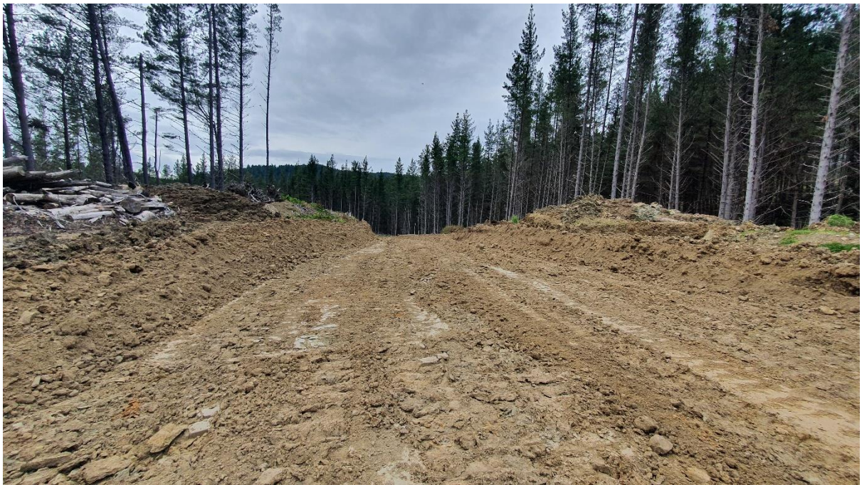
Photo 2: Commencement of construction in Setting 502, Davis Road.
