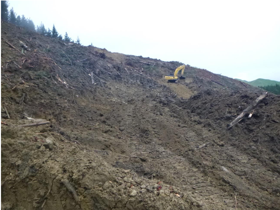
Photo 19: Tahurua Earthmovers beginning benching for the formation of Wood Road from the intersection of Mad Mutt Road and Landing 106.
