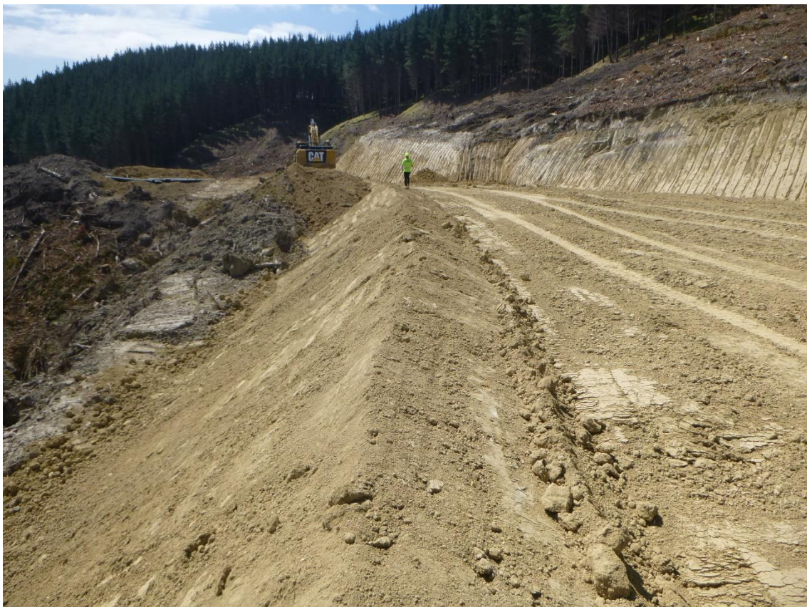
Photo 16: Tahurua Earthmovers linking Landing 106 with Wood Road.
