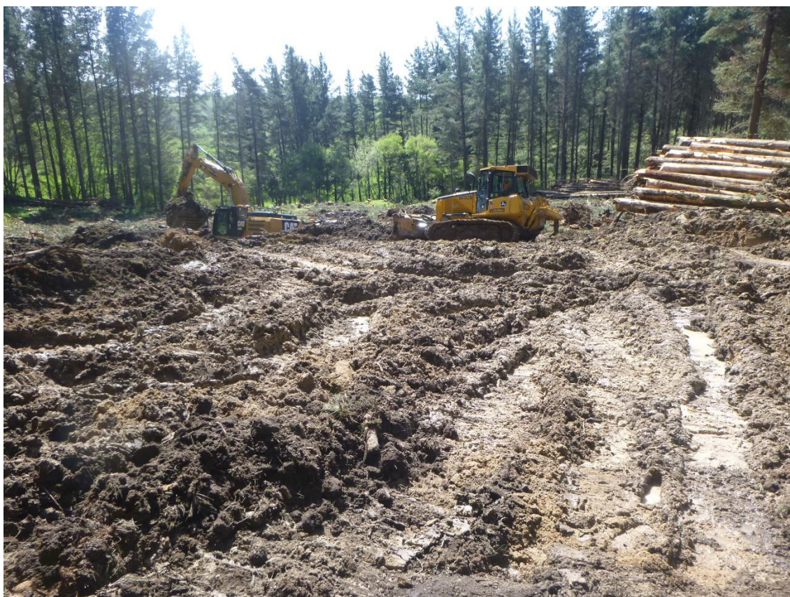
Photo 11: Tahurua Earthmovers forming Landing 4, removing poor soil.
