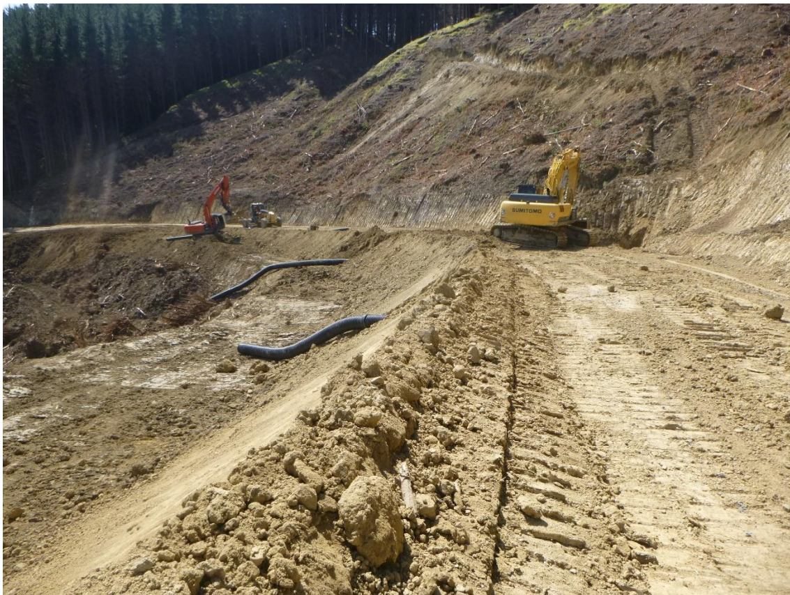
Photo 20: Tahurua Earthmovers forming Wood Road and installing water controls between the intersection of Mad Mutt Road and Landing 106.
