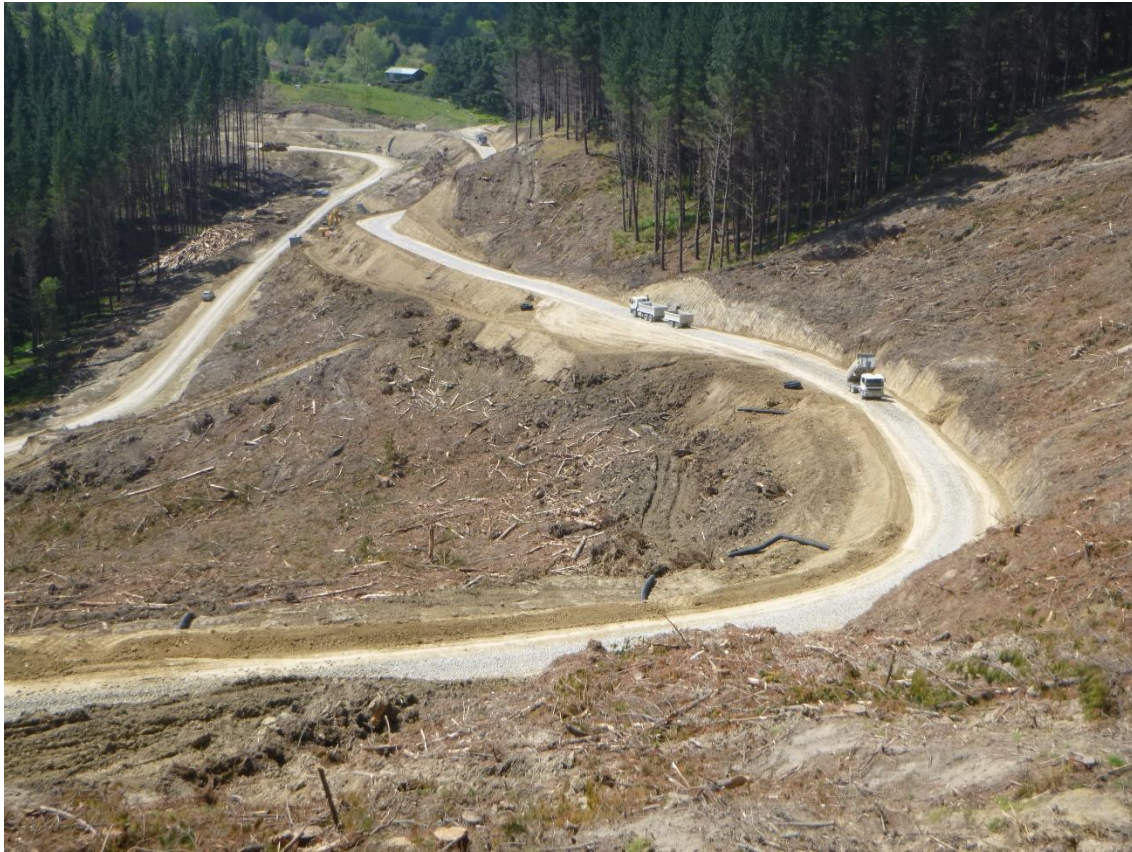
Photo 21: Tahurua Earthmovers metalling Wood Road.
