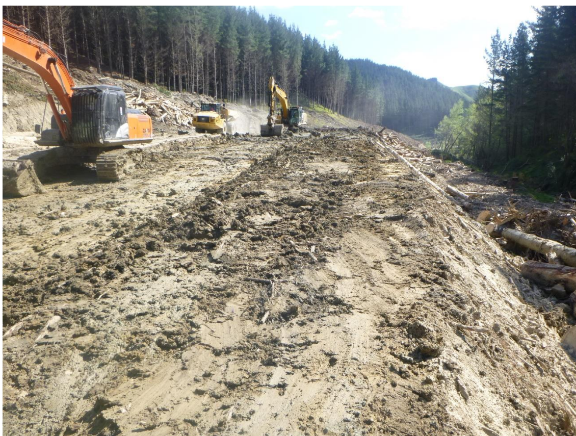
Photo 14: Tahurua Earthmovers rehabilitating Landing 105 and reinstating Mad Mutt Road passing through it.
