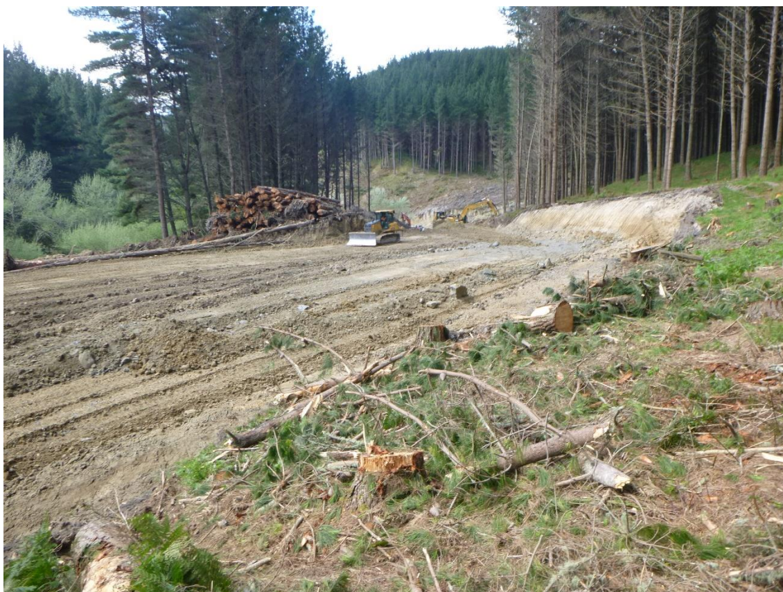
Photo 13: Tahurua Earthmovers forming Landing 4.
