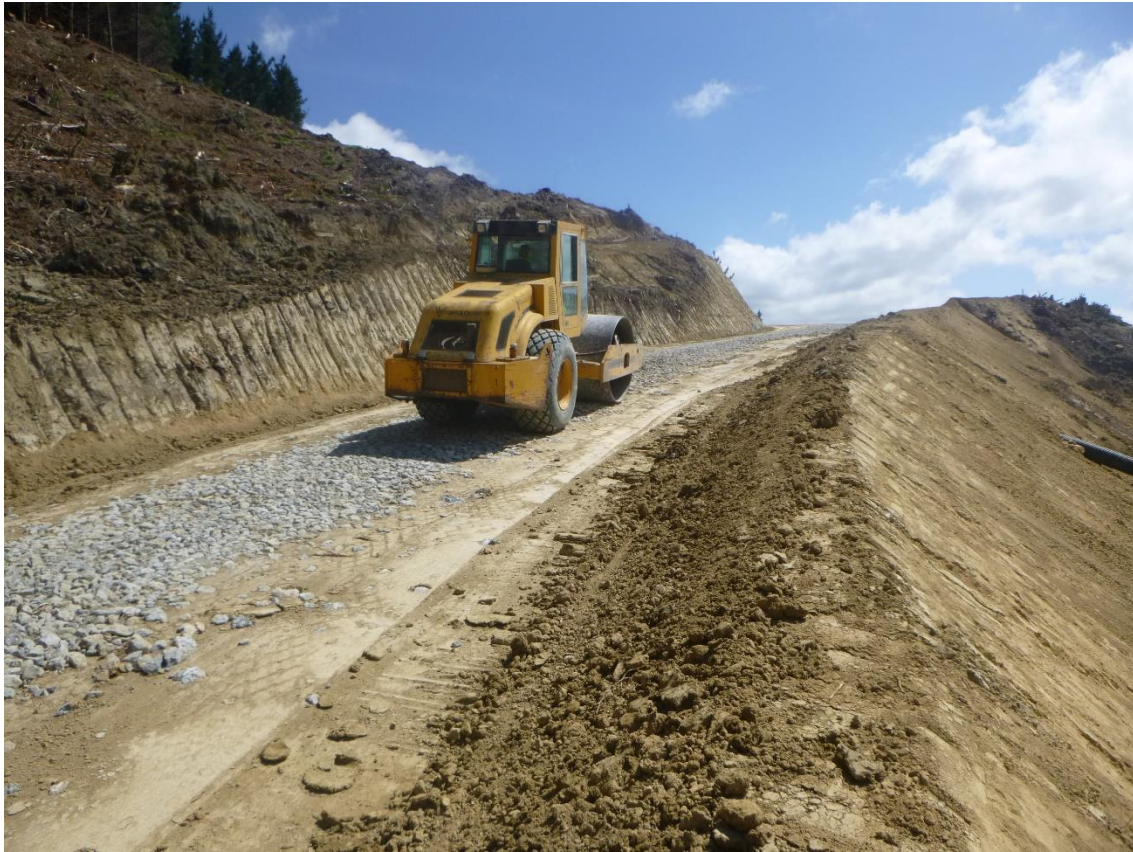
Photo 23: Tahirua Earthmovers rolling Wood Road while metalling.
