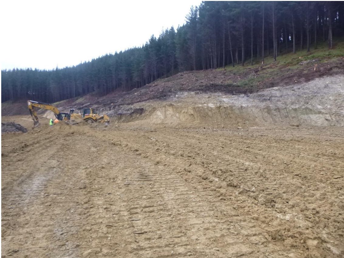
Photo 15: Tahurua Earthmovers completed Landing 106 on Wood Road.
