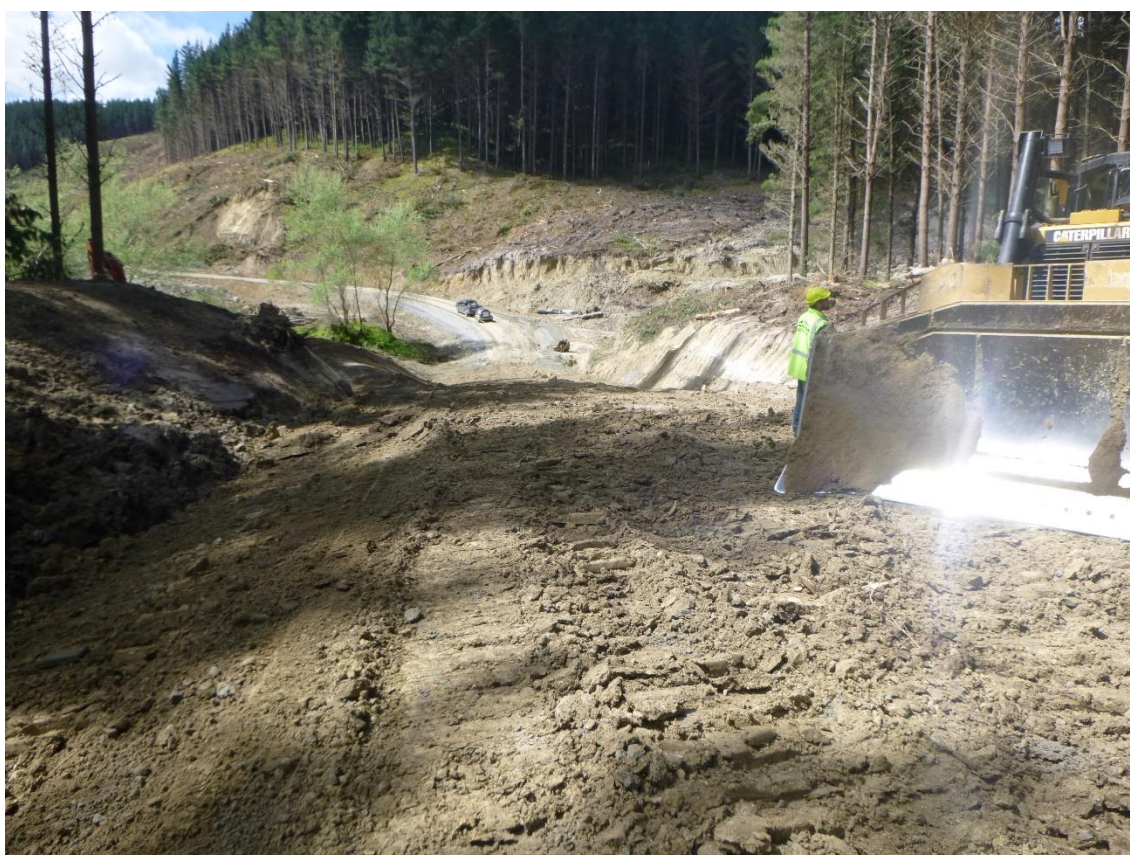
Photo 12: Tahurua Earthmovers forming Landing 4.
