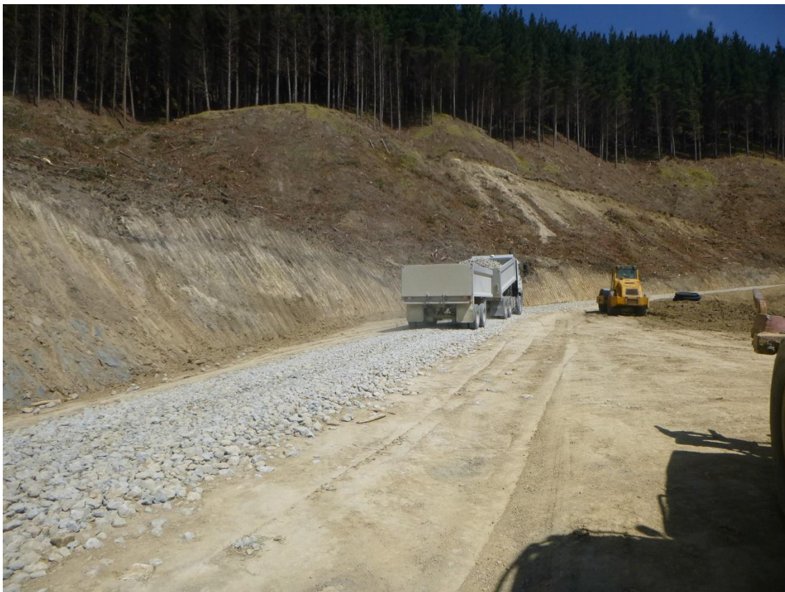
Photo 22: Tahurua Earthmovers metalling Wood Road.
