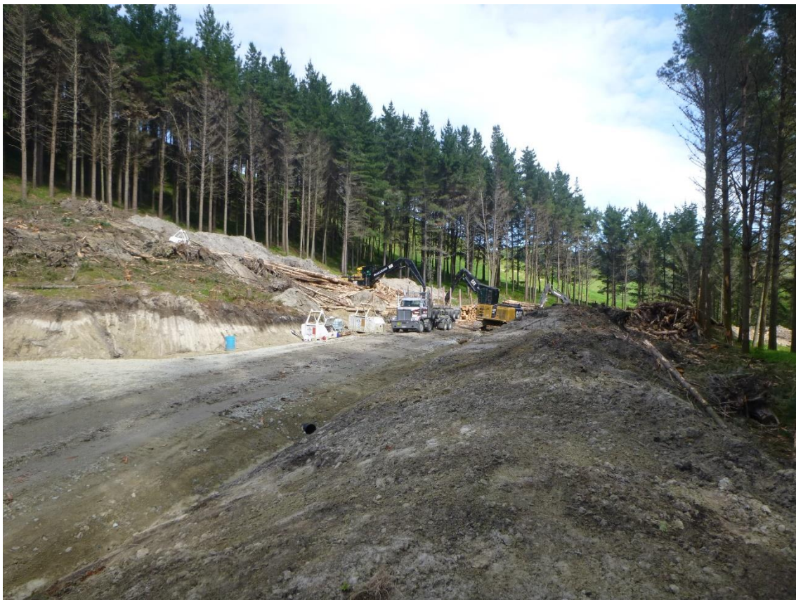
Photo 8: Log 19 loading logs on Landing 4.
