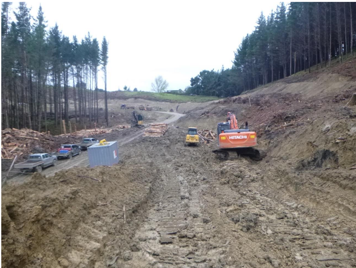
Photo 18: Tahurua Earthmovers constructing Wood Road.
