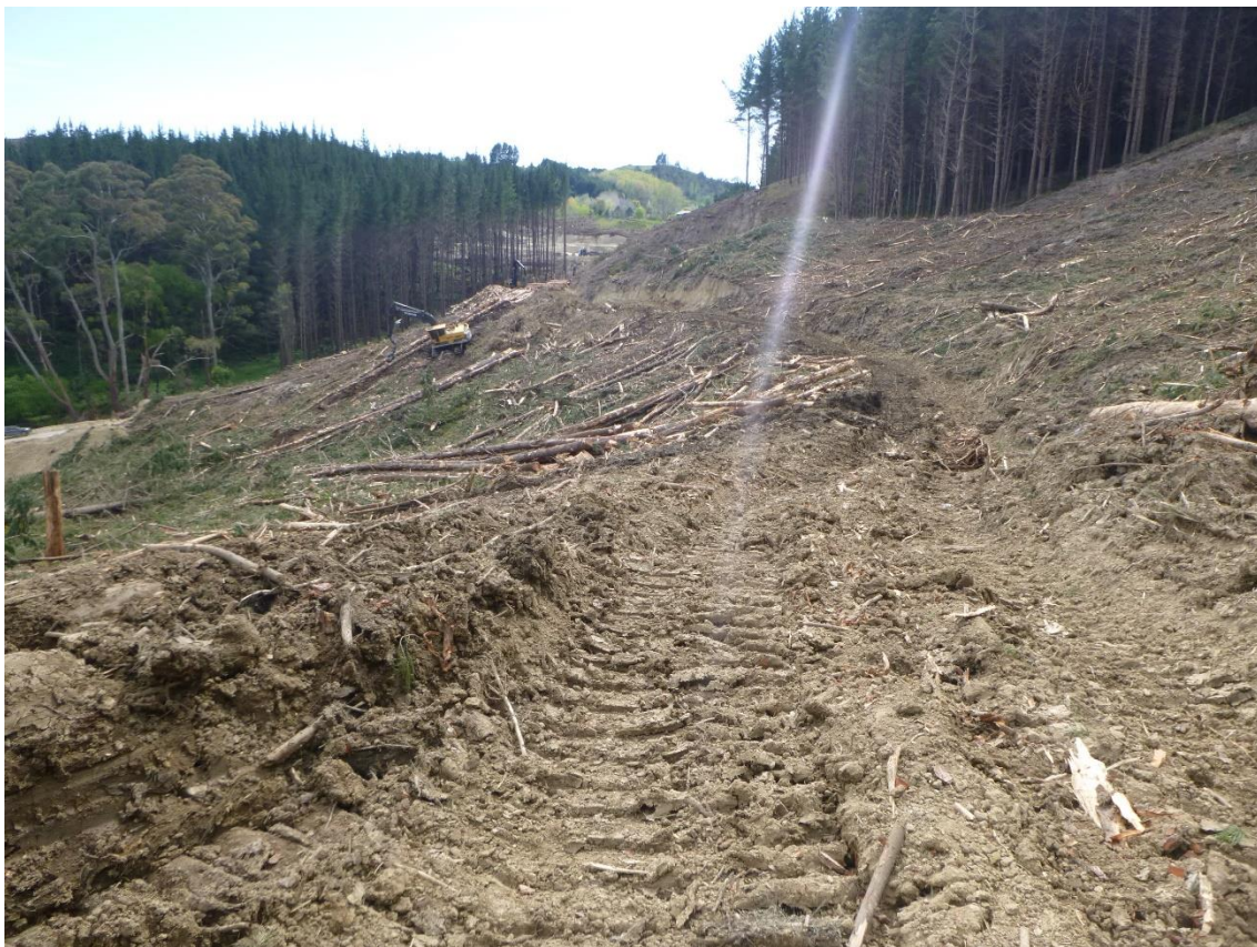
Photo 4: Log 19 extracting stems from Setting 502 to allow the formation of Wood Road.
