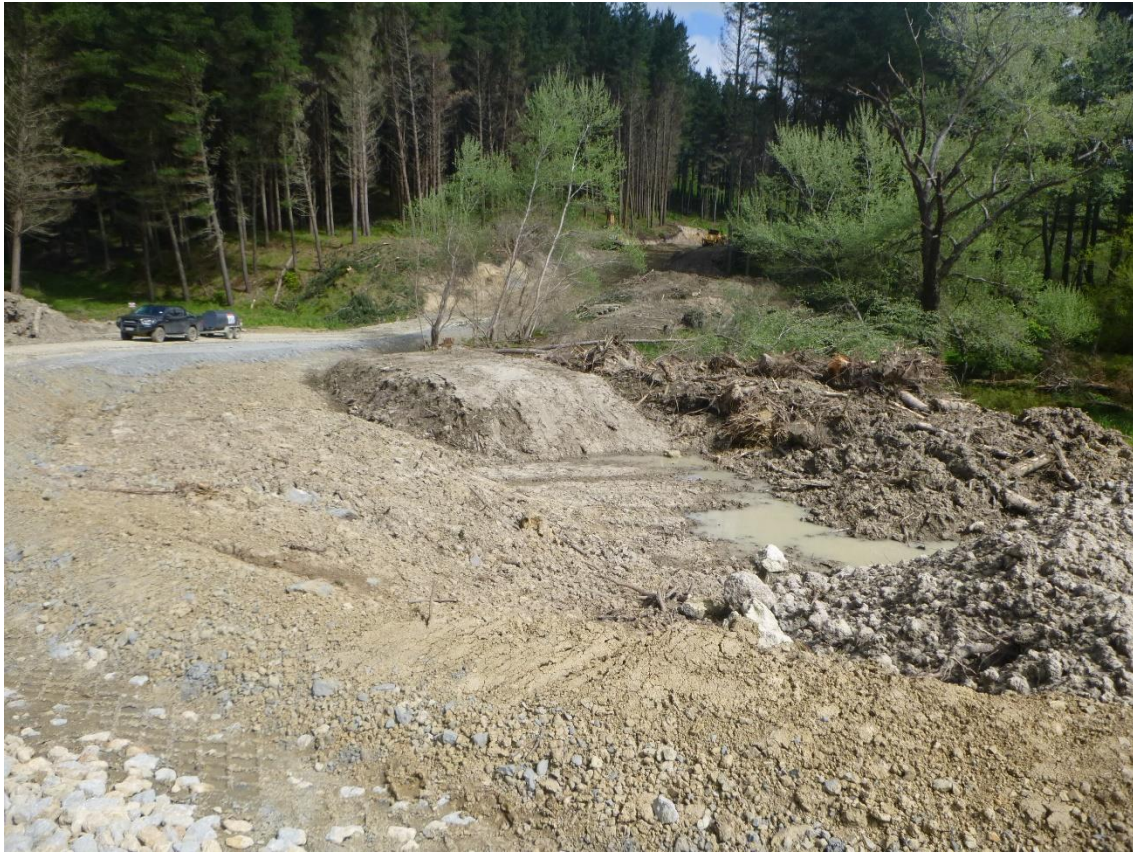
Photo 17: Tahurua Earthmovers stockpiling spoil on the edge of Mad Mutt Road.
