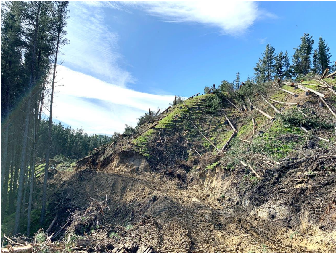
Photo 3: Setting 500 roadline corridor heading out towards Landing 10.
