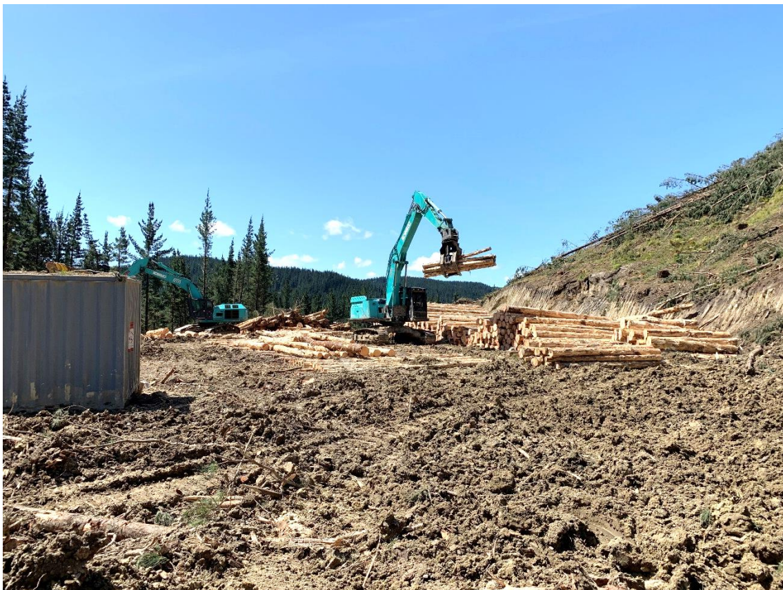
Photo 14: Log 6 Kobelco loader and processor working on Landing 10.
