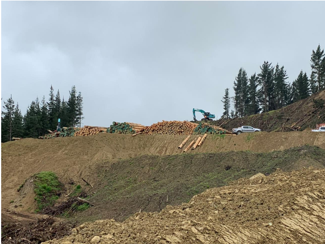
Photo 9: Log 6 working on Landing 5.
