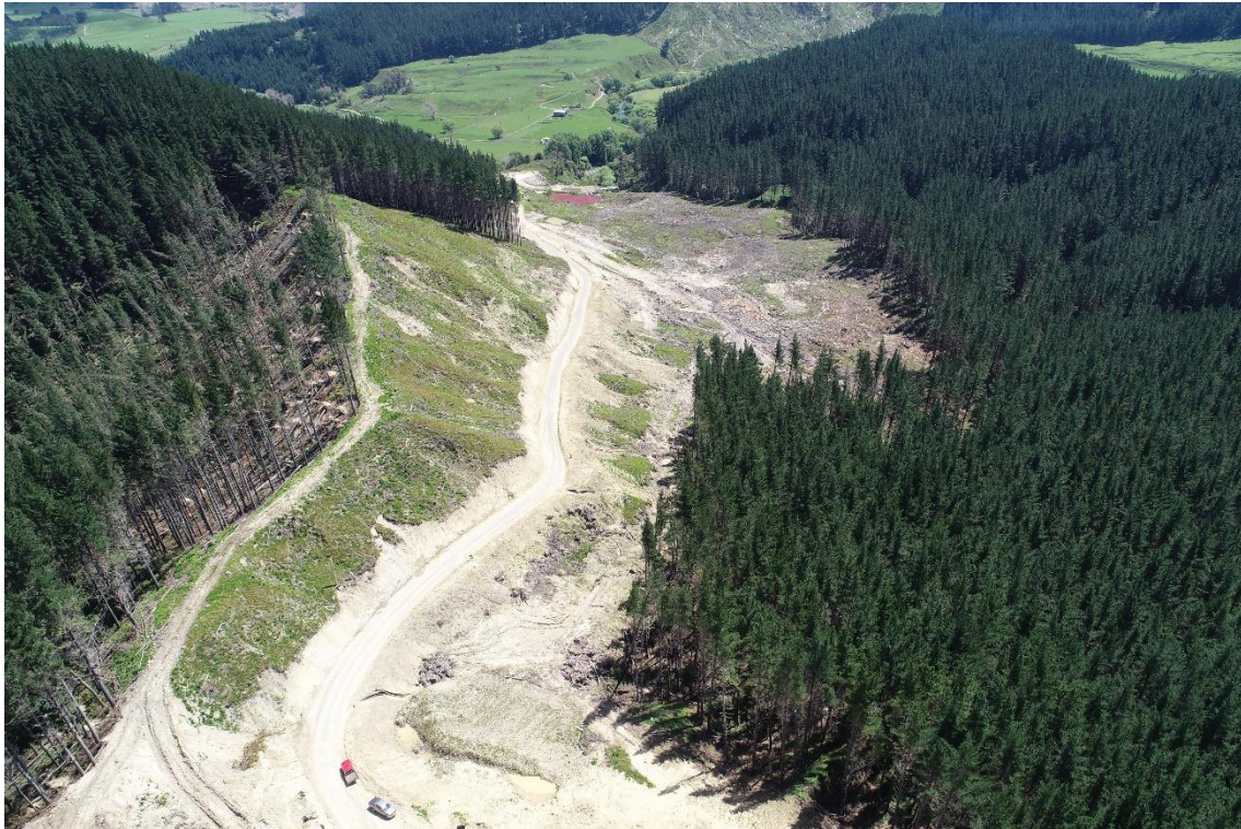
Photo 13: View of Smith Road looking back towards the highway.
