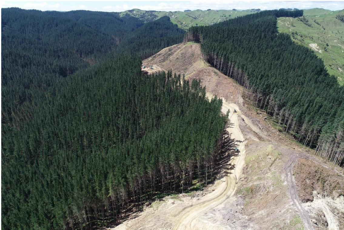
Photo 10: Aerial view of Setting 500 roadline corridor looking from Landing 5 out to landing 10.
