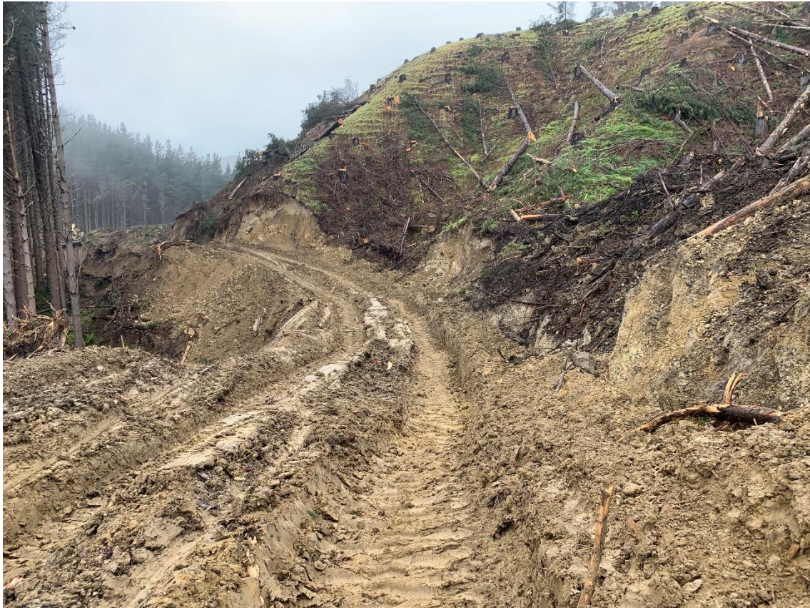
Photo 7: Skidder haul track.
