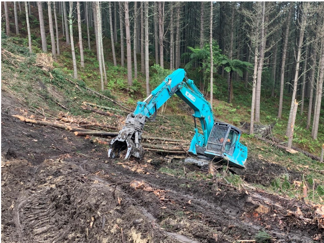
Photo 8: Kobelco shovel loader working in Setting 500 roadline corridor.
