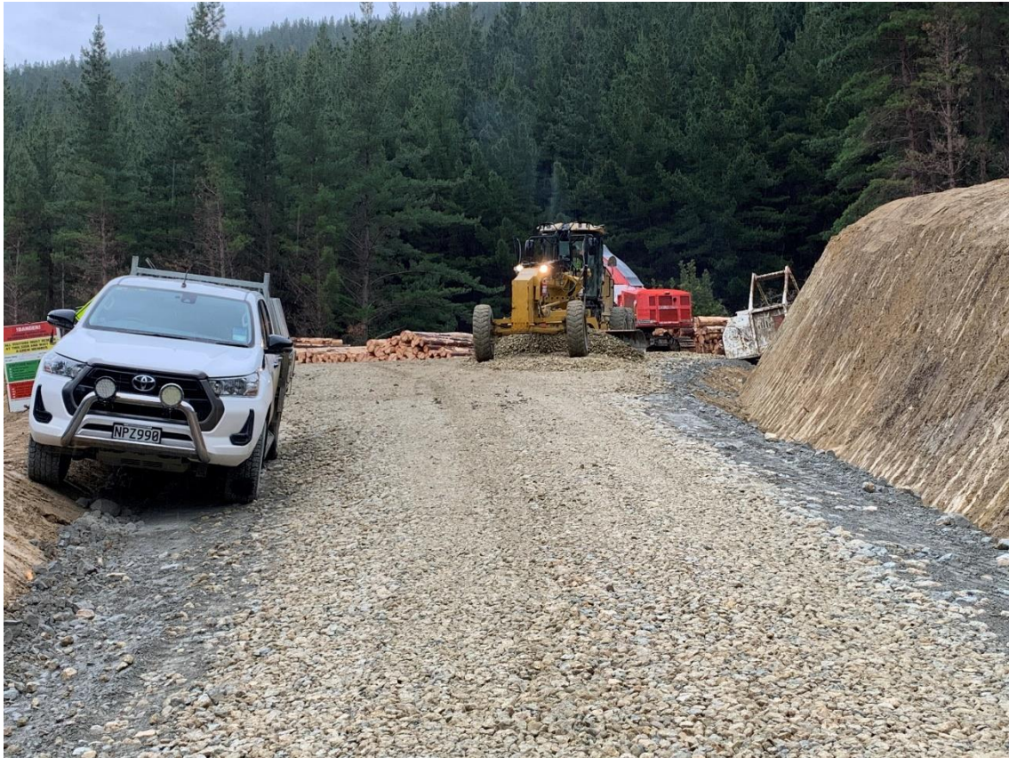
Photo 3: Tahurua Earthmovers grader working on truck turnaround with Madill processor cutting on Landing 7.
