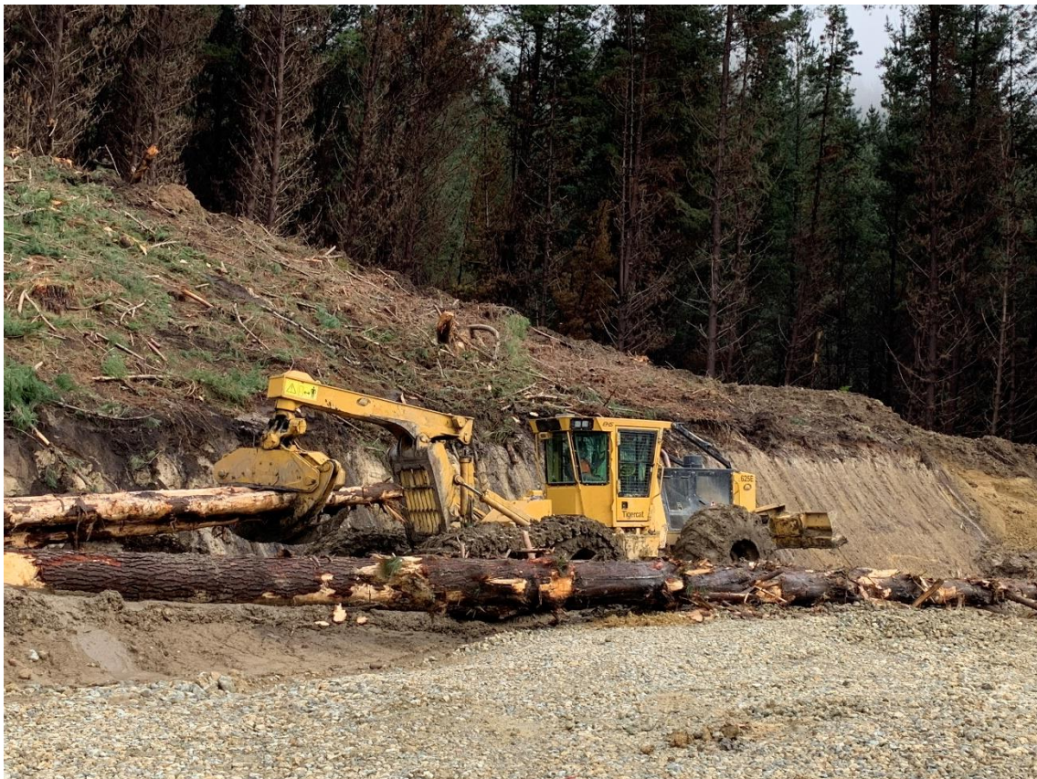
Photo 4: Log 16 625E Tigercat skidder pulling a drag on Landing 8.
