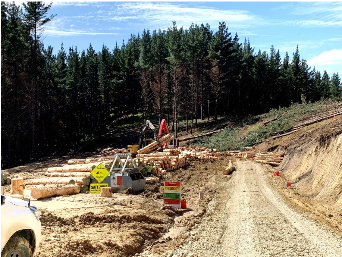
Photo 4: Log 16 working on Landing 55, Long Road.
