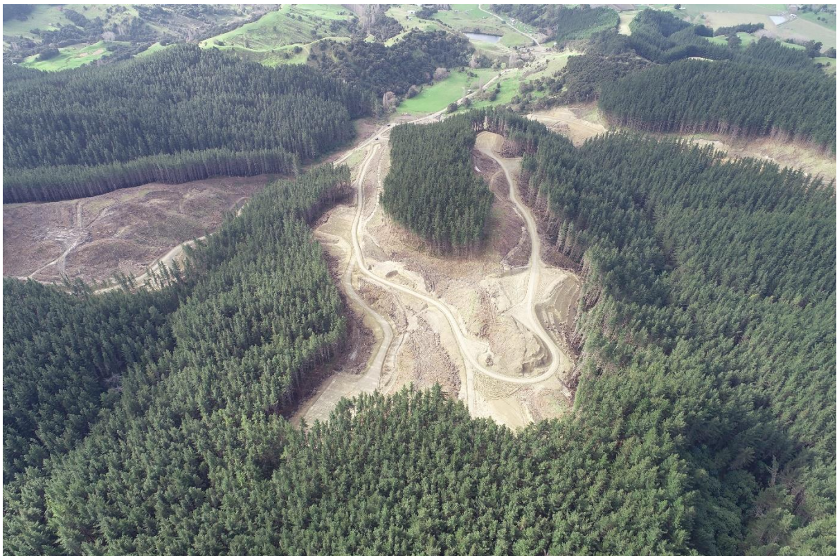
Photo 2: Engineering and harvesting work carried out on Hoko Road with Lee Pee Road to the right of the photo.
