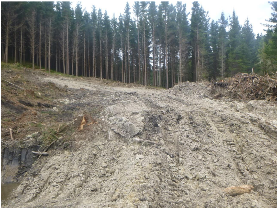
Photo 22: Tahurua Earthmovers stripping off slash in the construction of Landing 6.
