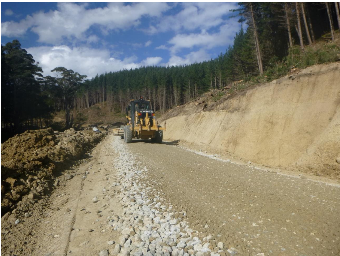
Photo 12: Tahurua Earthmovers grading Mad Mutt Road between Landings 3 and 105.
