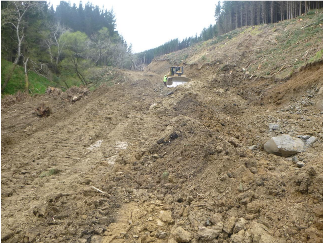
Photo 15: Tahurua Earthmovers forming Mad Mutt Road between Landings 105 and 4.
