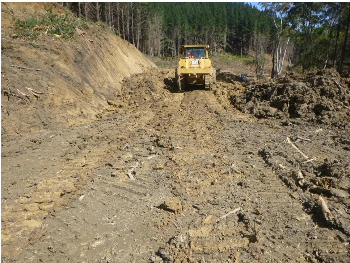
Photo 8: Tahurua Earthmovers constructing Mad Mutt Road between Landings 3 and 105.
