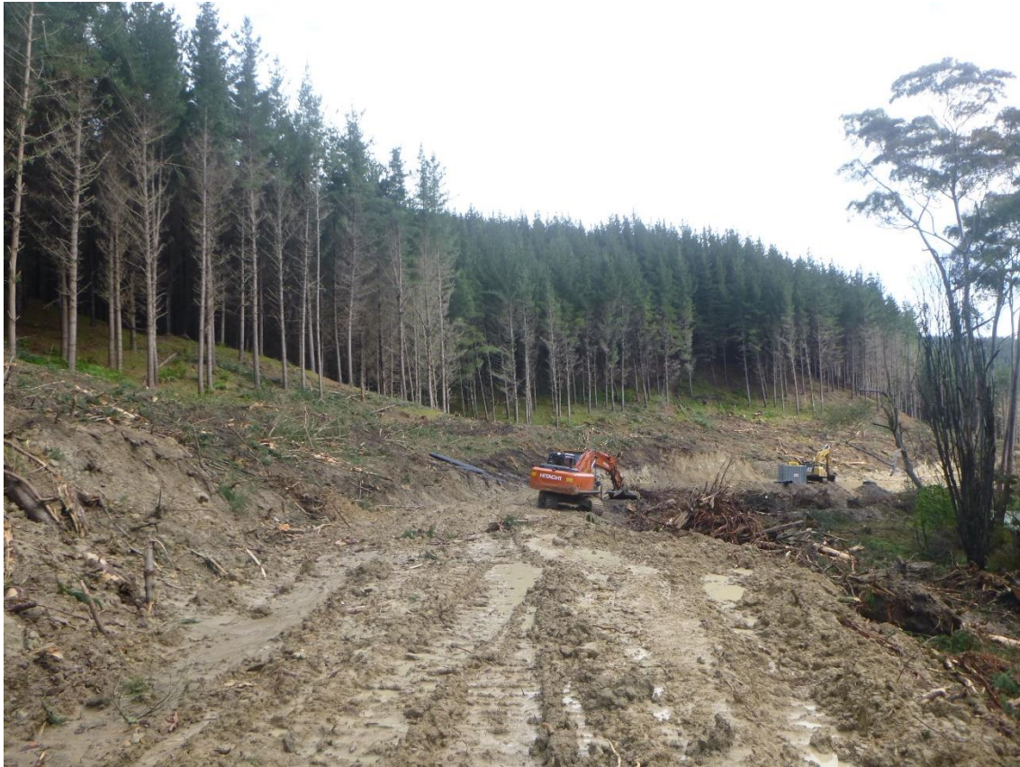
Photo 7: Tahurua Earthmovers constructing Mad Mutt Road between Landings 3 and 105.
