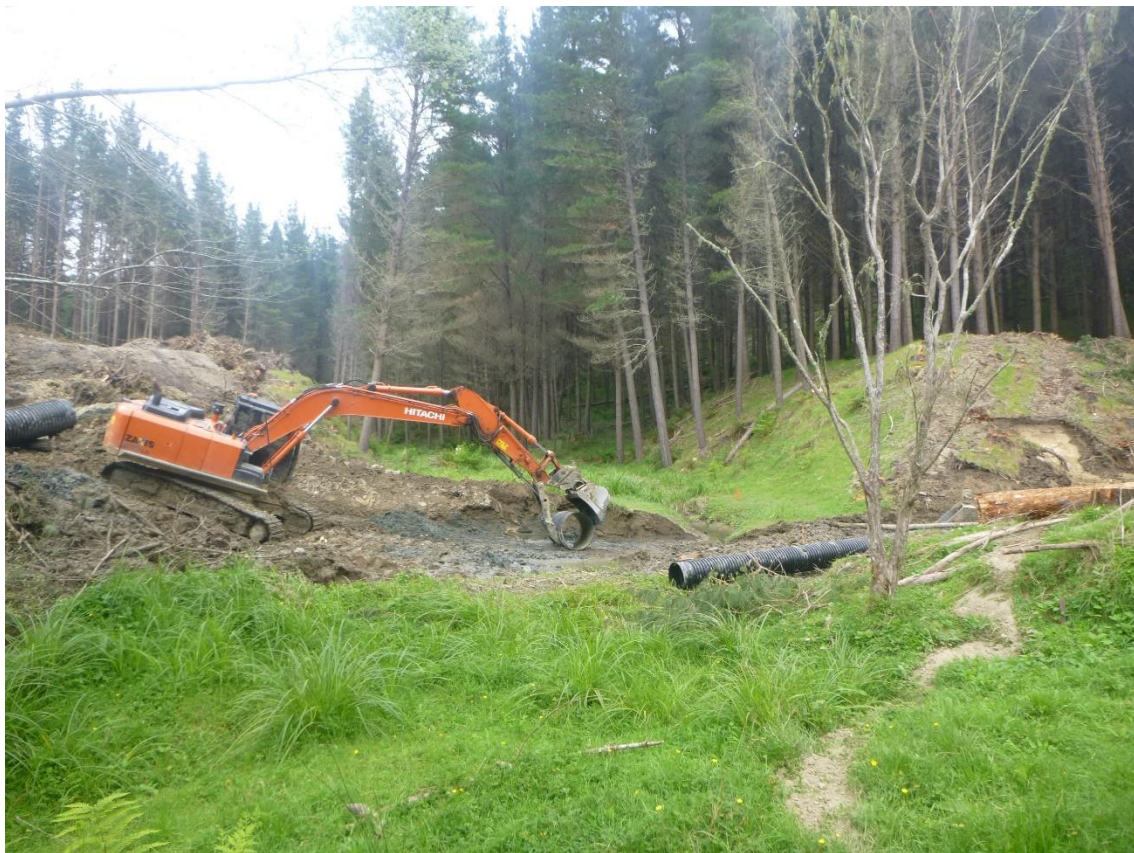
Photo 20: Tahurua Earthmovers constructing a temporary crossing on Mad Mutt Road near Landing 4.
