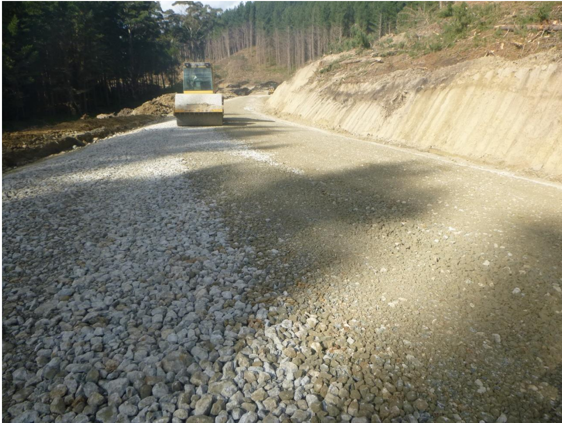
Photo 13: Tahurua Earthmovers rolling Mad Mutt Road between Landings 3 and 105.
