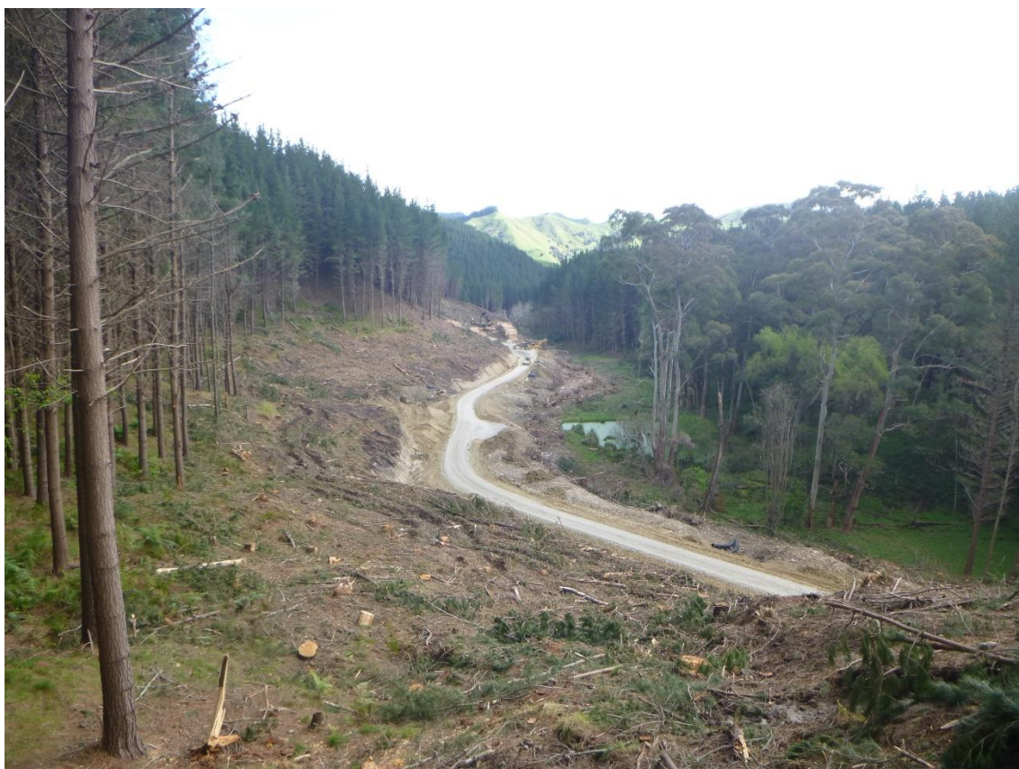
Photo 23: Tahurua Earthmovers completed section of Mad Mutt Road between Landing 3 and 105.
