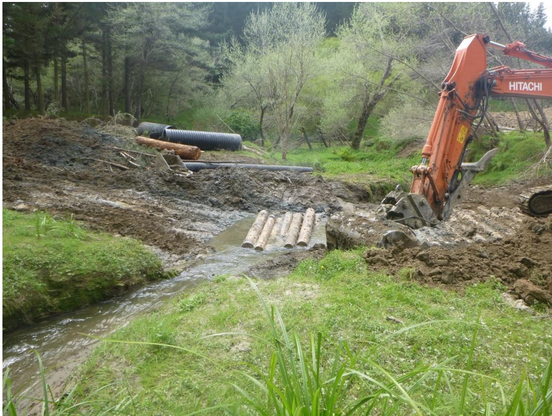
Photo 19: Tahurua Earthmovers constructing a temporary crossing on Mad Mutt Road near Landing 4.
