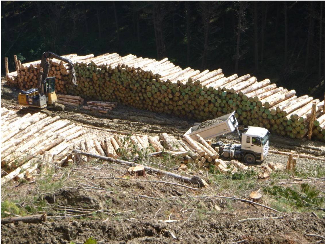
Photo 11: Tahurua Earthmovers metalling Mad Mutt Road through Landing 105.
