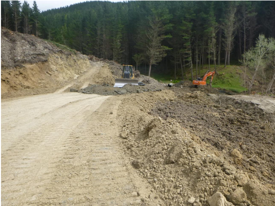
Photo 17: Tahurua Earthmovers forming Mad Mutt Road – pushing out borrow pit material with the bulldozer between Landings 105 and 4.
