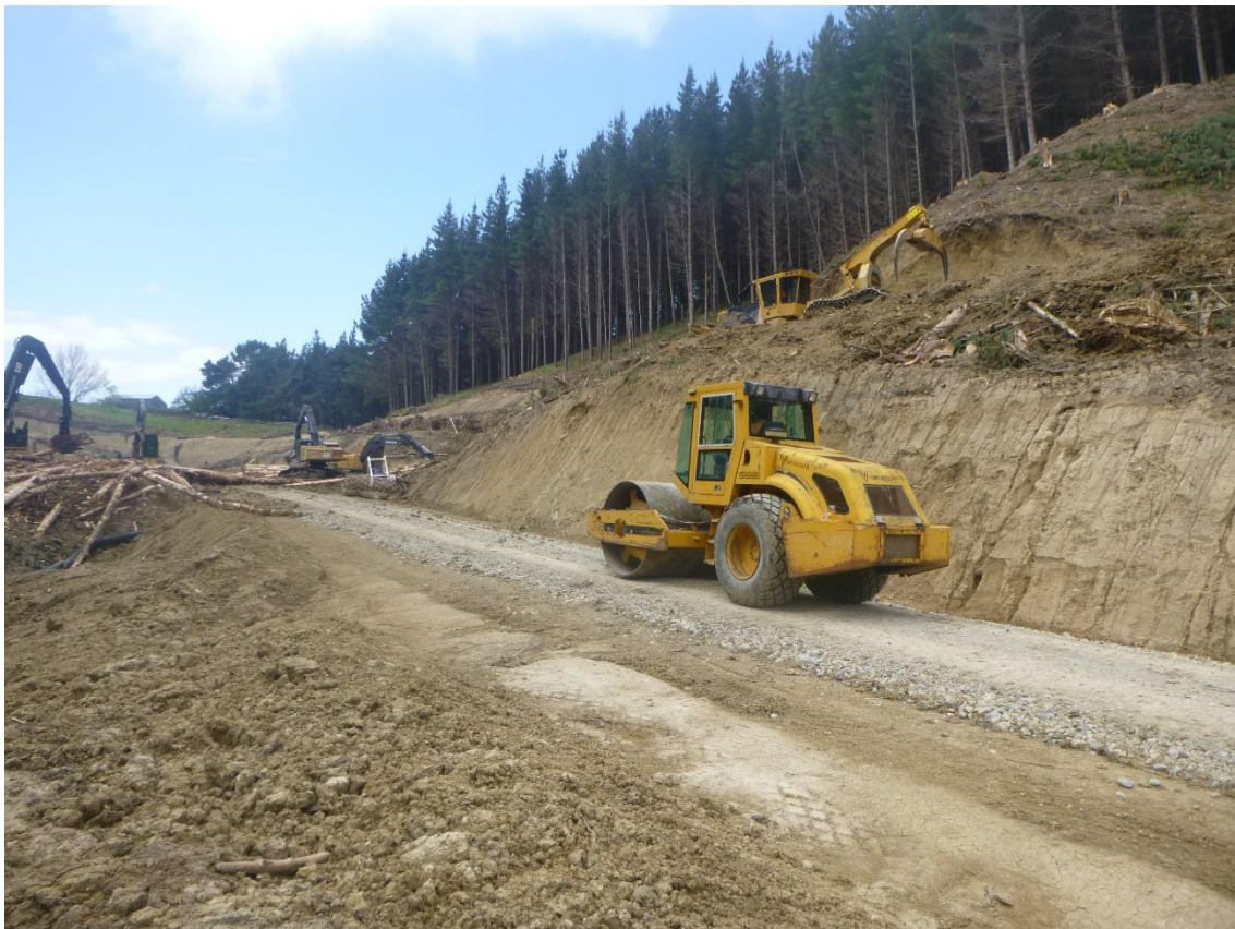
Photo 18: Tahurua Earthmovers rolling Mad Mutt Road near Landing 3.
