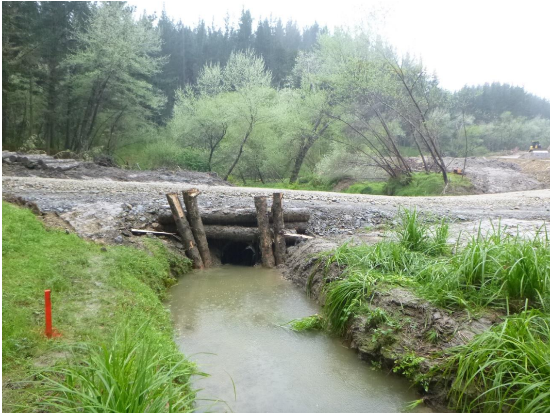
Photo 21: Tahurua Earthmovers completed temporary crossing on Mad Mutt Road near Landing 4.
