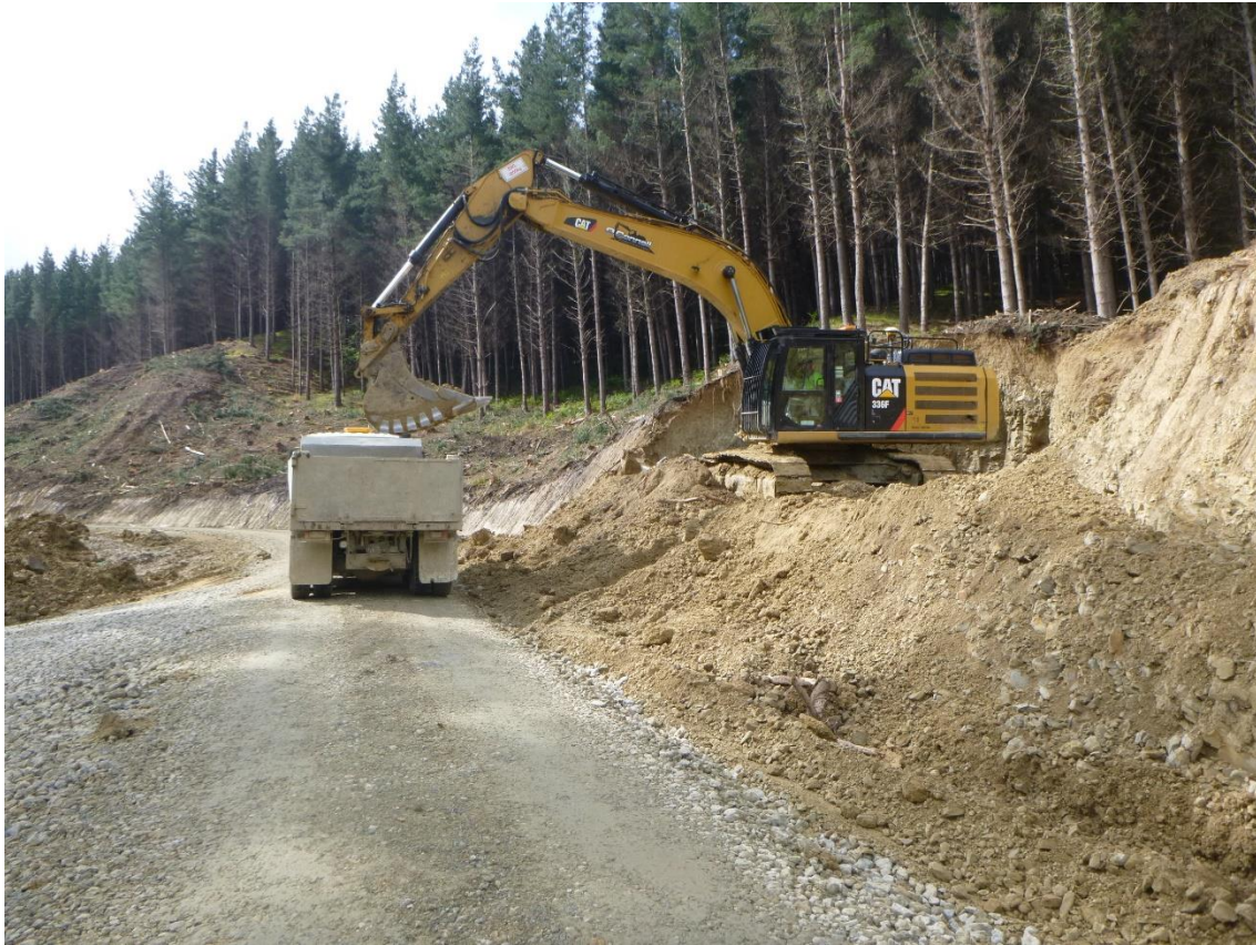
Photo 9: Tahurua Earthmovers constructing Mad Mutt Road between Landings 3 and 105, using borrow pit material to “rock the road”.
