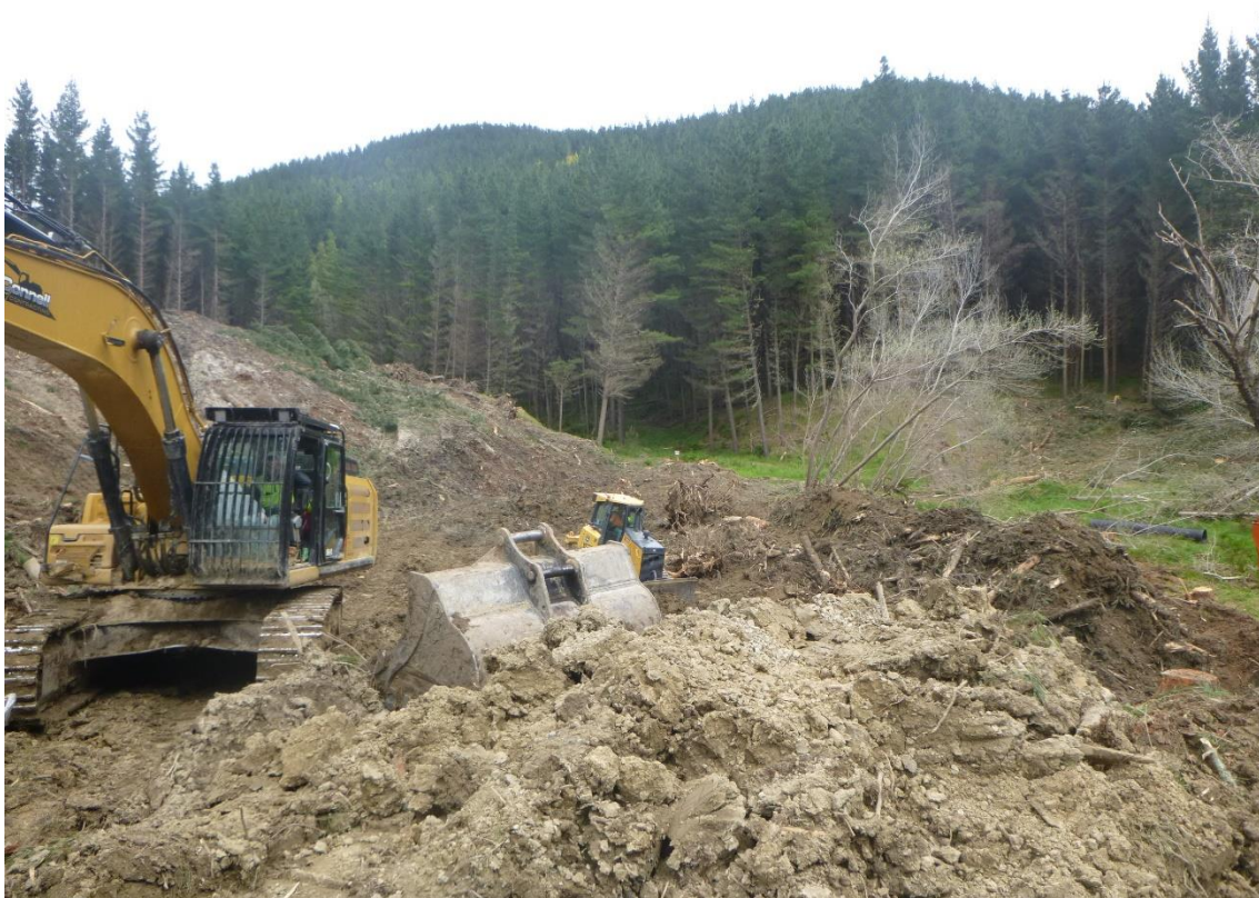
Photo 14: Tahurua Earthmovers forming Mad Mutt Road between Landings 105 and 4.
