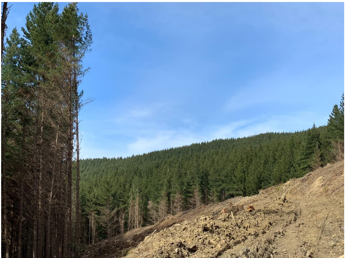
Photo 2: Setting 500 roadline corridor out to Landing 7.
