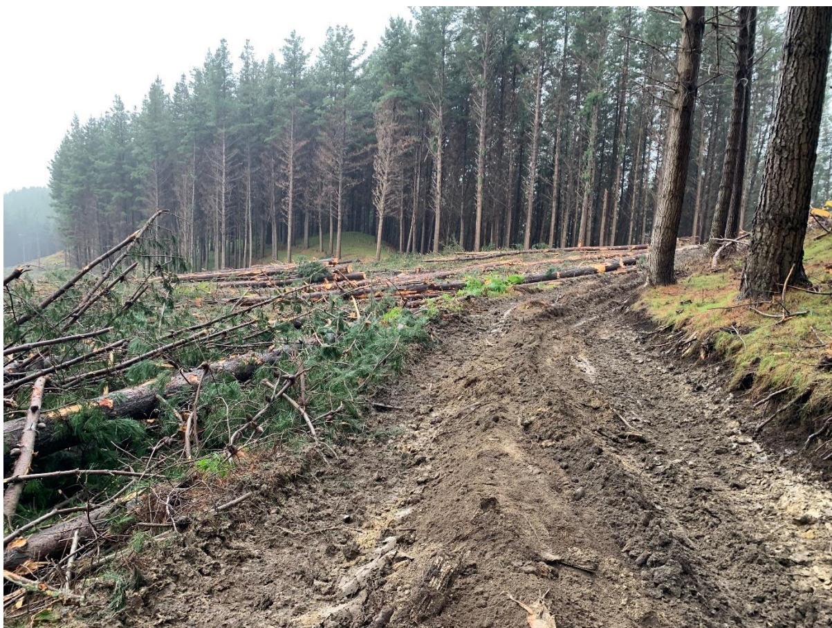
Photo 8: Setting 503 haul track.
