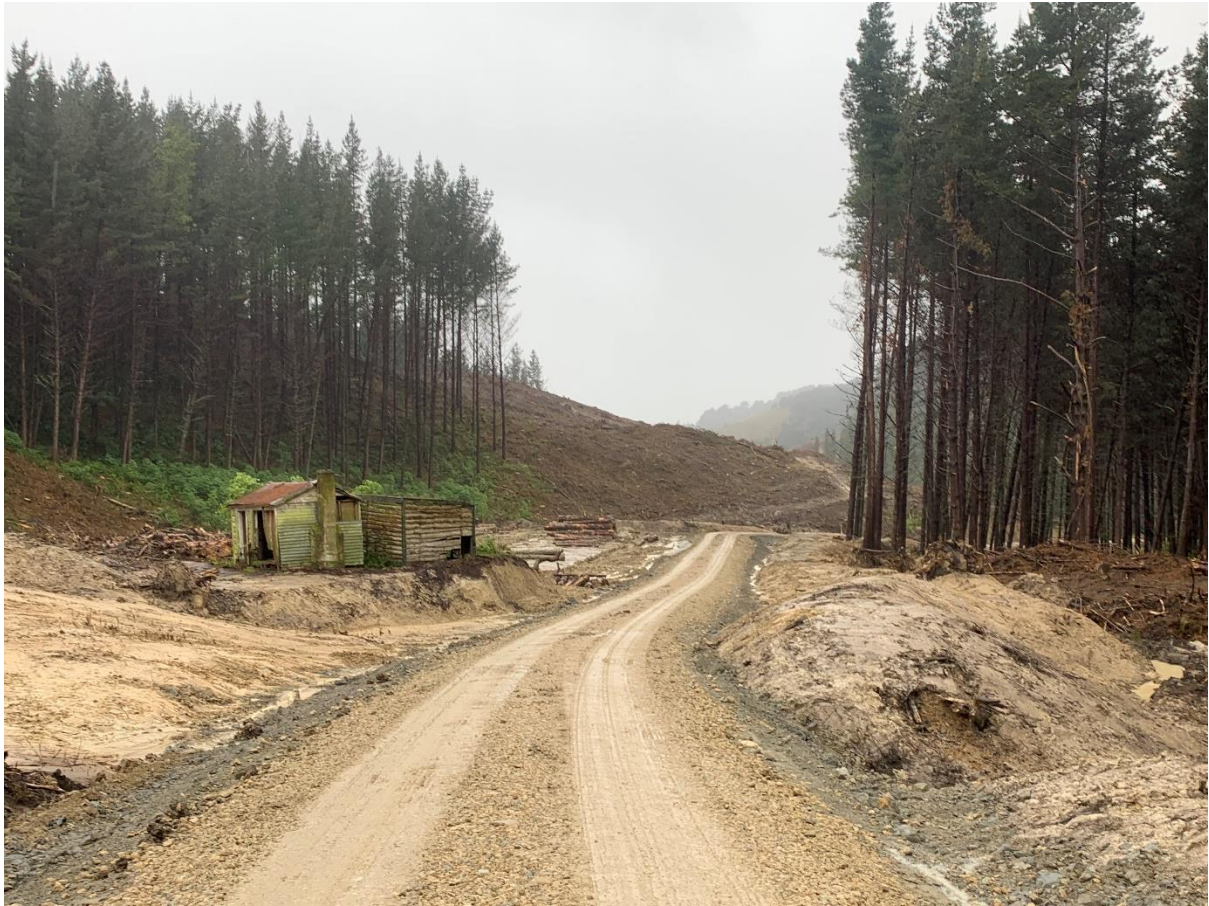
Photo 11: Clarke Road with hut and shed left standing.
