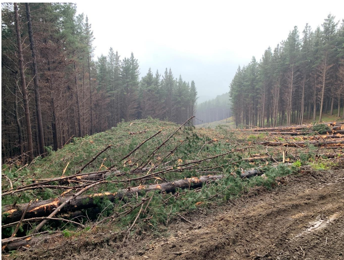
Photo 7: Setting 507 roadline corridor.
