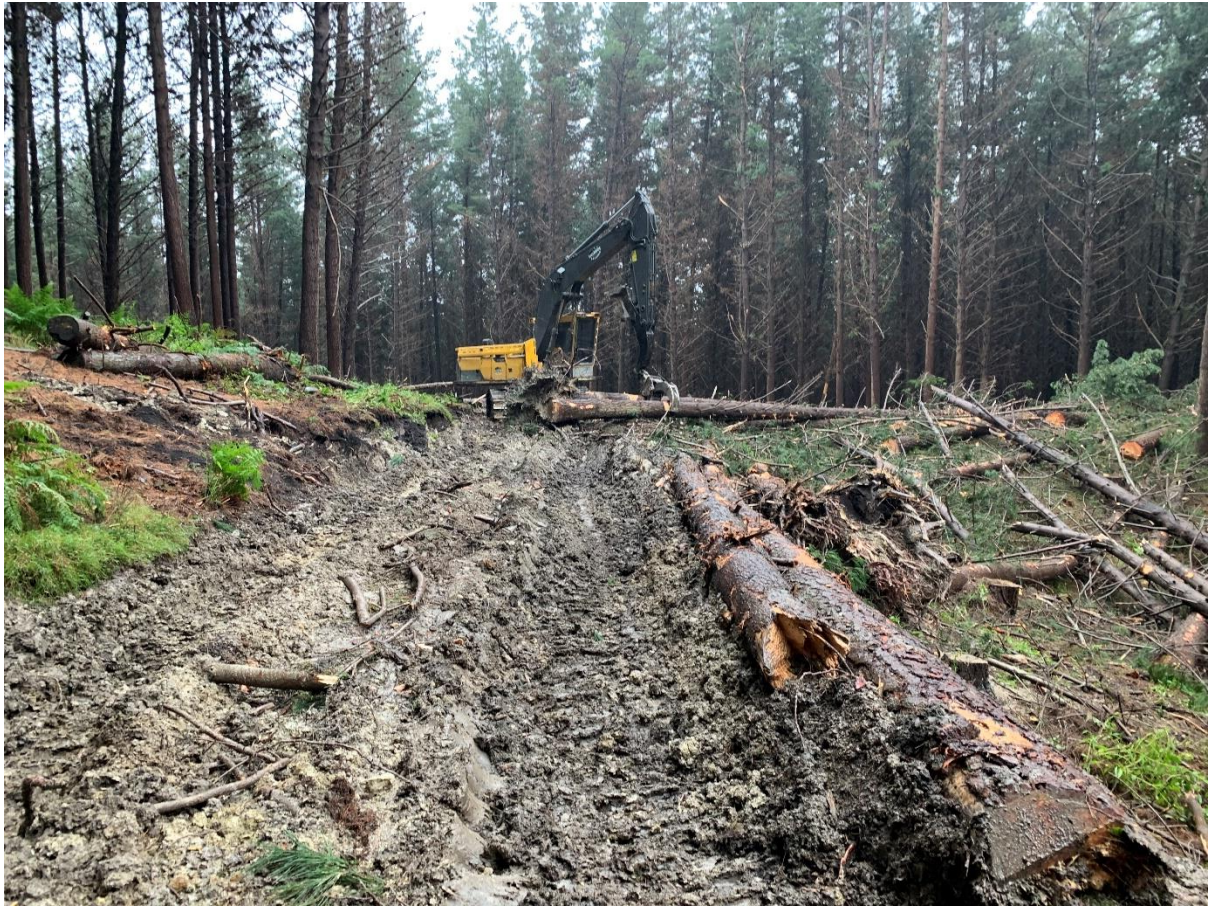
Photo 9: Volvo 300 shovelling on Setting 503 roadline corridor.
