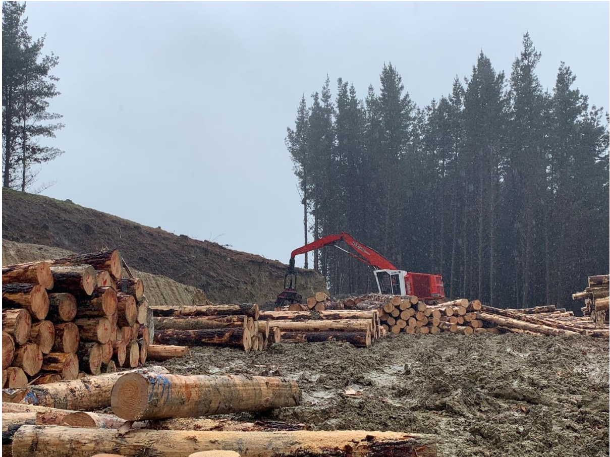
Photo 5: Madill 2250C processor working on Landing 25.
