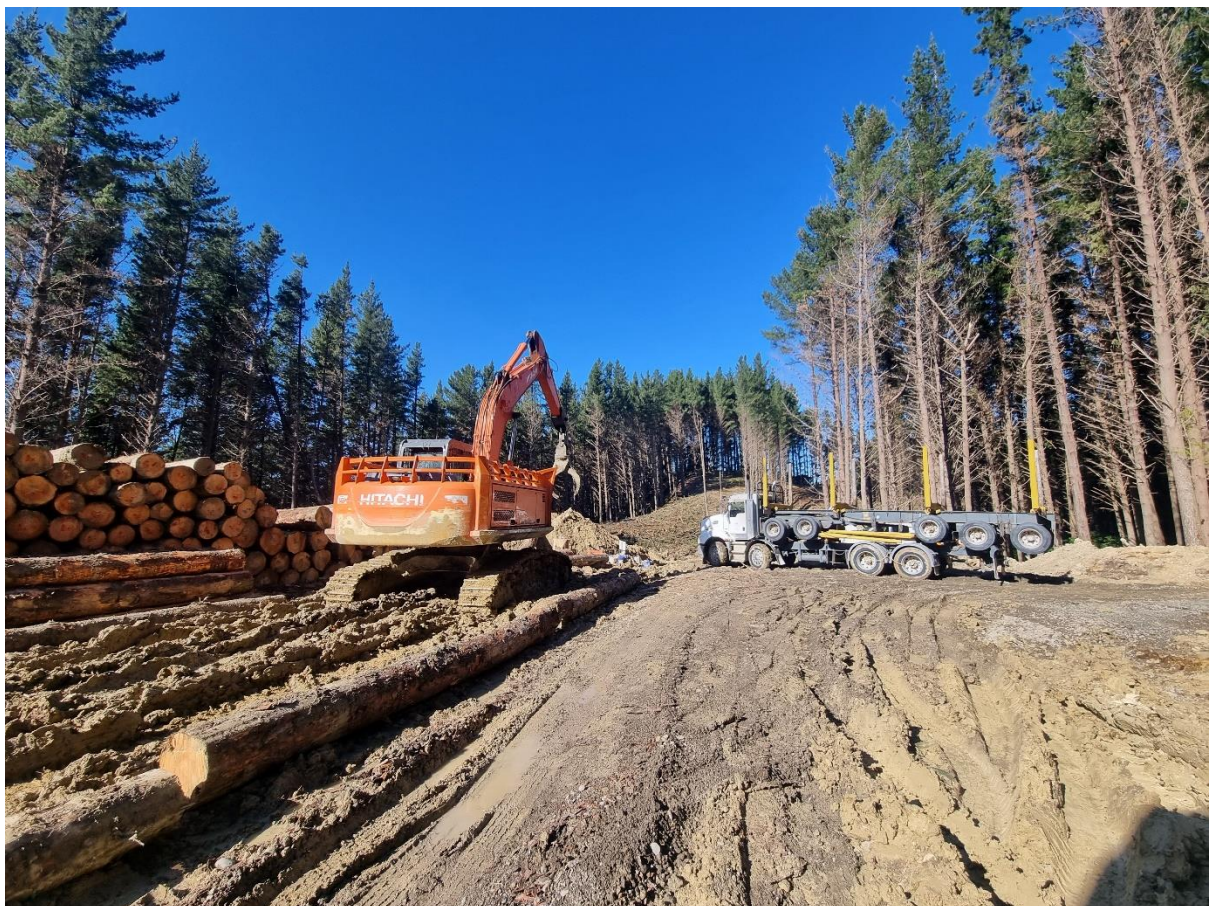
Photo 2: Log truck ready to be loaded up.
