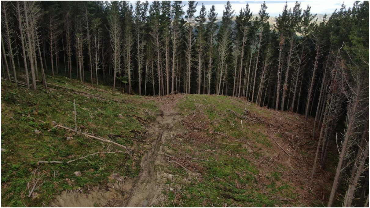
Photo 5: Site for Landing 14 to be constructed on..
