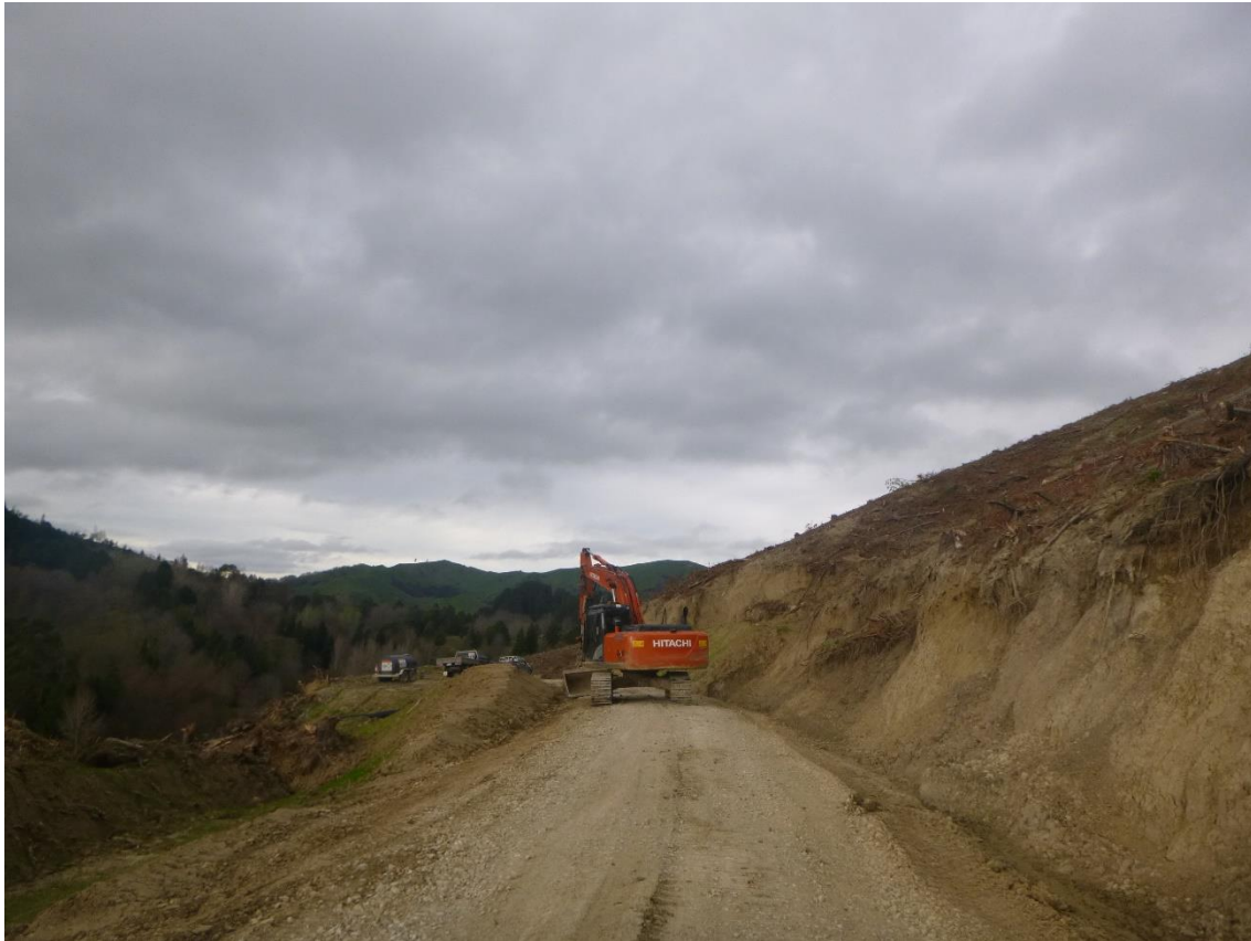
Photo 23: Tahurua Earthmovers conducting maintenance works on Mad Mutt Road between the 0.5 and 1 km markers following heavy rain.
