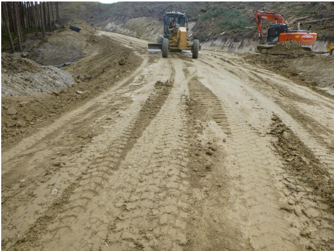
Photo 16: Tahurua Earthmovers forming Mad Mutt Road between the 1.5 and 2 km markers.
