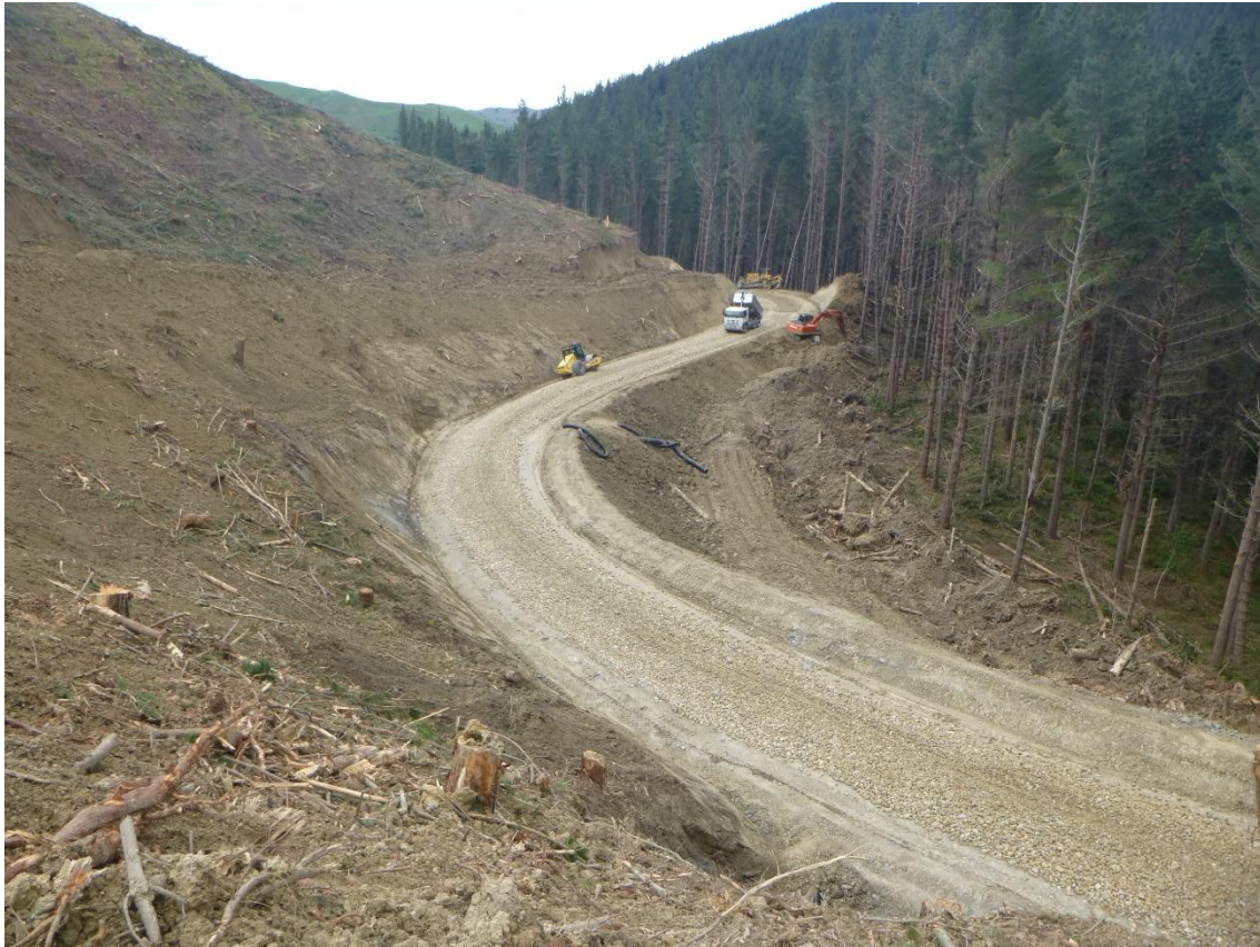
Photo 11: Tahurua Earthmovers formed and now metalling and rolling a section of Mad Mutt Road between the 1 and 1.5 km markers.
