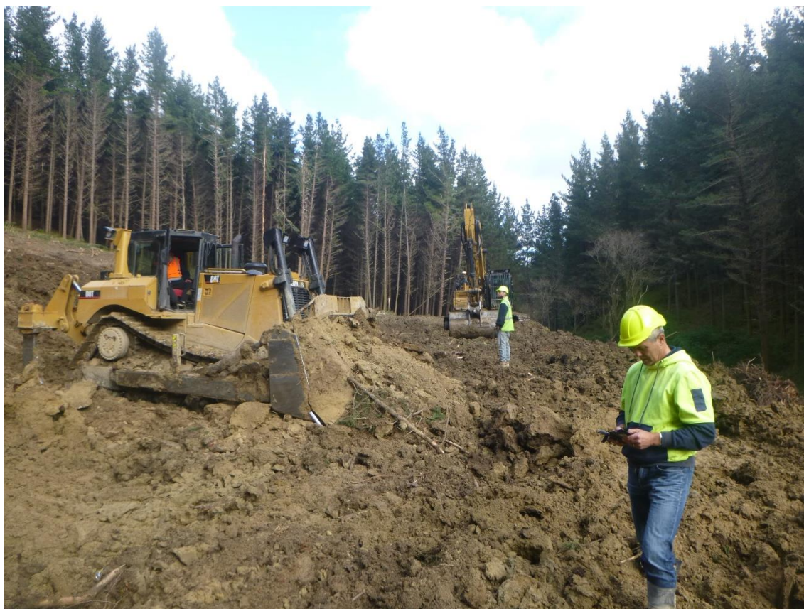
Photo 19: Tahurua Earthmovers constructing Landing 105 on Mad Mutt Road.
