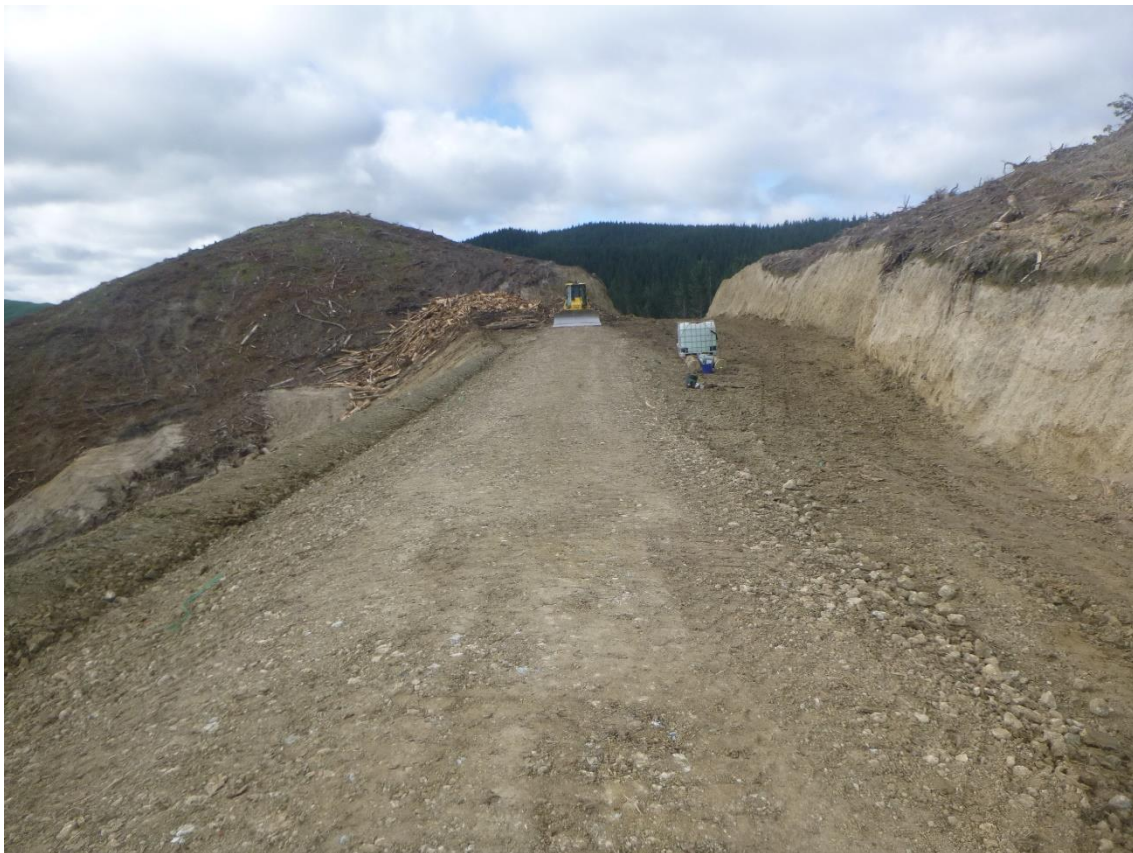
Photo 22: Rehabilitated Landing 2 after being used by A & R Logging in Setting 500.
