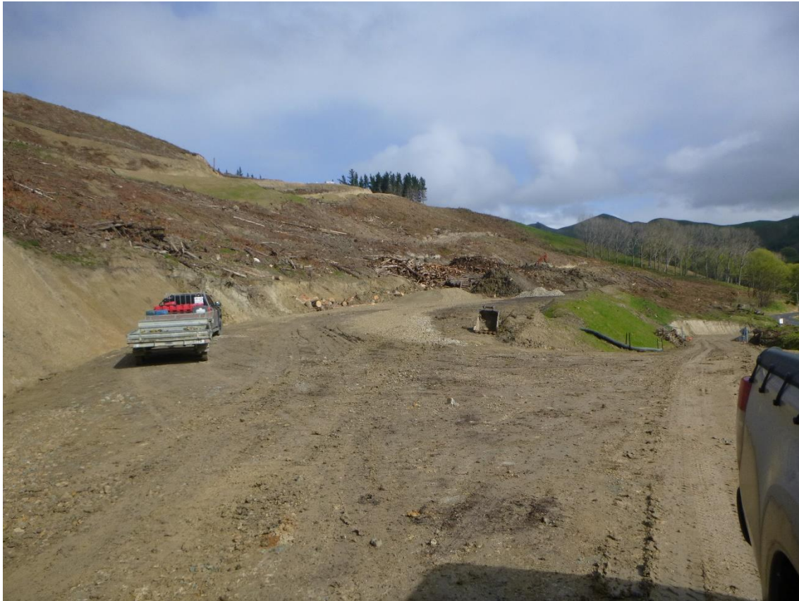
Photo 21: Tahurua Earthmovers rehabilitating Landing 1 which was used by A & R Logging in Setting 500.
