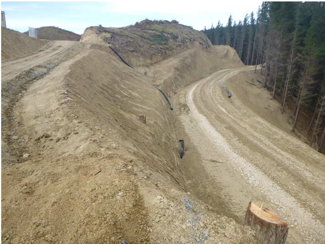
Photo 10: Completed section of Mad Mutt Road between 1 and 1.5 km markers (earthworks in photo 9 above).
