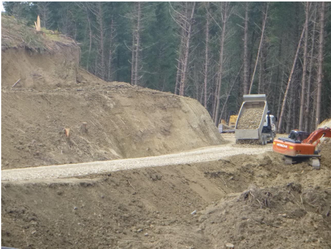
Photo 12: Tahurua Earthmovers metalling a section of Mad Mutt Road between the 1 and 1.5 km markers.
