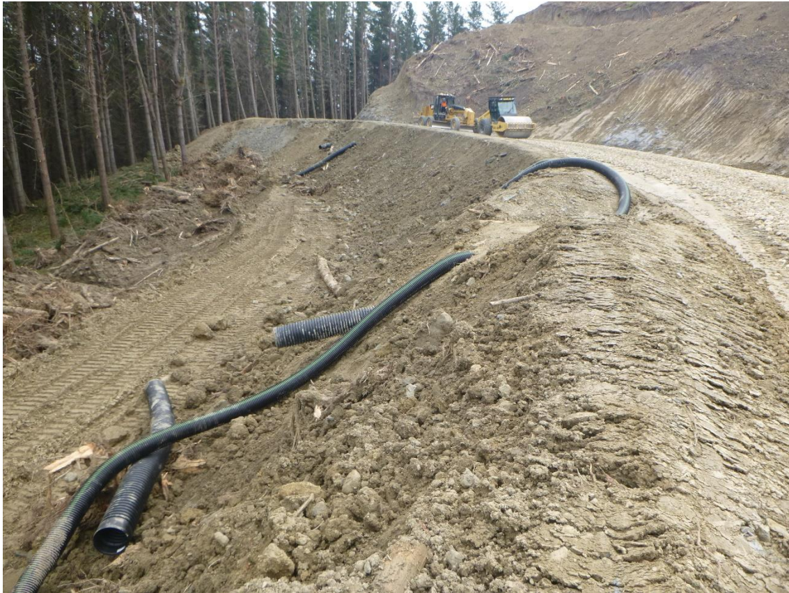
Photo 13: Tahurua Earthmovers grading and rolling Mad Mutt Road between the 1 and 1.5 km markers.
