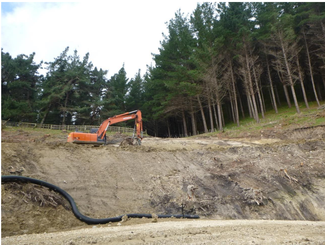
Photo 18: Tahurua Earthmovers forming Wood Road just past the intersection of Mad Mutt Road.
