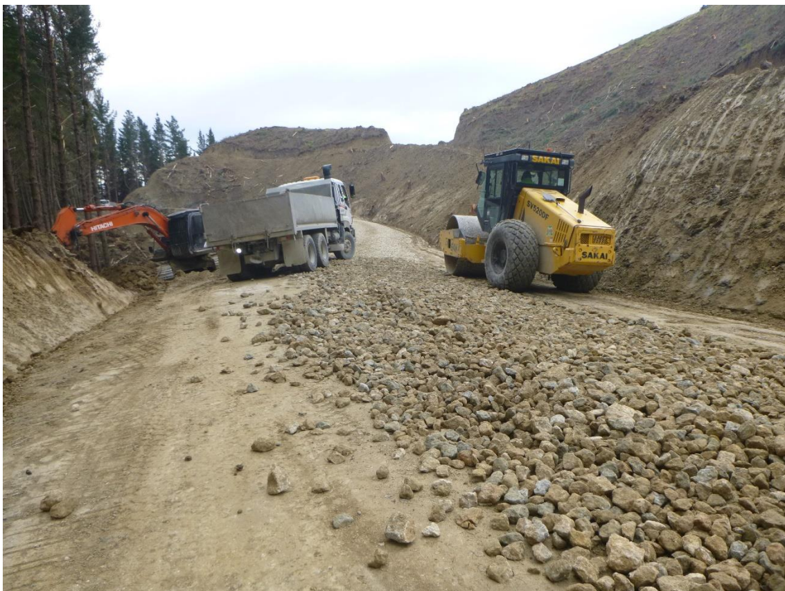
Photo 14: Tahurua Earthmovers metalling and rolling metal on Mad Mutt Road between the 1.5 and 2 km markers.
