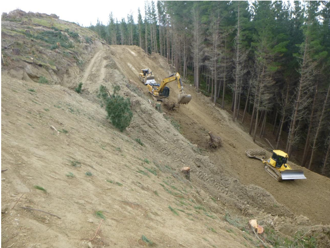
Photo 9: Tahurua Earthmovers constructing Mad Mutt Road between 1 and 1.5 km markers – bringing up large fill bench.
