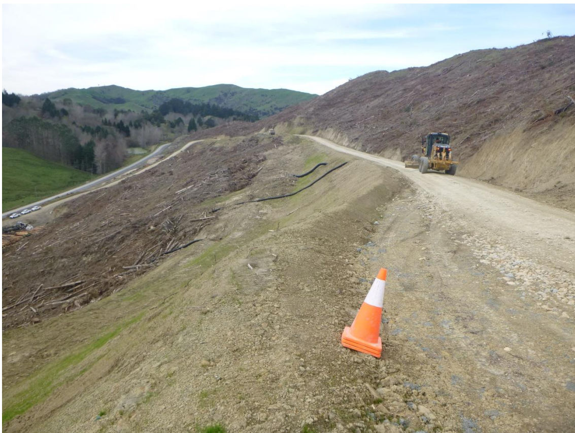
Photo 24: Tahurua Earthmovers conducting maintenance works on Mad Mutt Road between the 0.5 and 1 km markers following heavy rain.
