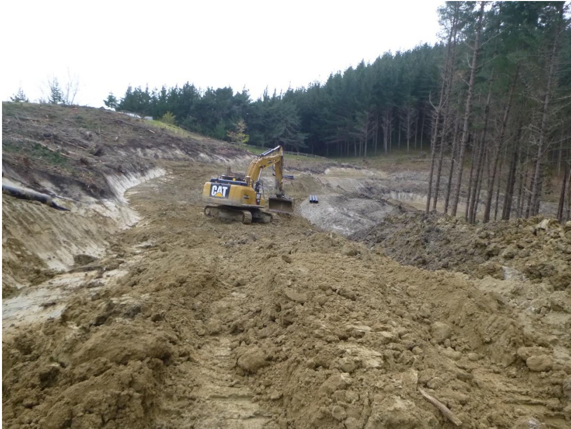
Photo 15: Tahurua Earthmovers forming Mad Mutt Road between the 1.5 and 2 km markers.
