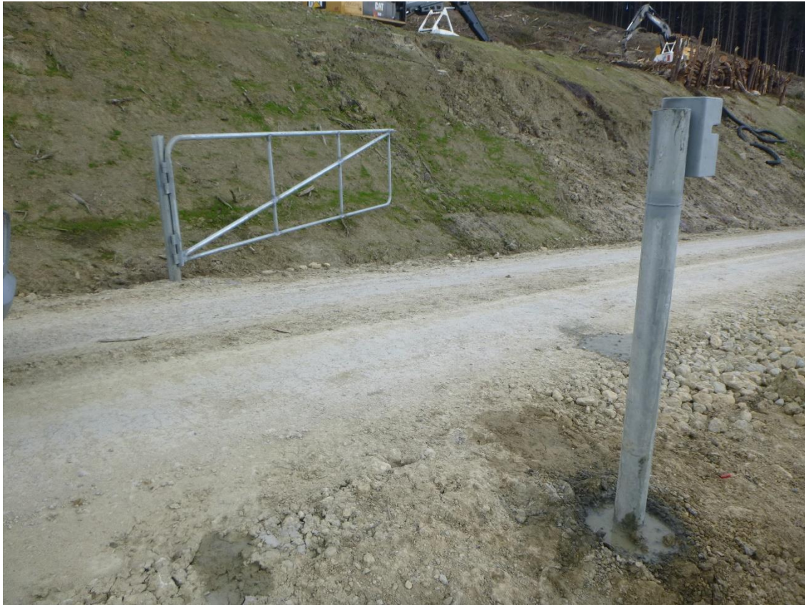
Photo 25: Security gate installed near the start of Mad Mutt Road.
