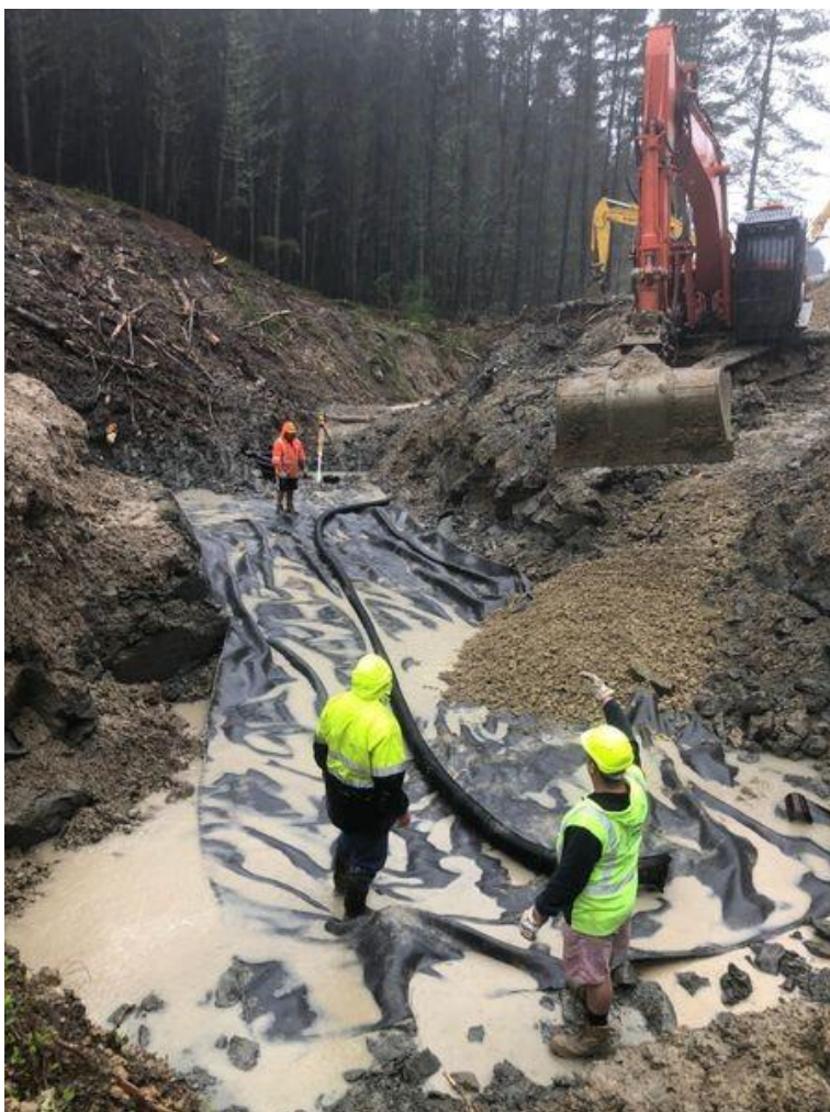
Photo 2: Installation of 2550 mm culvert in Monterey Forest which will be used to cart out logs from Portobello Forest.
