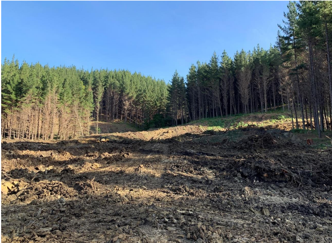
Photo 1: Komatsu D51 stripping ground for roadline in Monterey Forest with Portobello Forest in the background.
