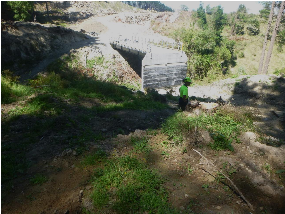
Photo 7: Looking back towards bridge from planned road alignment from northern side of crossing.
