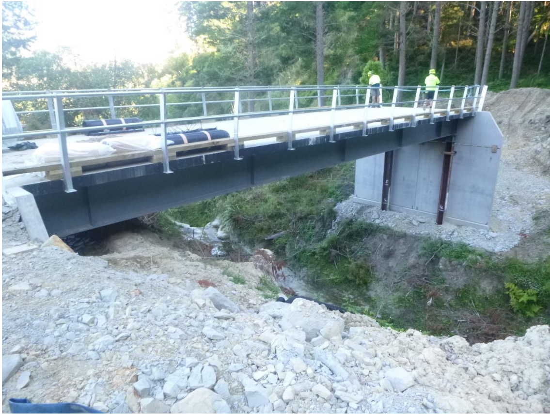
Photo 1: Final touches on bridge installation.
