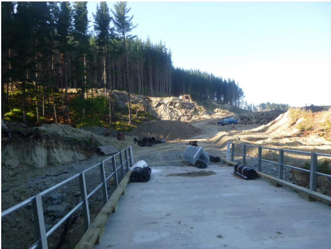
Photo 2: Looking back towards the Smith Road approach from the bridge.
