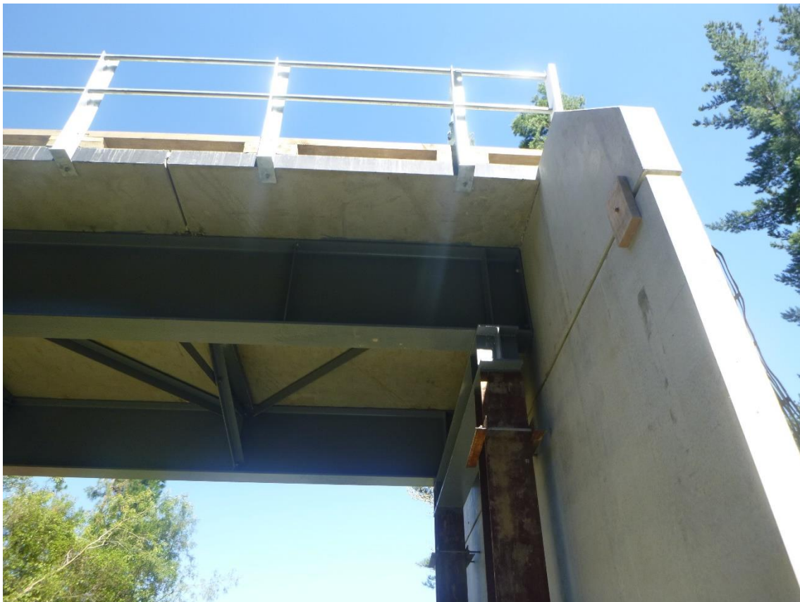
Photo 6: View from underneath the bridge up towards the steel beams.
