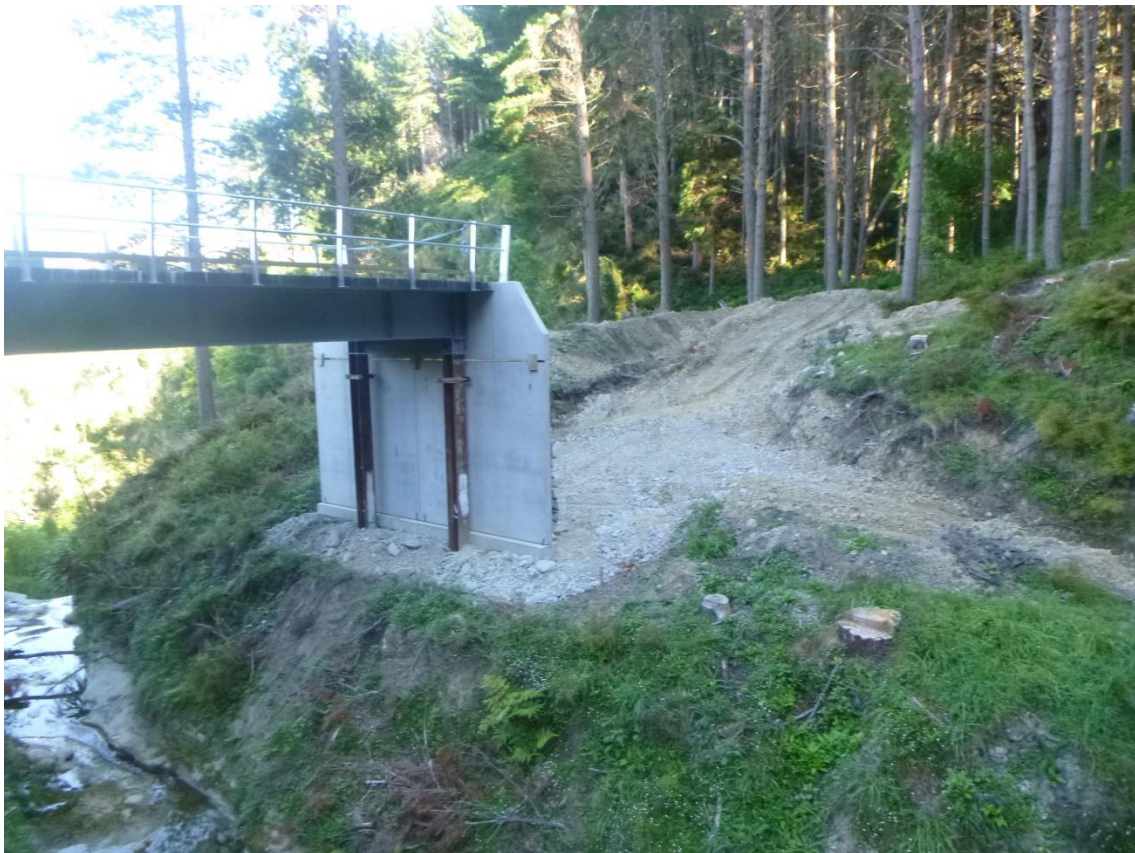
Photo 4: Looking towards the north bank at the completed bridge abutments and where the earth wall construction is to take place.
