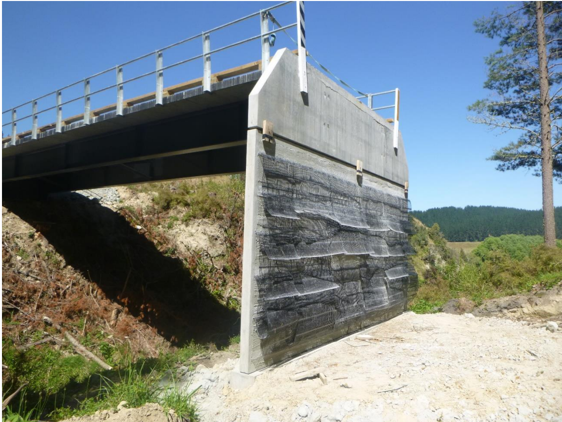
Photo 5: Looking at bridge from northern side of crossing. The sections of black geo-cloth hanging from the precast concrete structure will be tensioned and tied into the earth wall construction.
