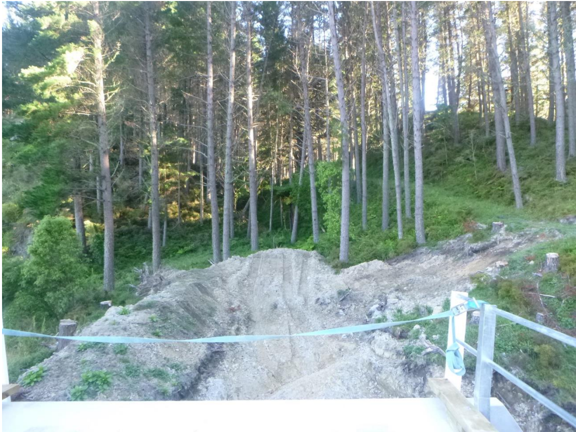
Photo 3: Looking north from bridge towards far side. An earth wall construction is required to complete this approach.
